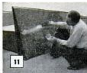
Photos show application of glass fiber and spray painting
