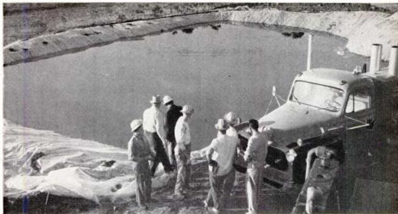
Near Hominy, Okla., this polyethylene-lined storage pit contains 2200 barrels of water for oil-well use
