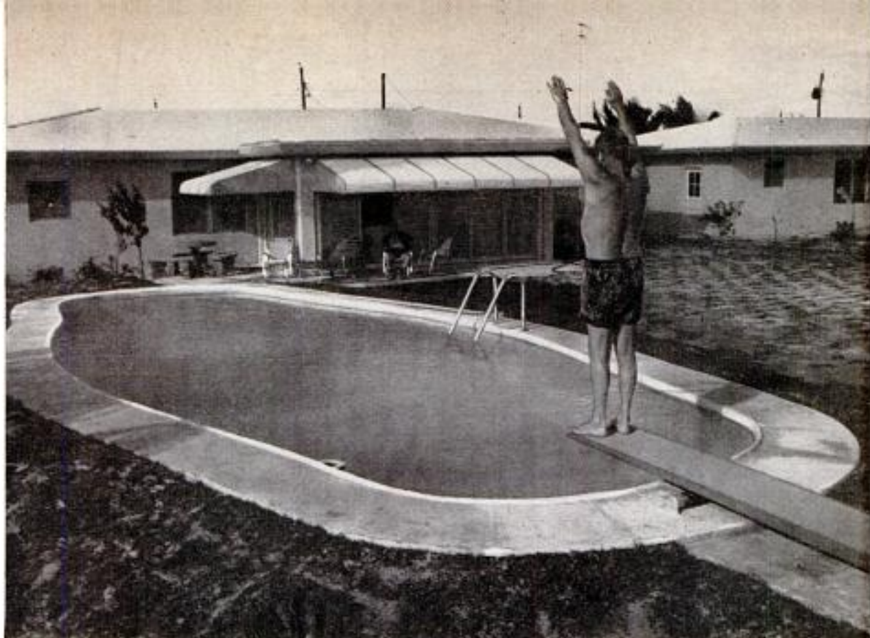
Molded glass-fiber pool arrives on the site in four sections. This is the easiest type of do-it-yourself pool
