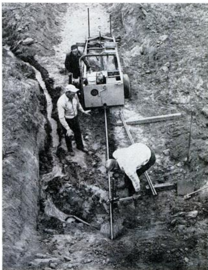
Flow is continuous from hillside wells, which can't be capped because of the high pressure. Below, workmen fasten pipe extension on drill bit
