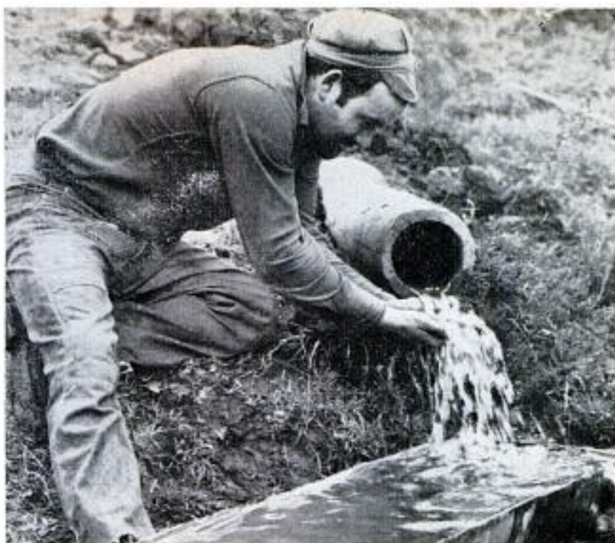
Flow is continuous from hillside wells, which can't be capped because of the high pressure. Below, workmen fasten pipe extension on drill bit
