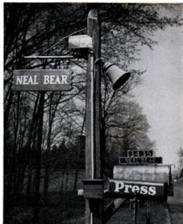
Mailbox-post supports signal lights for school bus as well as floodlight and an intercom unit to house
