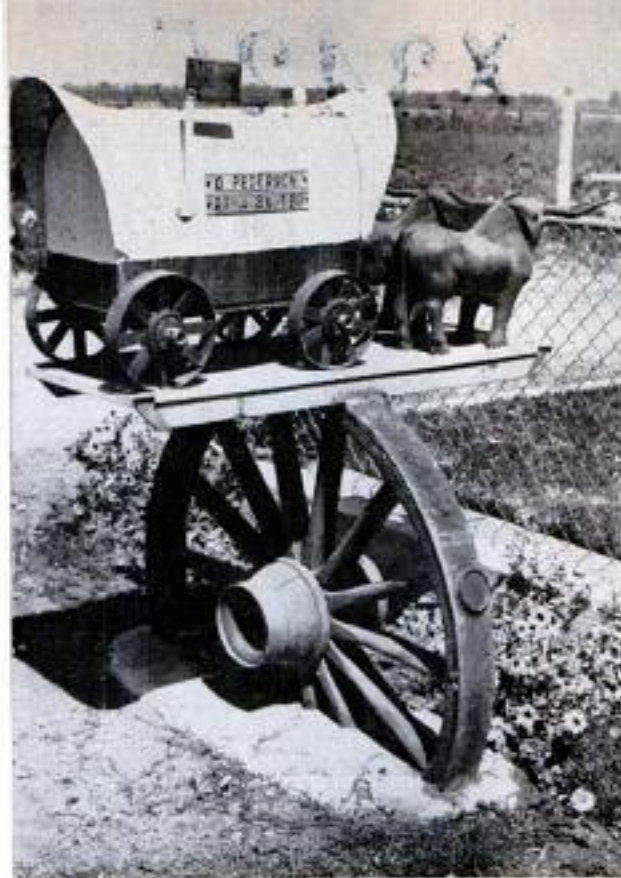
As a sturdy farm-mailbox support, a wagon wheel is hard to beat. Here a most unique box rests on a platform of angle iron which is welded to the steel tire
