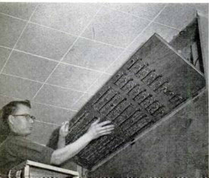
Above, on this birdhouse pole are mounted floodlights and an intercom unit to serve a lawn area. Below, the terminal board can be swung down to provide access to wires behind it for a major circuit change
