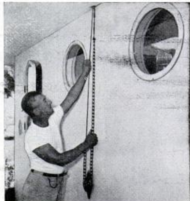
Cable on the rolling roof connects to this chain and leads into the fun room to a ship's wheel
