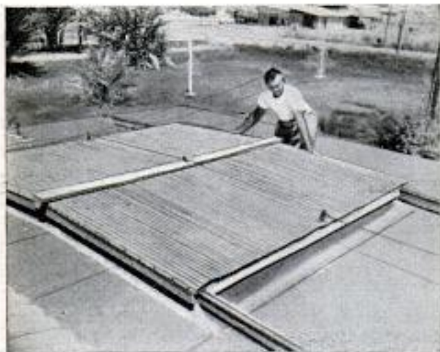
Moving on roller-skate wheels and channel-iron track, this rolling roof is closed from the room below
