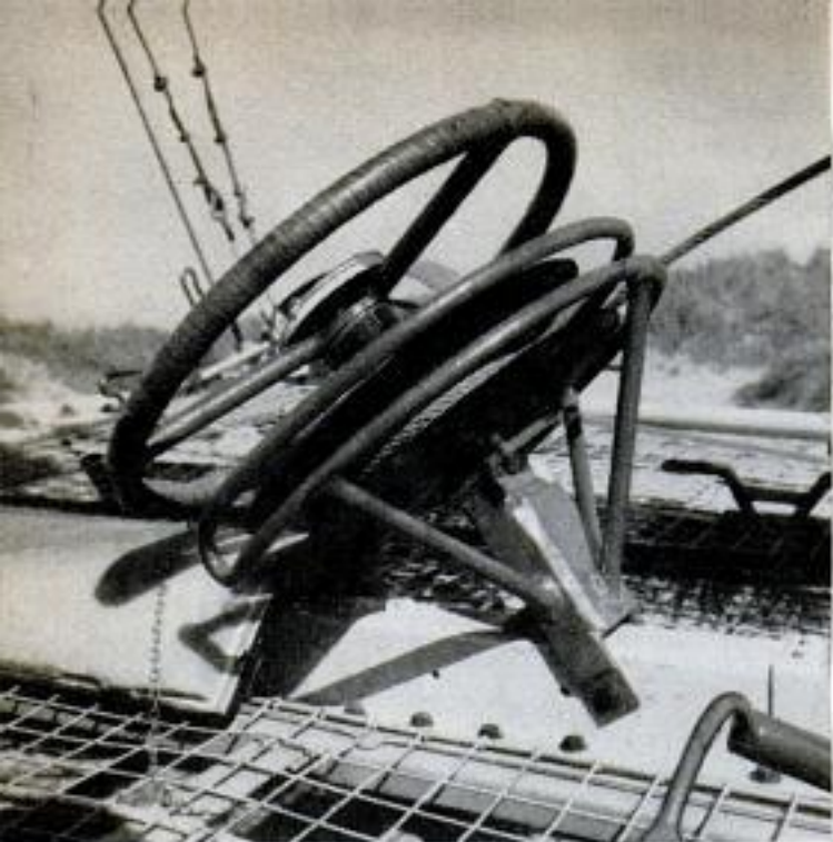
Above, located at the forward end of the yacht, this winch wheel and cable keep the mainsail taut
