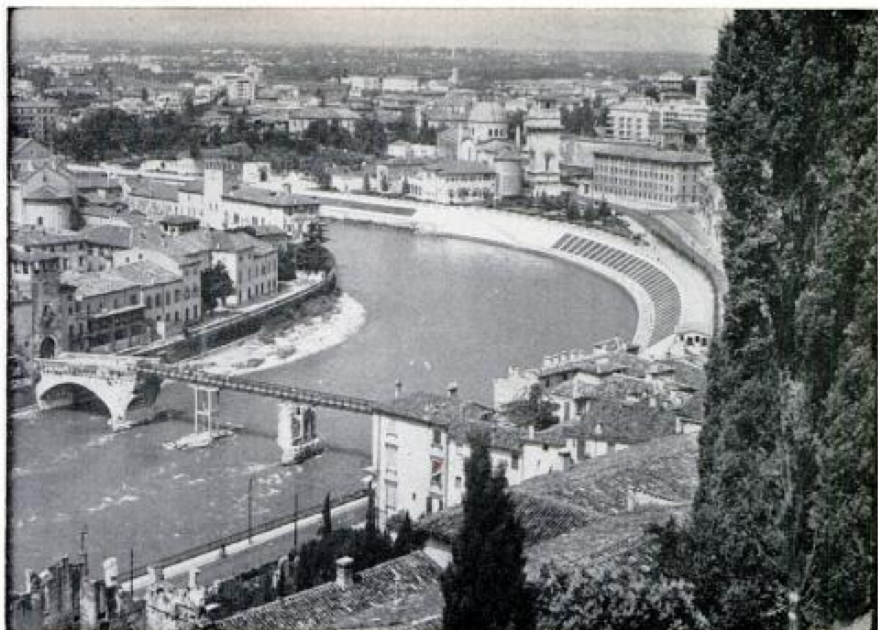
Aerial view of the blasted Ponte Della Pietra, showing temporary steel bridge for use during restoration
