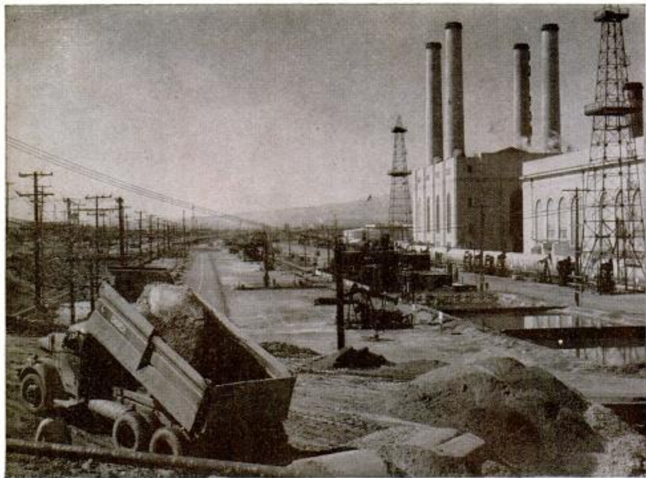
Dirt road at left is raised above high-tide mark. The steam electrical generating plant has sunk 22 feet
