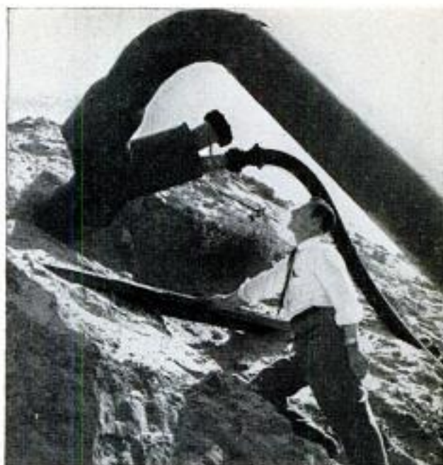
Discharge tube, pumped to keep rain and floodwaters from area, runs through one of the protecting dikes
