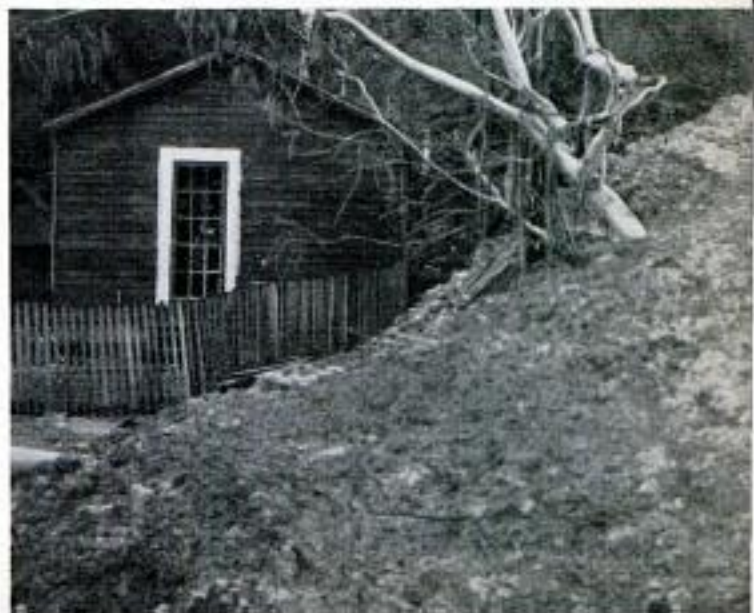
Heavy rains and melting snow caused the hillside to slide down and almost engulf poorly located cabin
