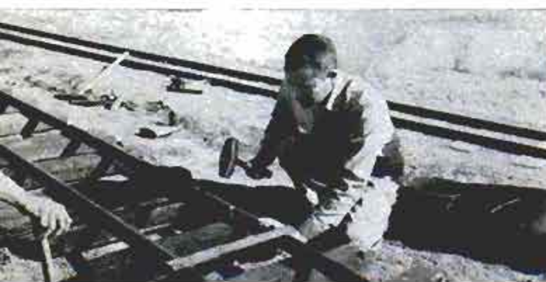
Below, Guy Stillman, owner of the Paradise and Pacific Railroad, applies muscle to spikes on the line
