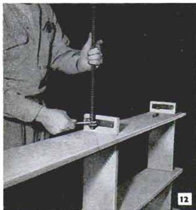
After assembling hangers as below, draw all fasteners tight. Make sure all threaded rods are vertical
