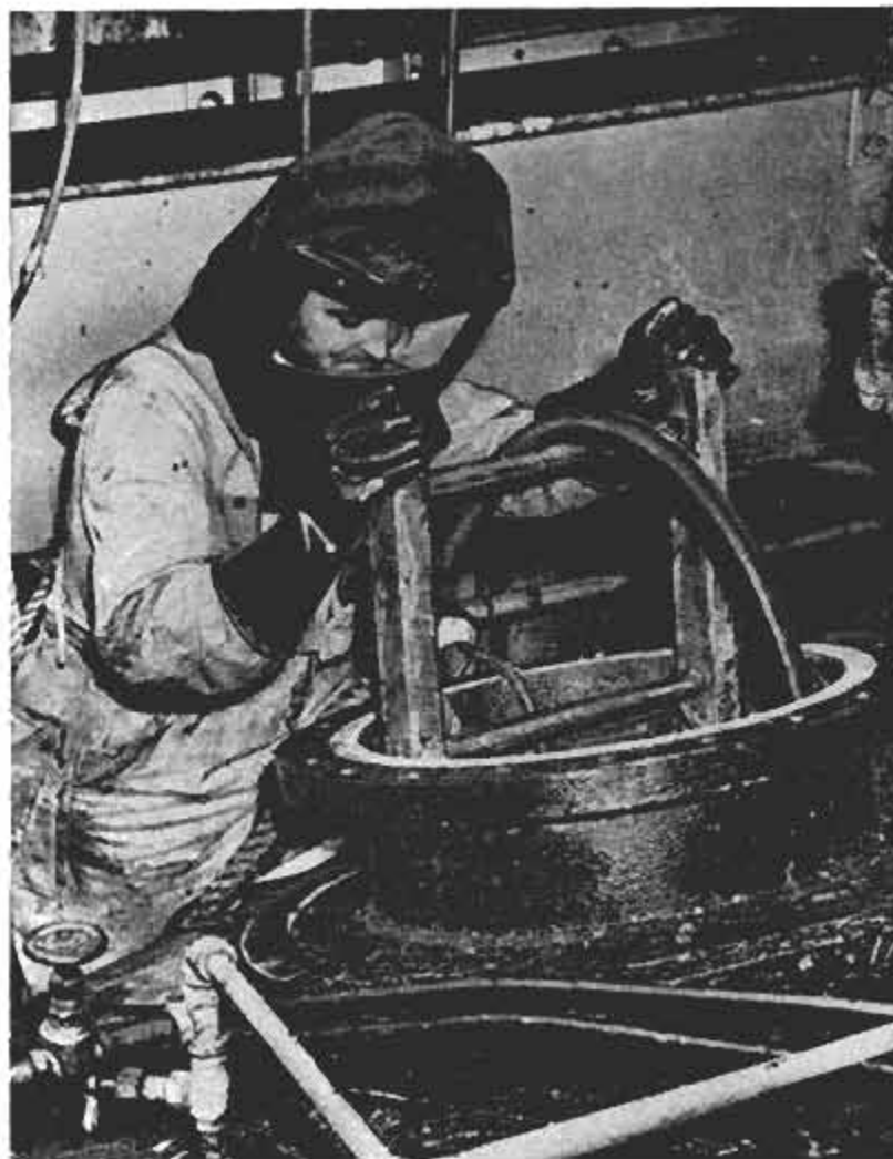
Woman operator of sand slinger wears a protective dustproof nose guard and goggles. Below, workman in rubber tank breathes fresh air piped to helmet
