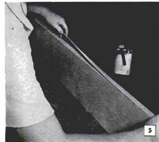
When necessary to leave plywood edge exposed, cover grain ends with Woodtape applied with special solvent
