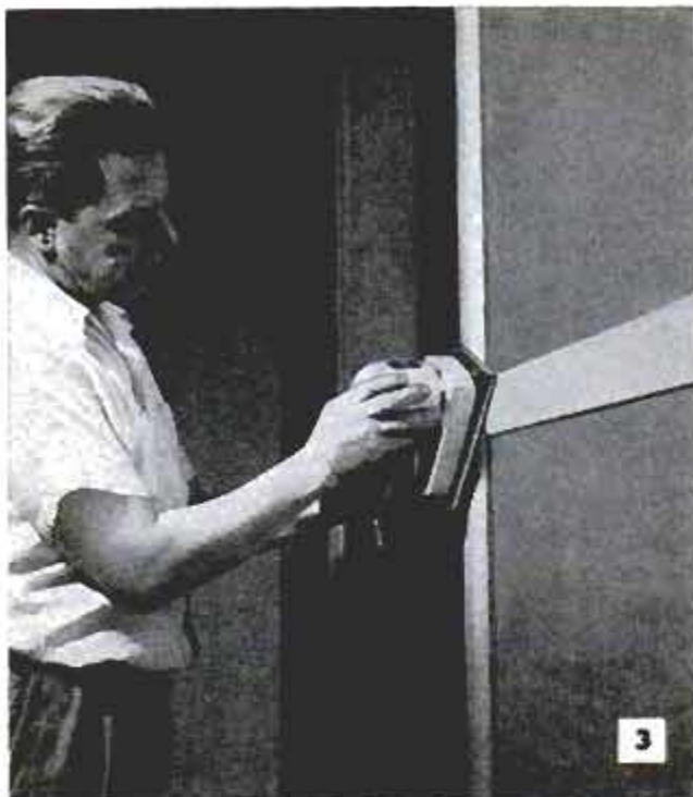
Although hardwood plywood has smooth surface, sand lightly before finishing. Sand the millwork, also
