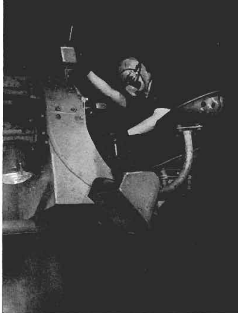
Woman operator of sand slinger wears a protective dustproof nose guard and goggles. Below, workman in rubber tank breathes fresh air piped to helmet
