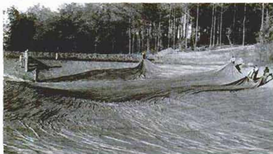
Waterproof plastic tarpaulin, above, is used to cover nearly half an acre of the dry bed of a manmade pond. Below, pond no longer seeps away
