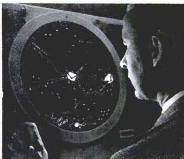
Below, electronically generated map of the control area is projected on AASR screen at flip of switch
