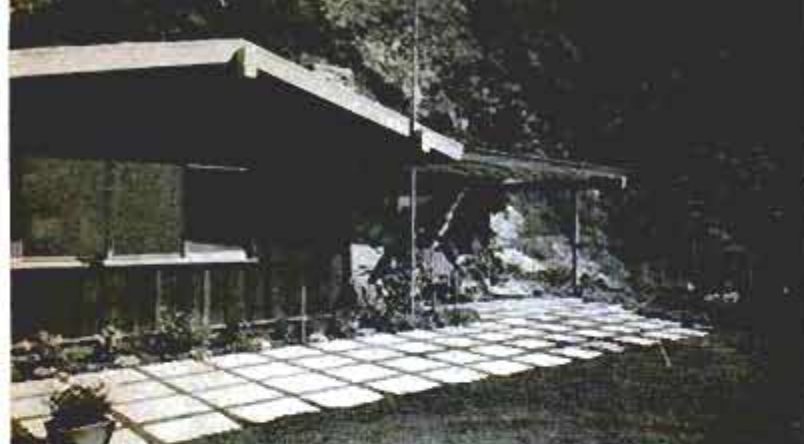
7. Above, precast-concrete squares laid on soil, spaced 1½ in. apart with dichondra planted between
