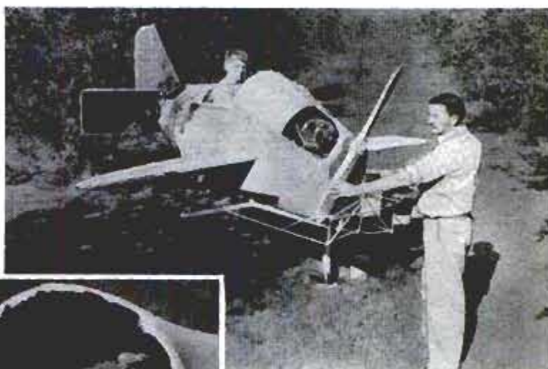
Child's plane is mounted on universal joint that is bedded in concrete
