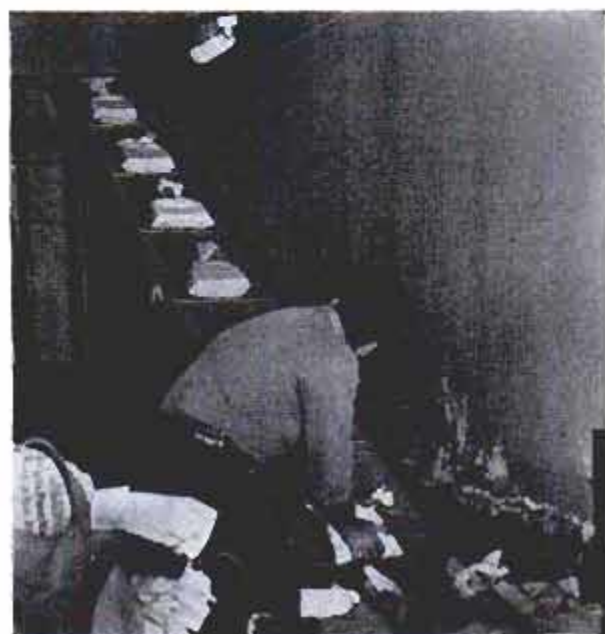
High-speed sorter separates and counts coins from pennies to half dollars, rejects slugs and foreign coins Semiautomatic machine wraps and counts rolls. Armed guard places bags on conveyor for delivery to surface
