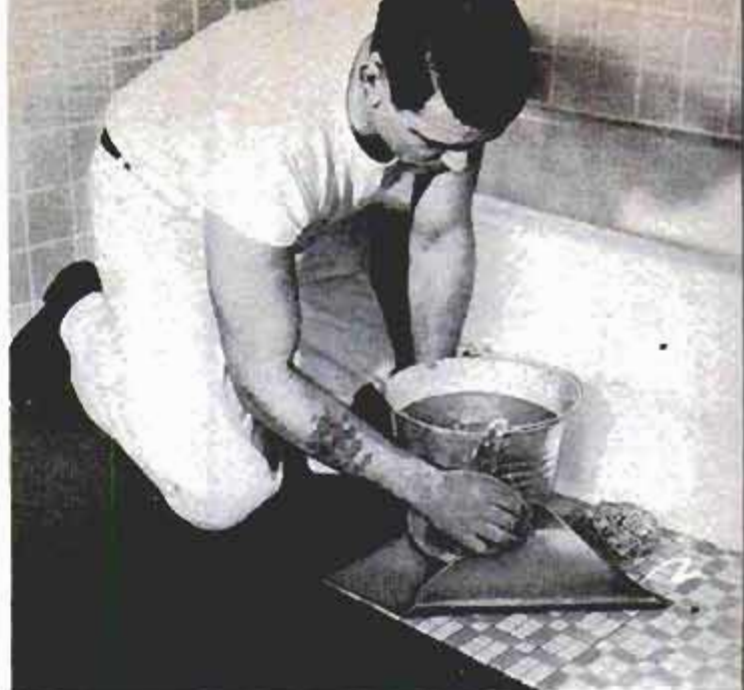
Minimum amount of water is used on paper, since moisture on adhesive greatly increases setting time
