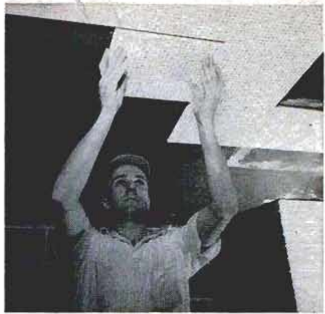
Acoustical tile on ceiling only often is sufficient to reduce noise levels to an acceptable minimum
