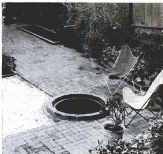
10. Above, brick laid in basket-weave pattern without use of mortar makes interesting walk around patio
