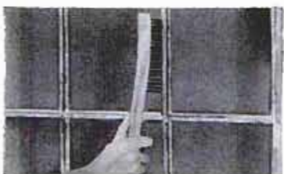
Clean metal surfaces with wire brush. Spot-prime bare spots on old metal.
