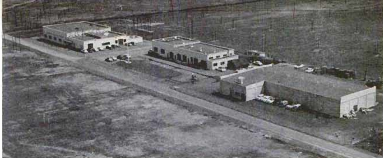
Above, Davis Communications Center from the air. Below, array of automatic teletypewriters at the center
