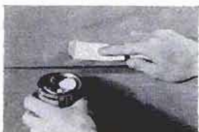
Caulk all joints next to windows, etc. Putty all nail heads.
