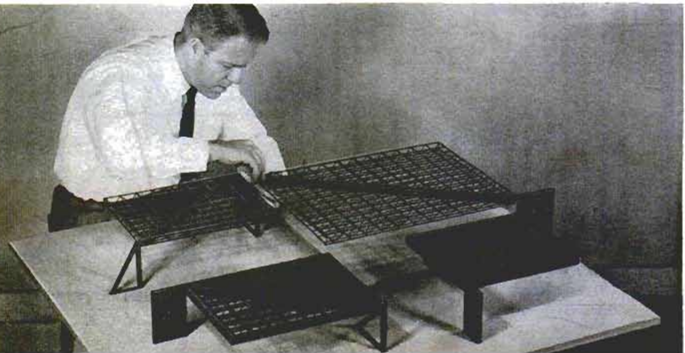
Close-up of structural section shows double steel beam and steel triangles which carry roof weight
