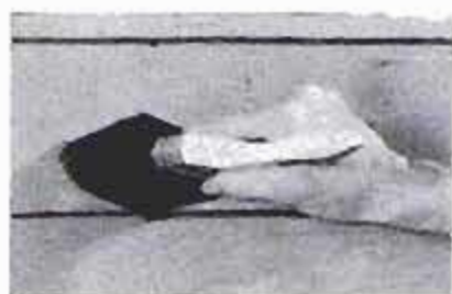
Surface must be clean, smooth and dry. Sand rough spots, dust clean.
