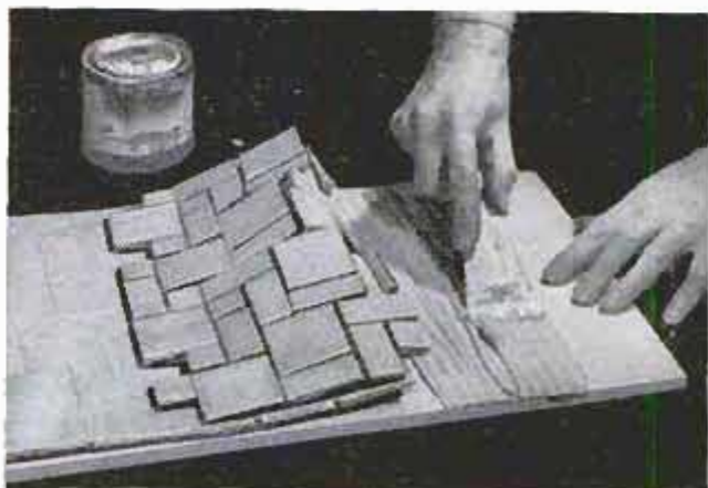
Below, after adhesive has dried for 12 hours, grout is wiped into joints and between tiles and angles
