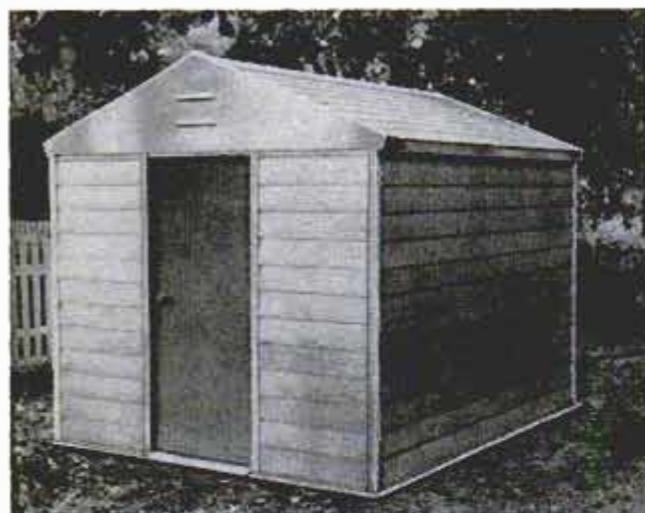
Parts of storage room are cut, shaped and drilled, all ready for assembly with pliers and screwdriver
