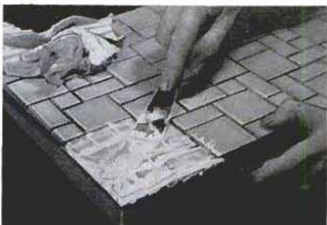
Below, after adhesive has dried for 12 hours, grout is wiped into joints and between tiles and angles
