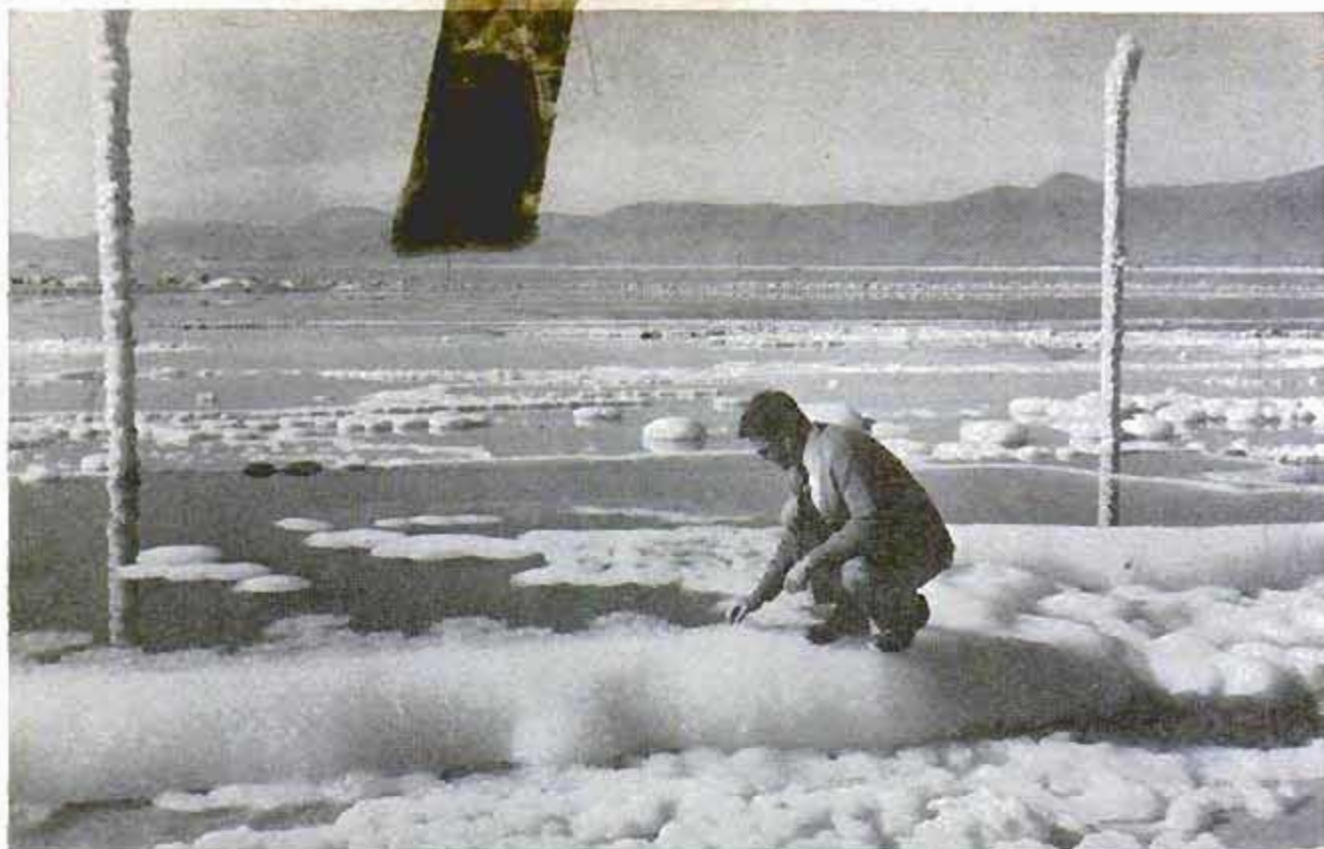
Glauber salt is precipitated out of brine by a spraying process at Searles Dry Lake, Calif. Methods similar to this may eventually be used to extract many products from ordinary igneous rocks such as granite
