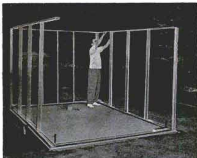
Parts of storage room are cut, shaped and drilled, all ready for assembly with pliers and screwdriver
