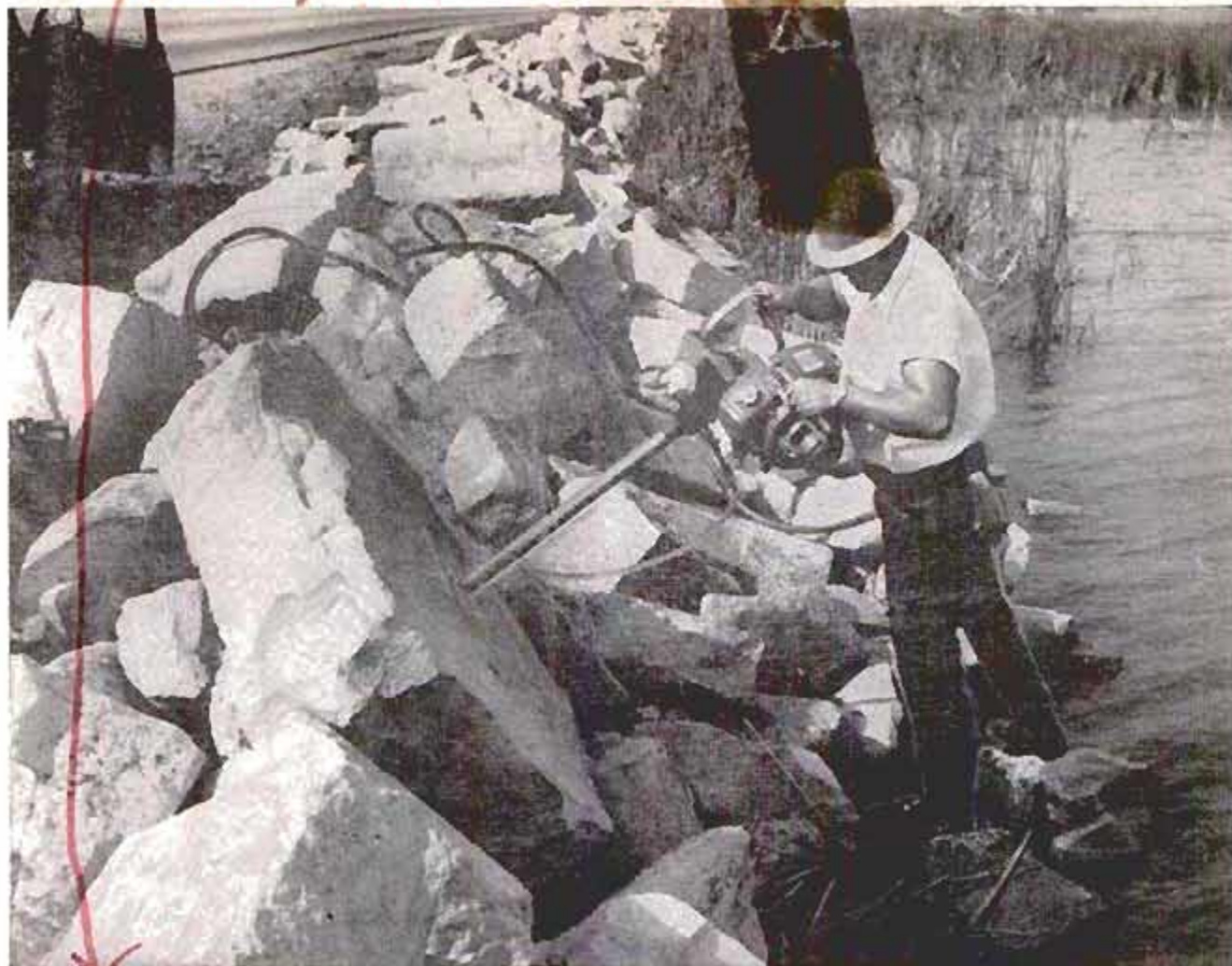
New portable coring tool replaces heavier, more expensive equipment, samples rock to depth of 50 feet
