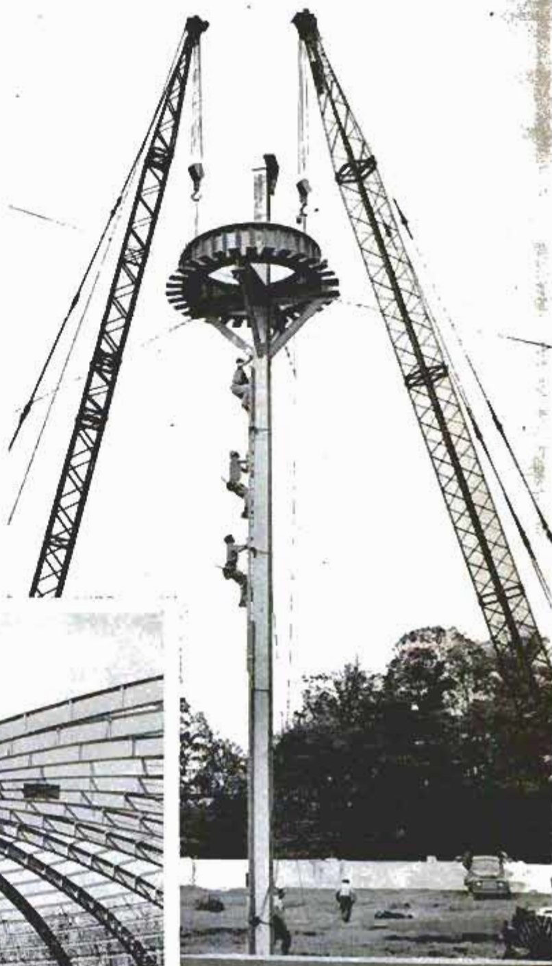
Completed framework of Alexander Memorial Center, in Atlanta, Ga., required 615 tons of structural steel
