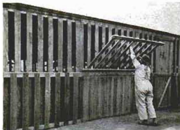
Panels in upper wall of Leo Zumwalt house open to any angle. Below, Elmer Moreland drops slatted panels. At right, Max Glick house has adjustable louvers
