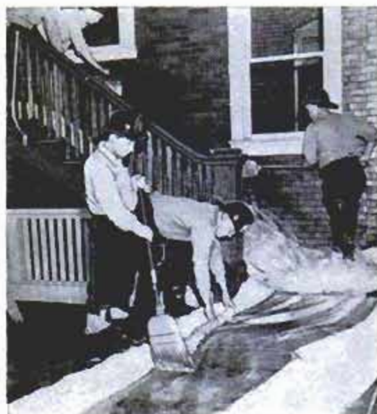
Rolled-up cloth serves as dam to keep water pouring down the staircase from spreading
