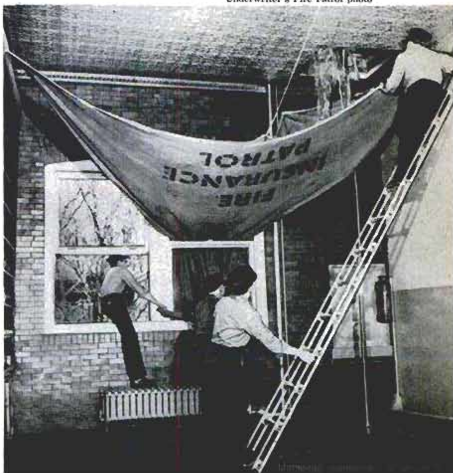
Ballooned cover is hung from ceiling where opening has been made to let the water flow down and be chuted out window Underwriter's Fire Patrol photo
