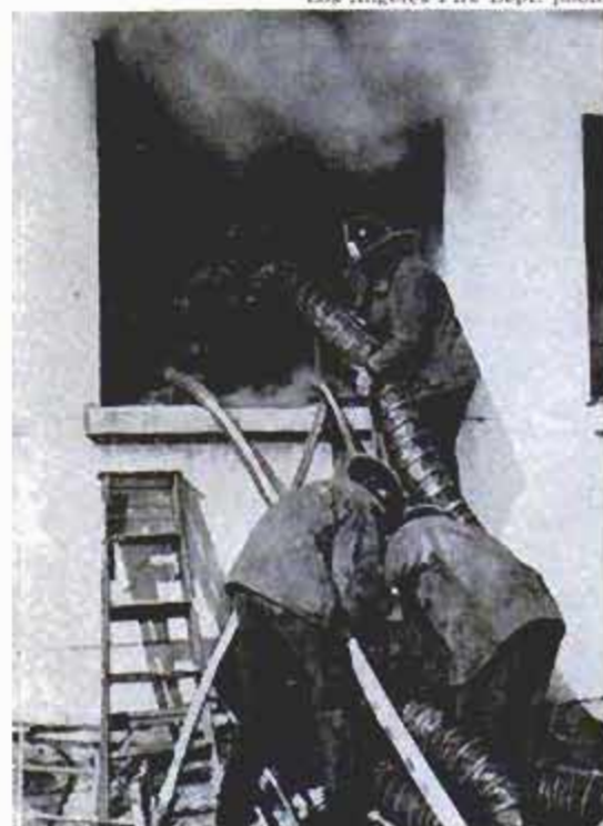
Flexible smoke-ejector tube is poked into basement to rid it of noxious fumes and gases
