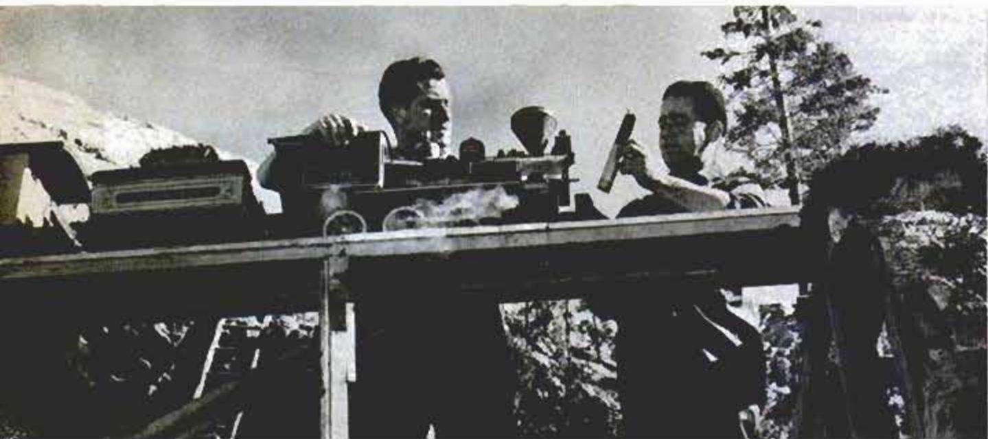
Special-effects men install a cartridge in locomotive which will provide realistic smoke during the filming
