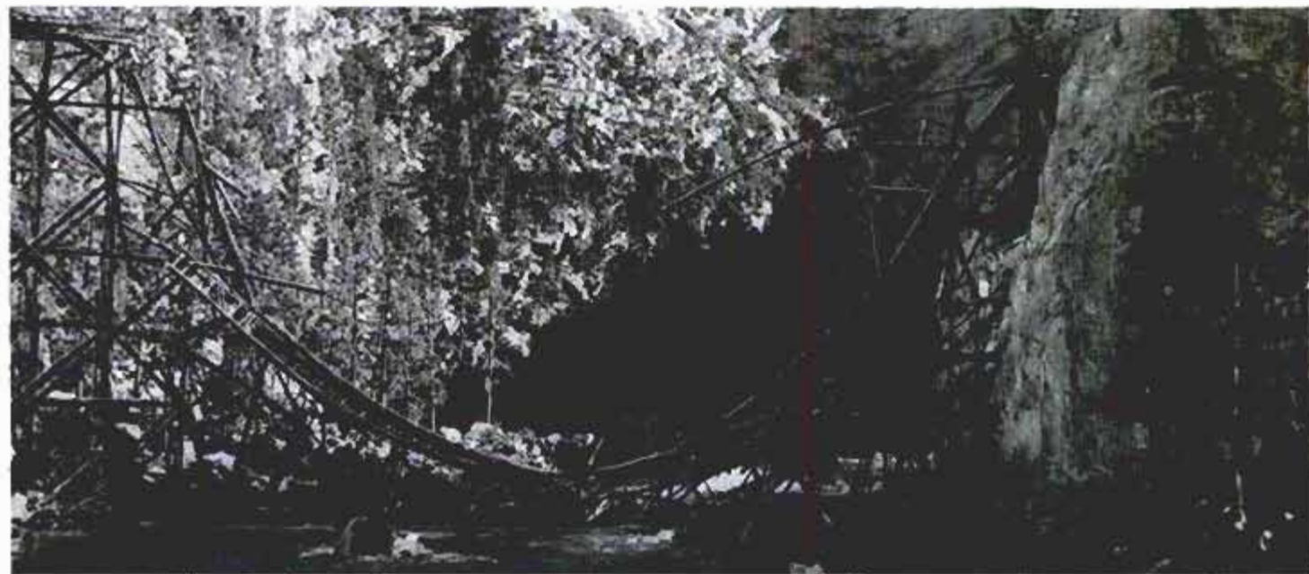
Cables are fastened to pipe hidden beneath the water. As the pipe turns, the timbers begin to break one at a time to bring down trestle just as the train thunders over the rails above
