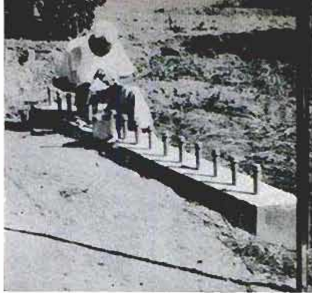
These are the exposed ends of plastic pipe Caryl is testing underground. Once a month he uncaps pipe ends and inspects them for water leakage, as shown
