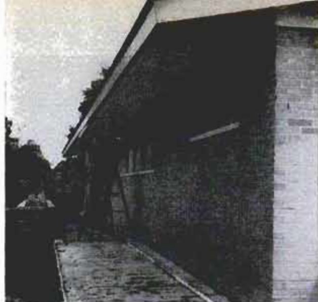
Air forced into attic by exhaust fan is discharged through vents cut in underside of roof overhang
