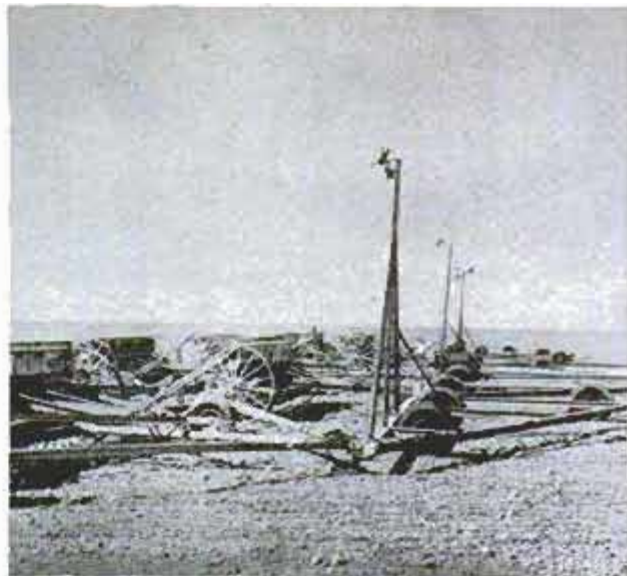
Intricate hitch, supported by 23 wheels, is made of steel beams and pipe. Floodlights permit night work
