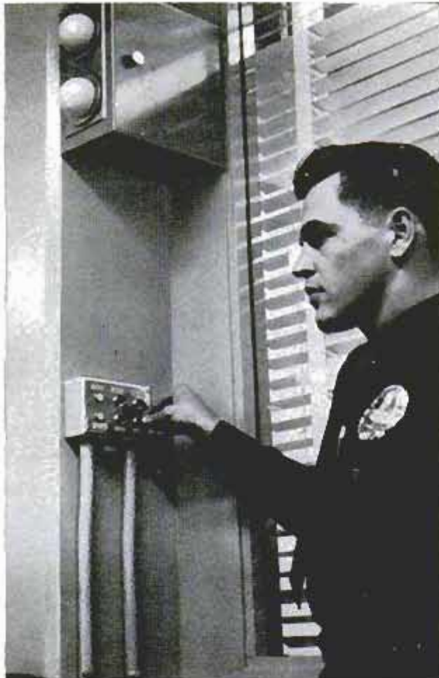
Doors throughout building are push-button operated and only two men have keys, which are seldom used
