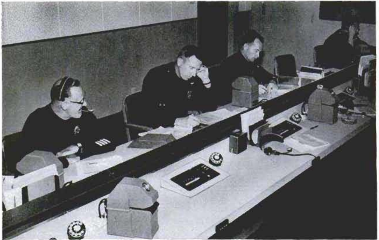
Complaint board is entirely automatic. Incoming calls are sent electronically to an open position. If all positions are busy, a call bank stores them until one is open, then releases them in the proper sequence
