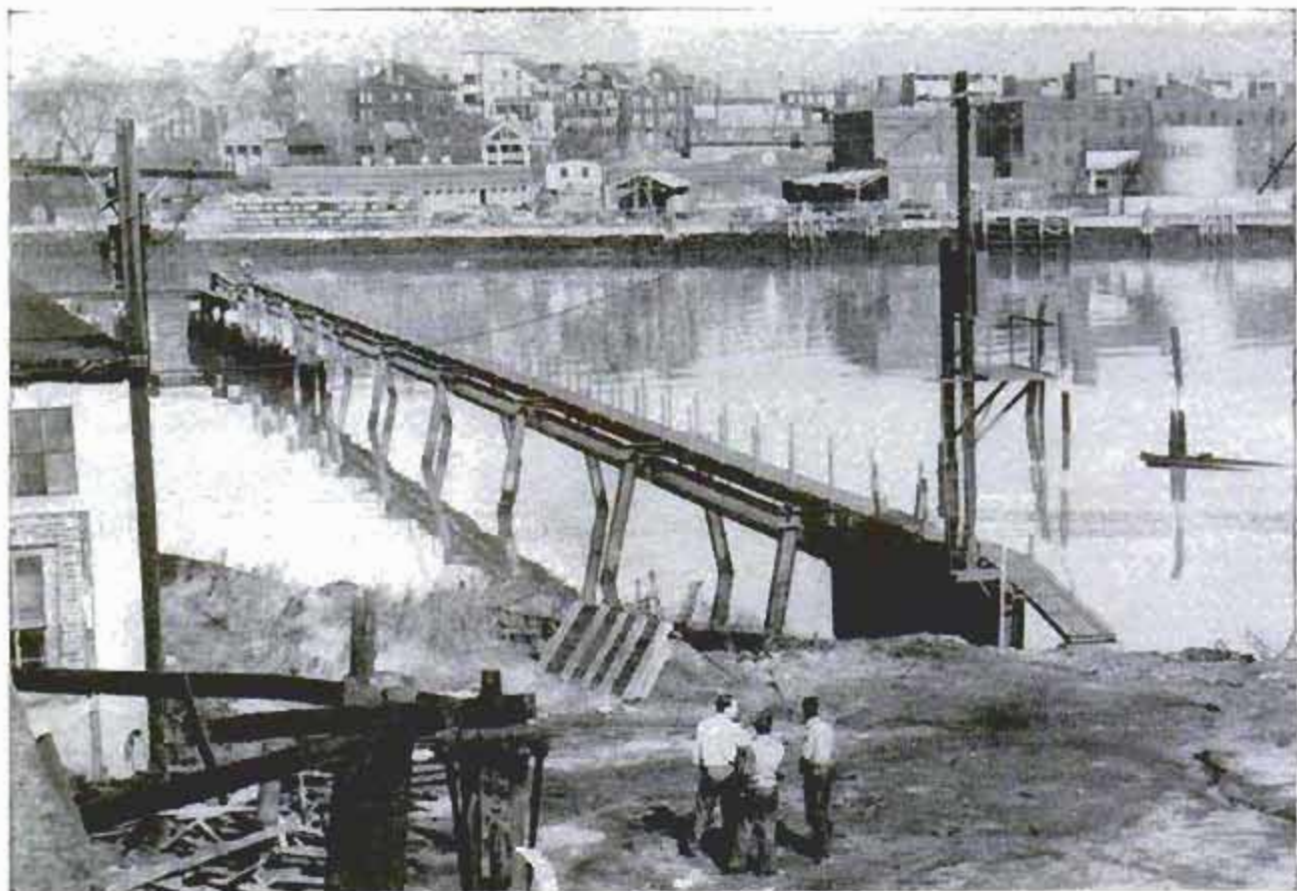
Platform on pole at shore end of floating fire barrier is control station for operating 400-foot booms
