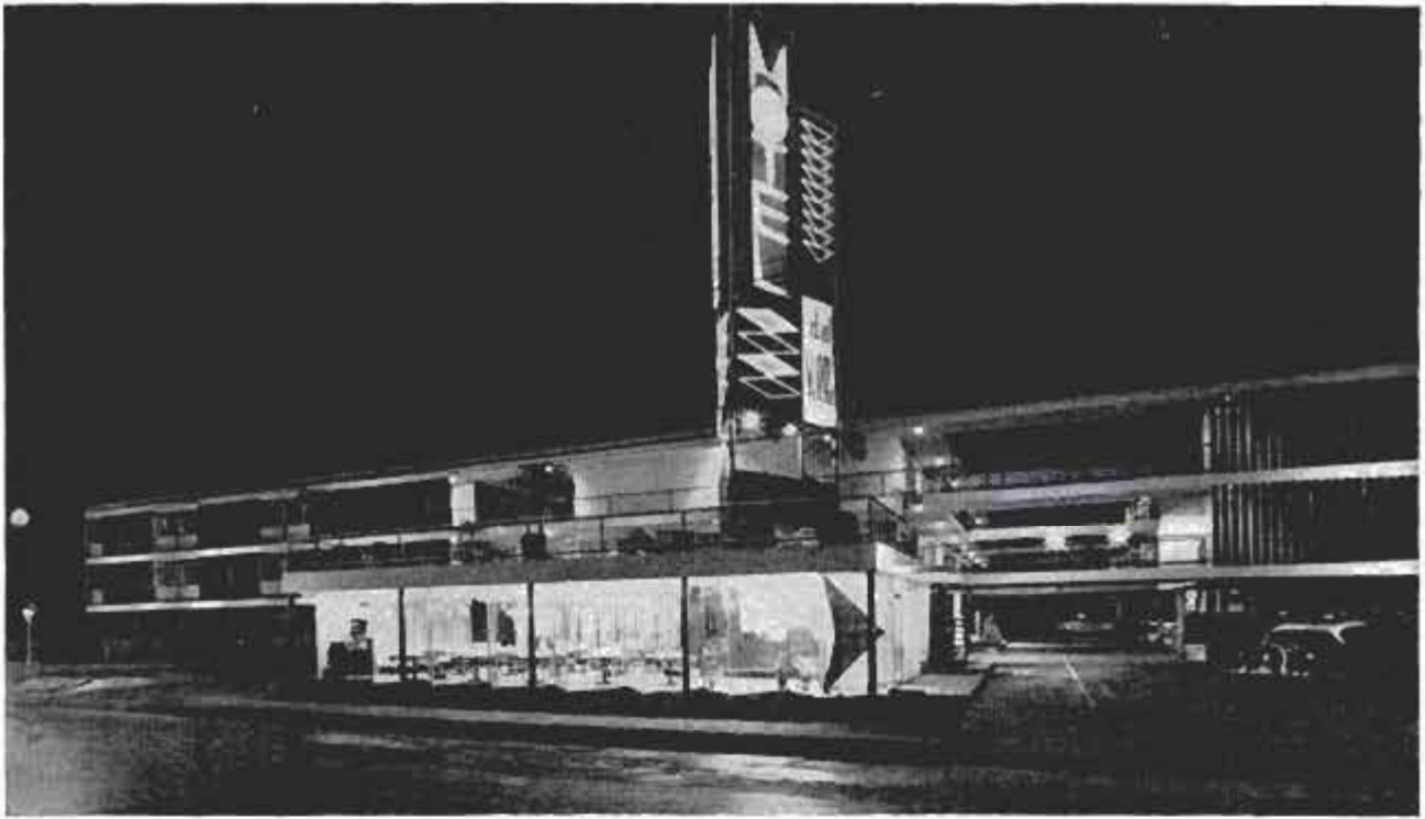
Sixty-foot pylon advertising motel in New Orleans is hollow, contains air conditioner for dining room
