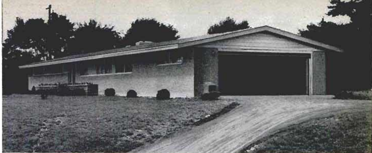
Common attic shared by house and attached garage, as in house pictured above, presents an ideal situation for locating attic exhaust fan in ceiling of garage, where it is isolated from the main living area
