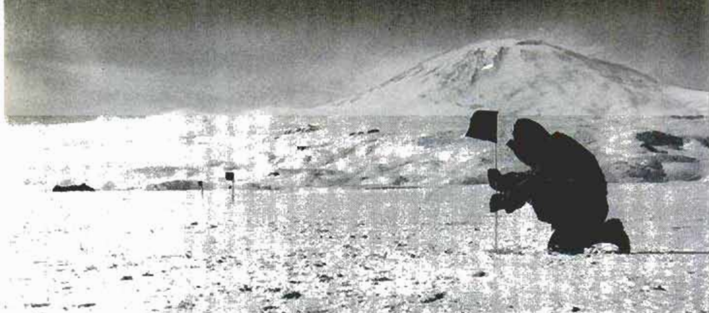
Scarlet trail flags were planted in holes in the ice and frozen in place to outline the runway boundaries
