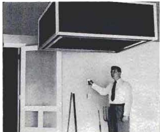
Lower left, finished installation of fan presents neat appearance and provides ample headroom. Timer and control switch are located on wall. Lower right, canvas strips fitted between wooden framework and fan frame prevent recirculation of exhausted air
