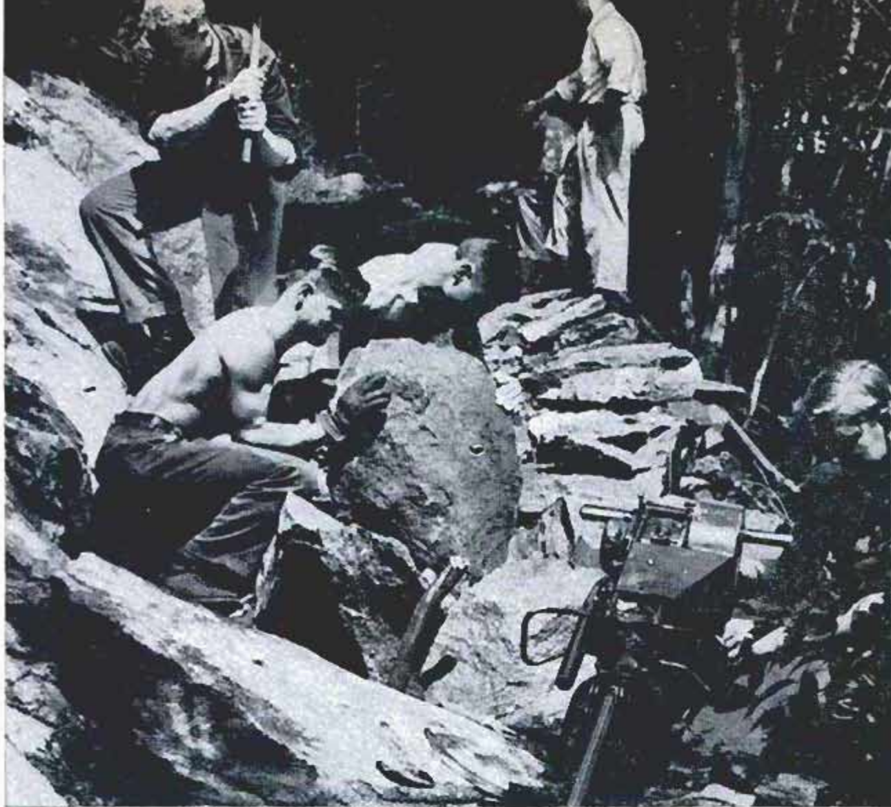
After rocks have been broken up, some are rolled out of the way and others are saved for building trail
