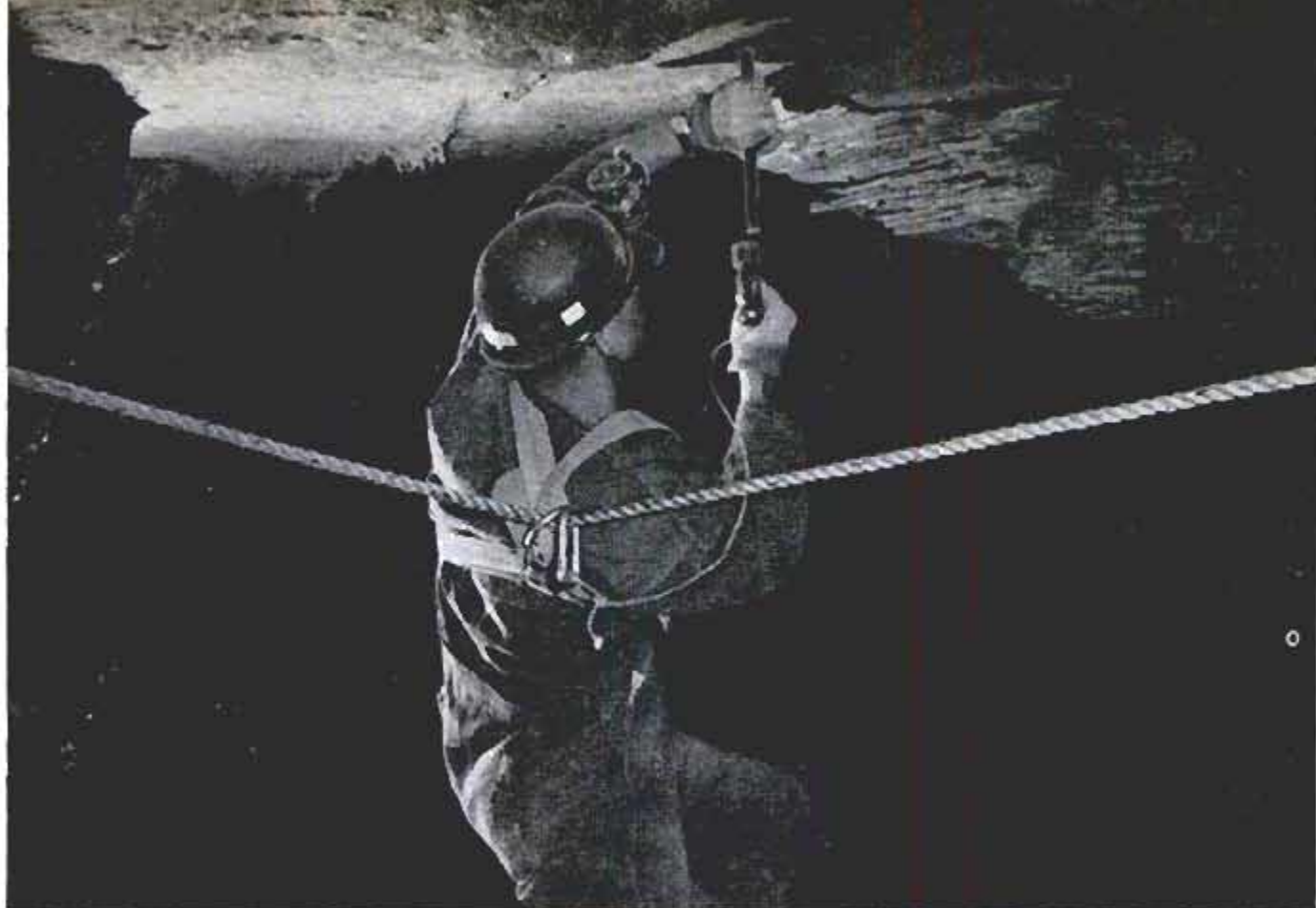
Working on a tilting slope at brink of pit, one of the men drills hole into ceiling for block and tackle
