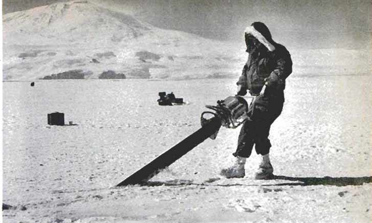
Ice for the runway at McMurdo Sound was tested for thickness with a seven-foot motorized chain saw
