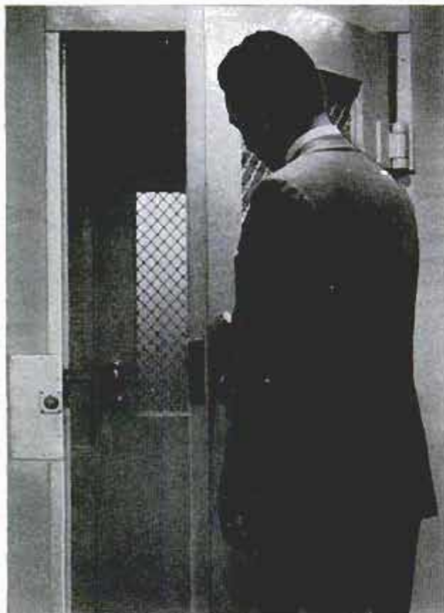
All exits to central jail have double doors. The second cannot be opened until the first has been closed
