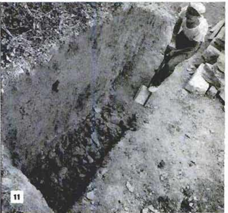
First step usually is to square earth shoulder against which wall is laid. Next is to excavate for stone or concrete footings
