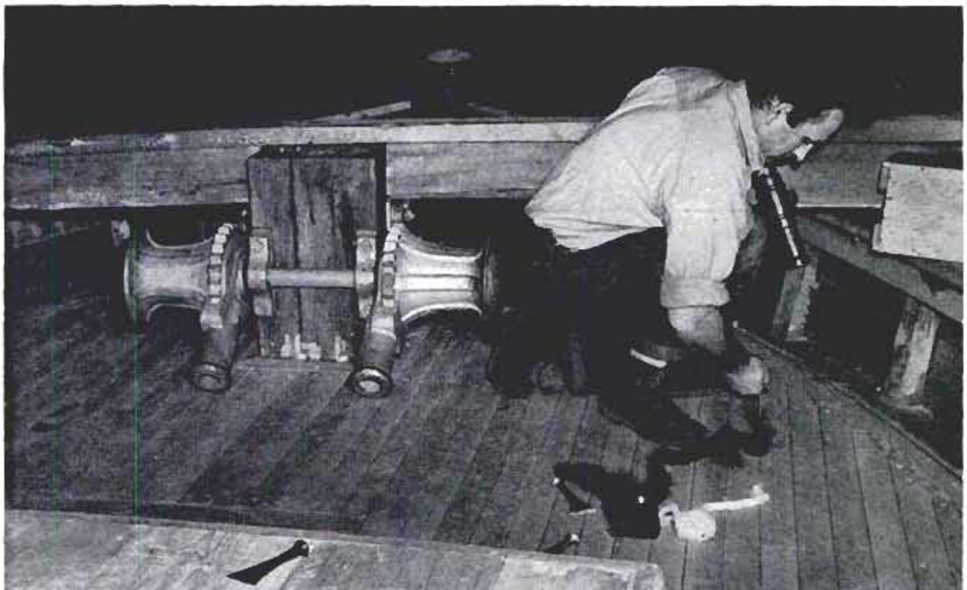
Carr completes calking of deck seams on the forward deck. Behind him is windlass. Cabin top is in foreground
