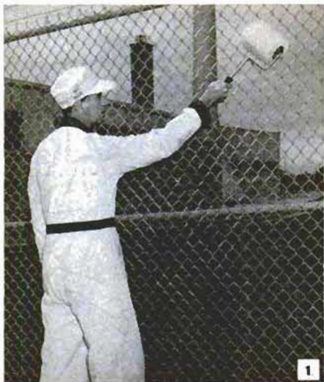
Although it cannot be used for applying rubber or water-base paints, lamb's wool does an excellent job of applying oil-base paints on irregular surfaces such as woven-wire fencing, as shown above
