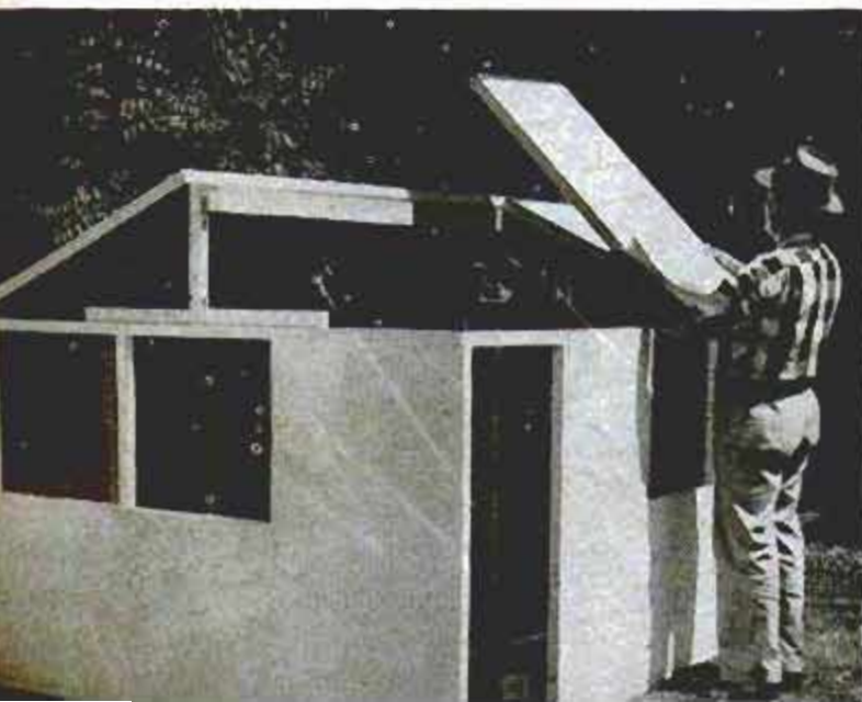
Above, two 1 x 2 members are used to tie each side of the roof together after the panels are all in place. Below, individual roof panels are attached to the ridge board with screws and mending plates, the plates being bent
