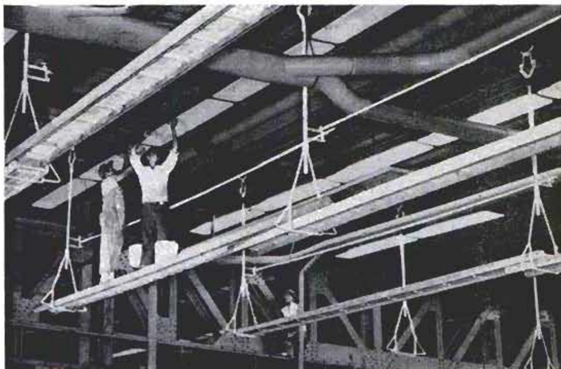
Hanger clamps flange in viselike grip. Pin holds adjusted position. Series of hangers support catwalks
