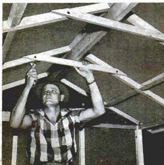
Above, two 1 x 2 members are used to tie each side of the roof together after the panels are all in place. Below, individual roof panels are attached to the ridge board with screws and mending plates, the plates being bent
