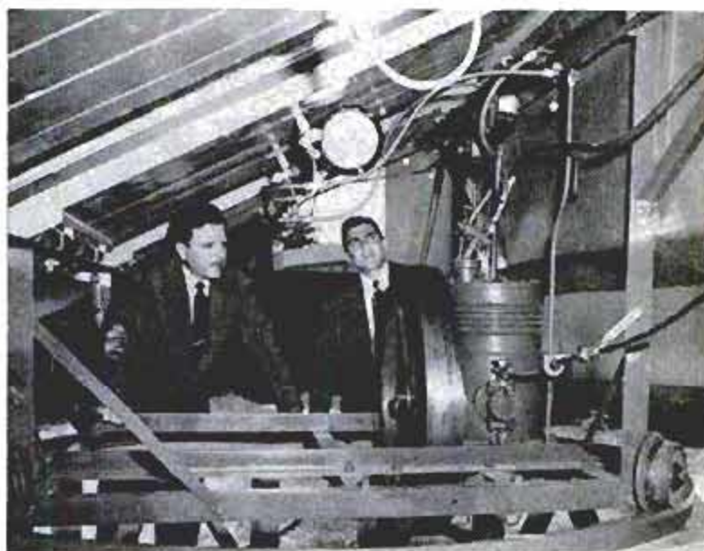
Heating surface of solar pump has 120 square feet, plus side reflectors to concentrate heat. The one-cylinder engine below the panels is run by steam from sulphur dioxide raised to the boiling point by the solar panels. It develops one horsepower
