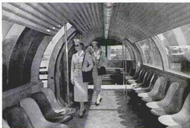
Coach seats 60 and carries 50 standees, is 7 feet high and 8 feet wide inside. It is suspended from power units that run on top of the rail. Pilot model has glass-fiber skin
