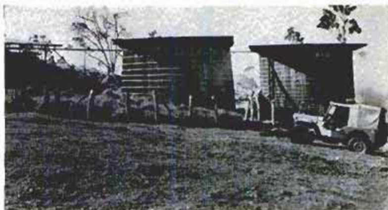
Huge metal roofs have been built on the islands to collect rainwater, which then is drained off into redwood storage tanks and saved for future use. Below, engines of the new water system are started by hand. They pump water up the mountainside
