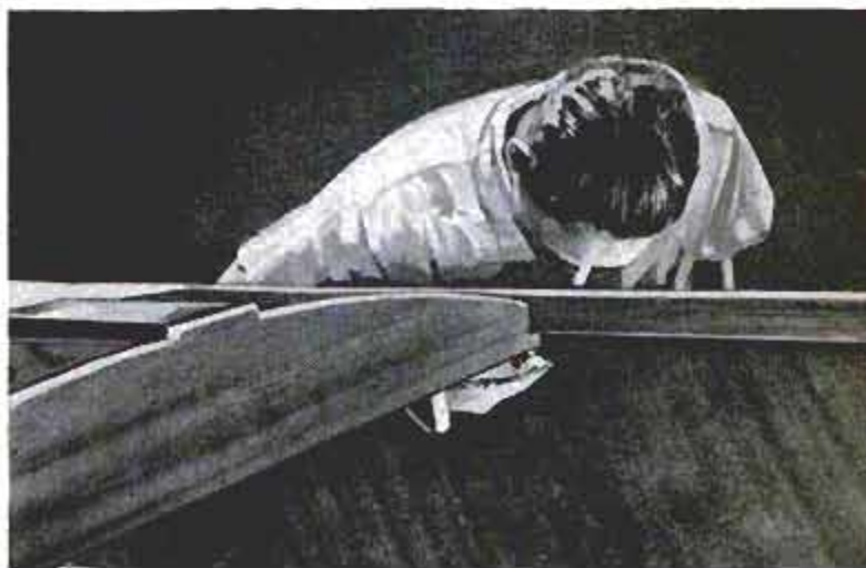
10. Beams of removable decks are attached to underside of cap rails by means of bolts and wing nuts
