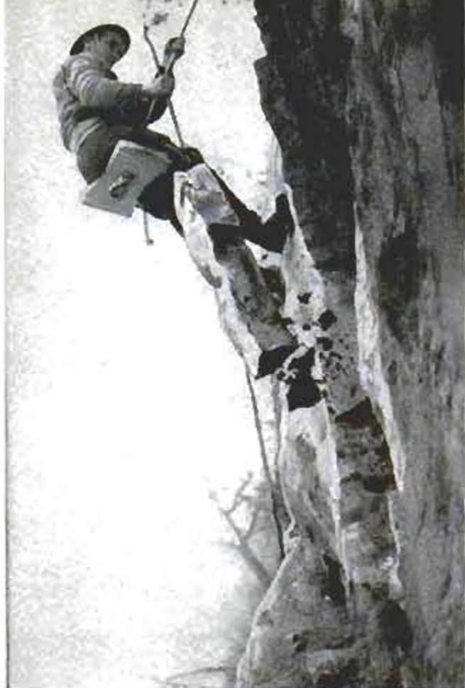
Dangling on the face of the precipice, the workman uses a long steel bar to break away loosened rocks
