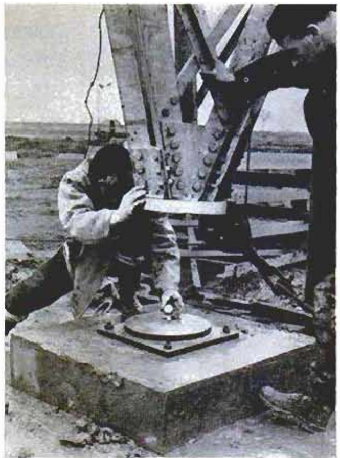
Workman inserts two-inch-thick steel ball into the base plate. Ball acts as rocker bearing between the recessed plates of the mast base and the foundation
