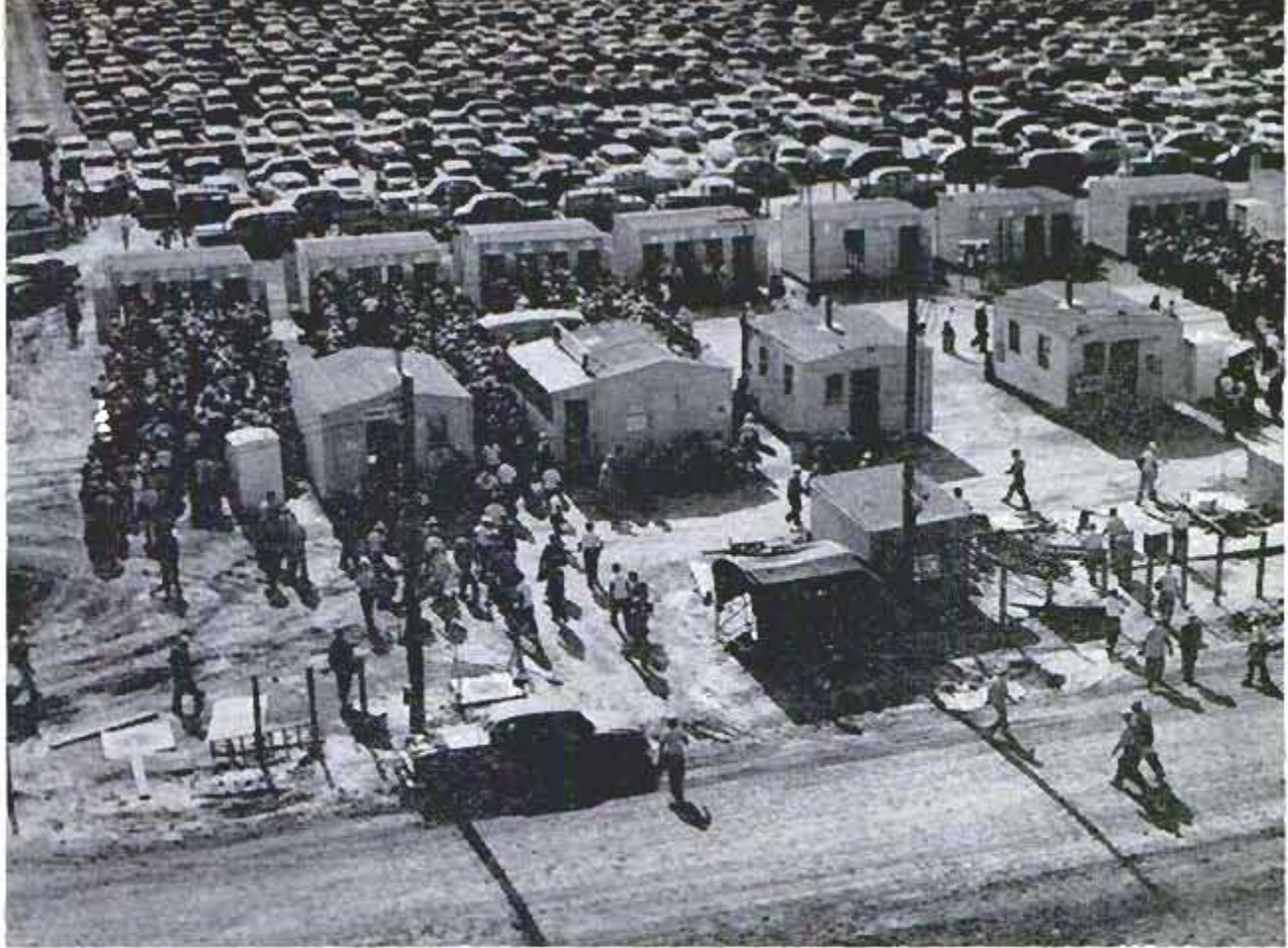
Some 20,000 new workers—plus their families—invaded the area. Here one shift files through time-clock gates
