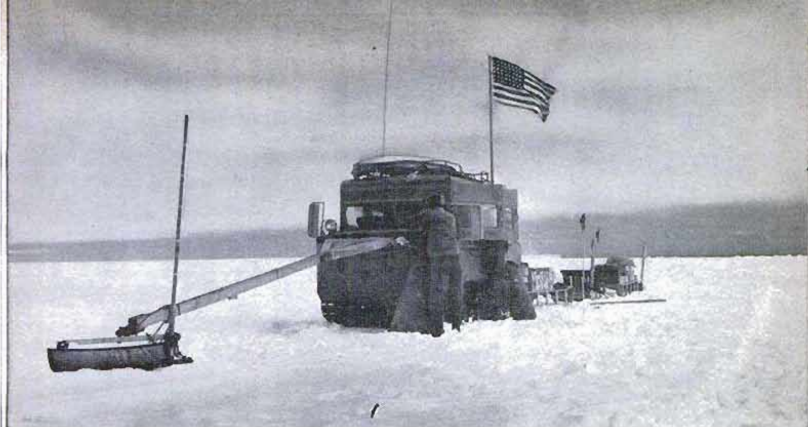
Crevasse detector out front, Weasel with sled train is prepared for 400-mile trip to Marie Byrd Land
