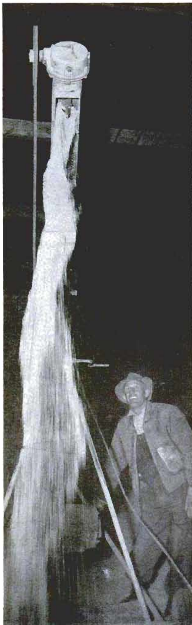
At the left, a portable worm takes the place of shovels in handling grain. Above, automatic scale weighs grain for mixing. Push of button does the rest
