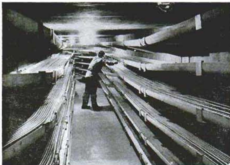
Project required 1600 miles of pipe and tubing, 4600 miles of wiring
