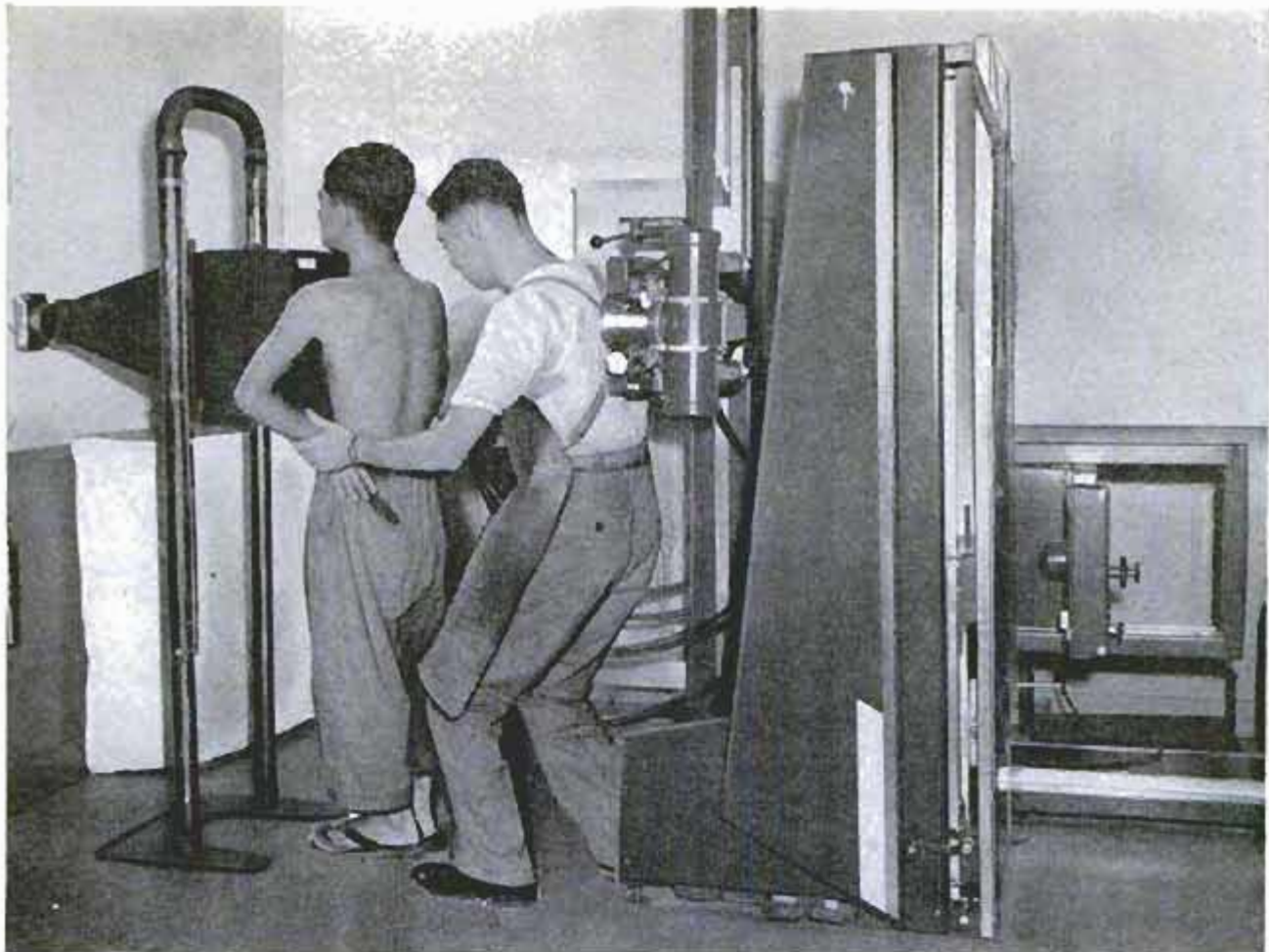
Homemade unit at left photographs fluoroscopic X-ray image of chest. Commercial X-ray source is at right
