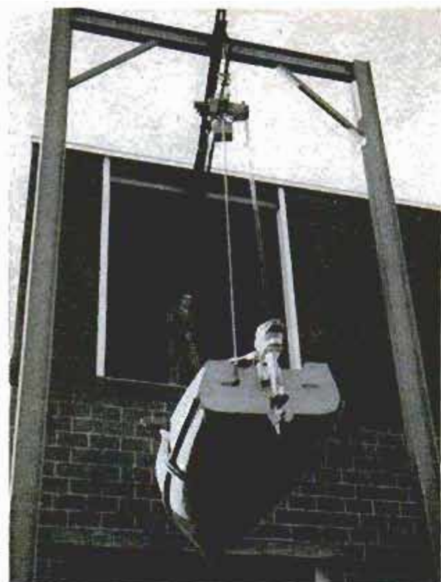
Hoist lifts boats to the second floor of this boat-house, where there are repair and storage facilities
