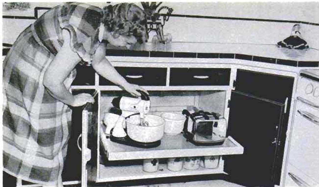
Appliances are always within easy reach when they are stored on roll-out shelf built into kitchen cabinet
