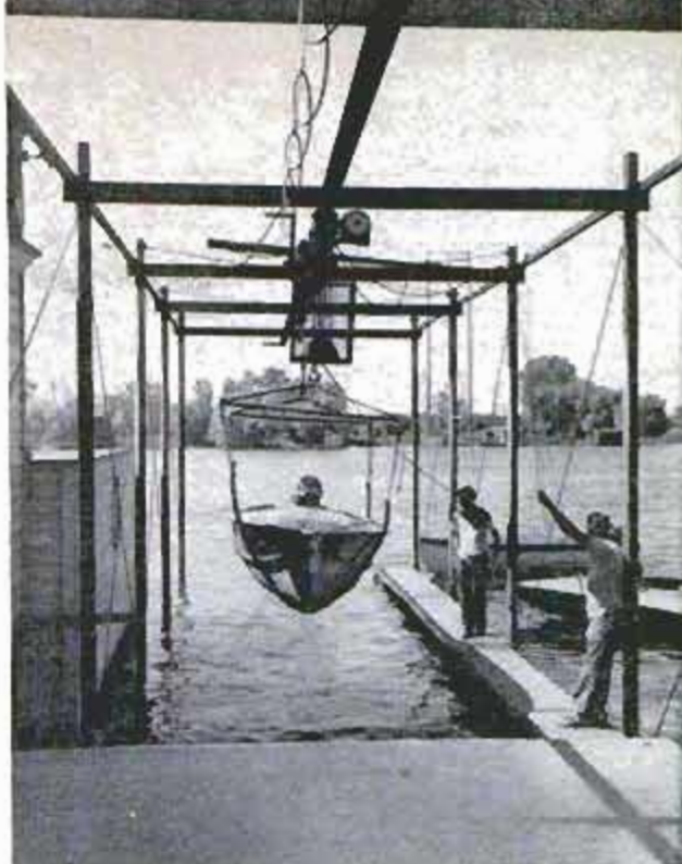
At a Wisconsin marina, boat is lifted in a sling and carried by monorail to the water or storage area
