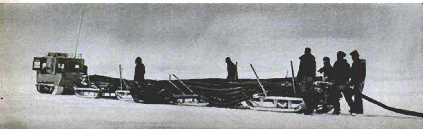
Oil-burning stoves warmed tents used by Seabees at Little America. Forty degrees was considered warm. Below, laying six-mile fuel line to a "tank farm"
