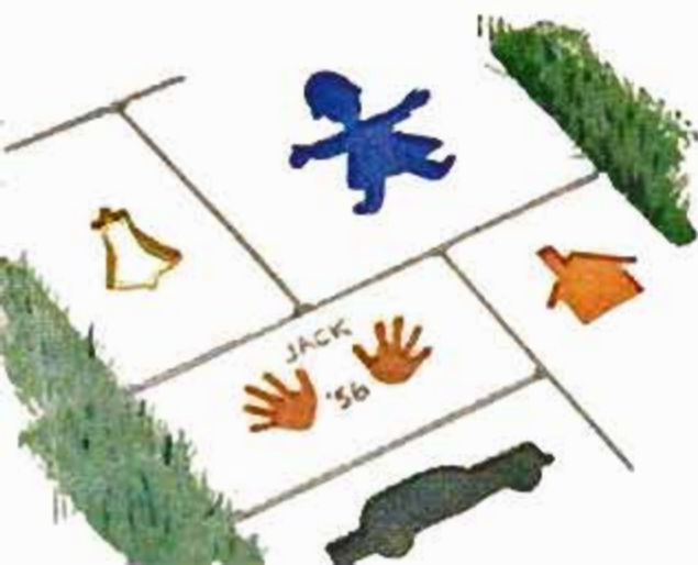
If you want a personalized patio you can cast concrete blocks yourself and impress designs of family interest. Forms of 2 x 2-in. lumber provide 2-in.-thick blocks. Designs are colored with concrete paint if desired. Use premixed concrete to make them
