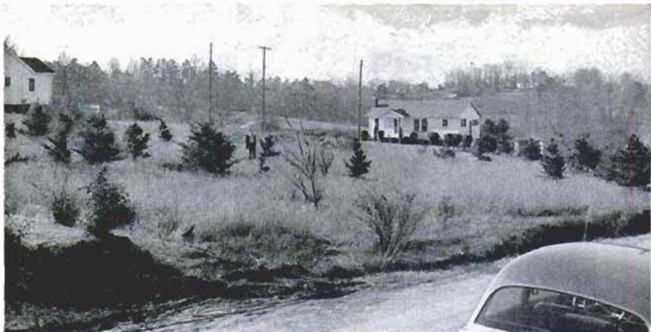
Material excavated for the basement is used as fill to raise the lower level of this lot above the street
