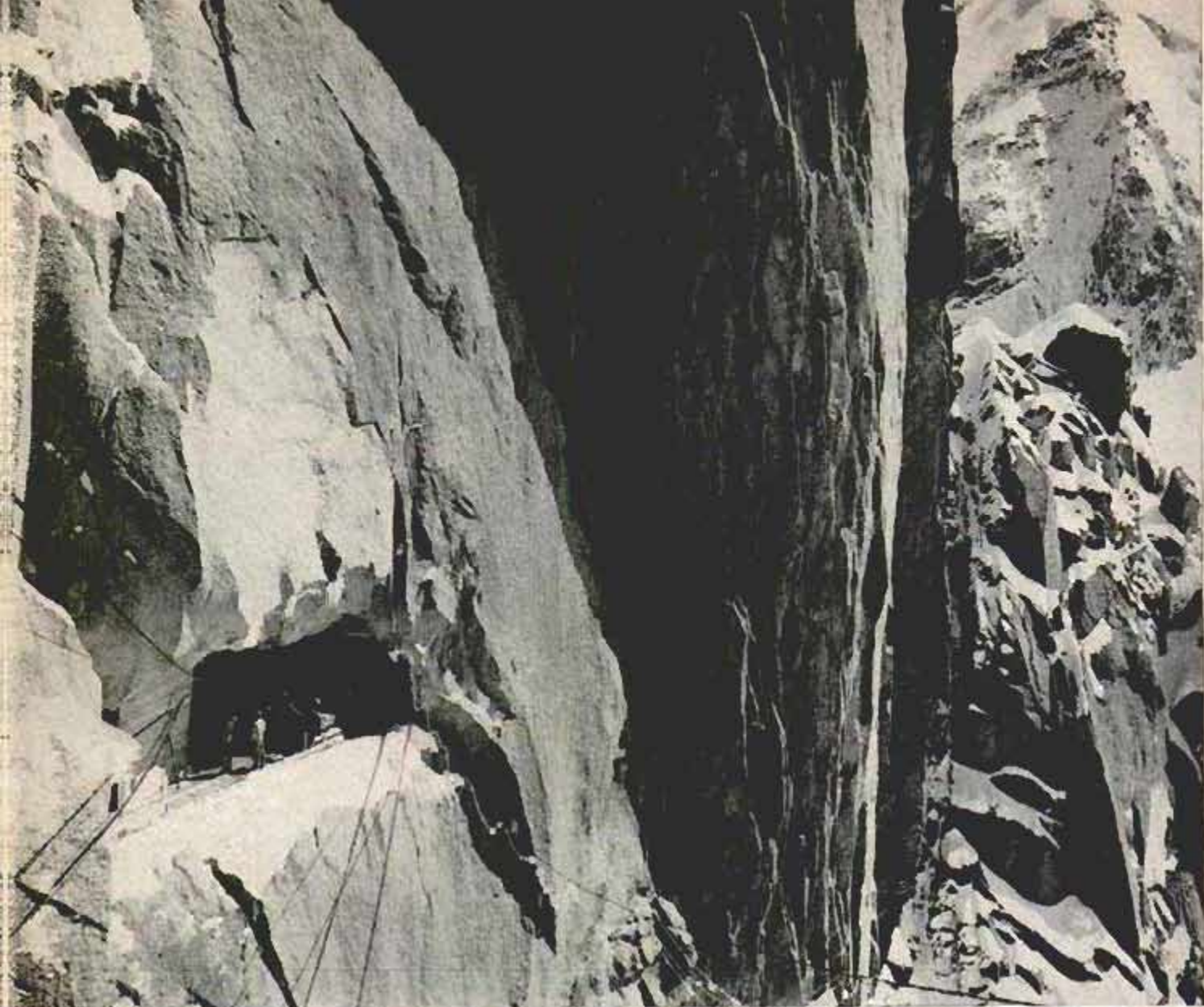
Men worked on edge of precipice to blast tunnel through peak so tourists can view valley on other side
