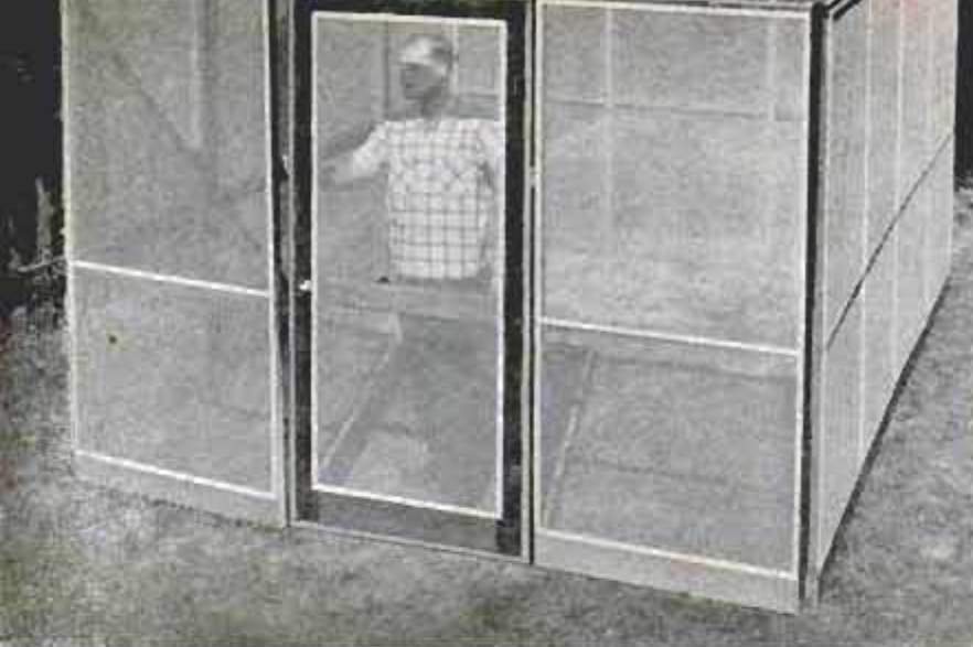
When assembling wall in which door is located, keep it as level as possible to assure doorframe does not twist out of shape. Photo at right shows how tape is stapled over hinged joint on corner sections of house
