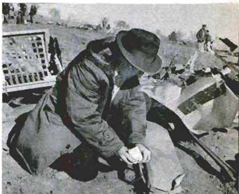
Every large piece of wreckage is tagged to identify it and to indicate where in the wreckage pattern it was found. Pattern often yields valuable information
