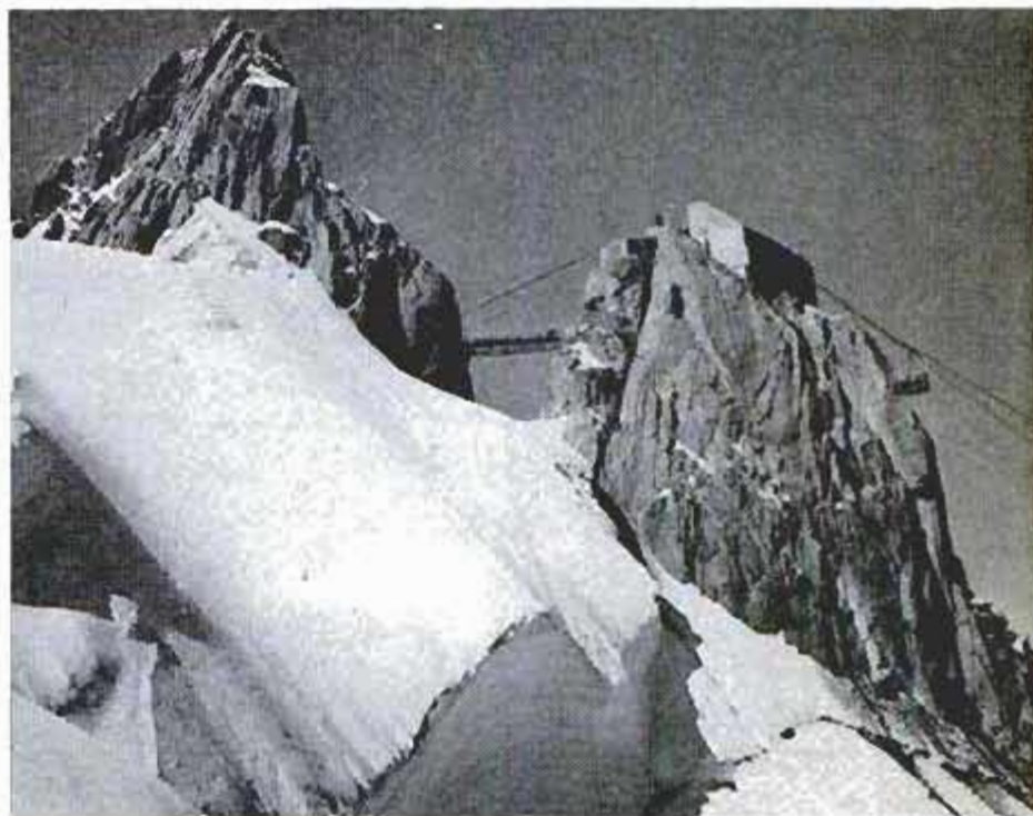
Car approaches North Point of Aiguille de Midi (with hotel). Cableway goes through shaft to steel bridge to South Point
