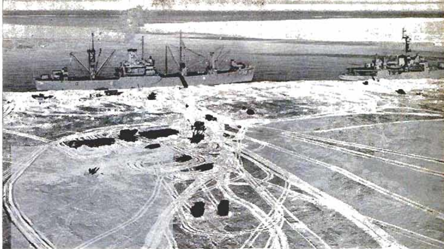
Ships moor to "deadmen" frozen in holes at the edge of Antarctica's bay ice, and supplies move off on sleds
