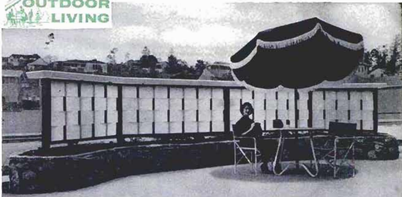
Glass-fiber panels woven around dowels form a fence that both enhances property and serves as wind screen
