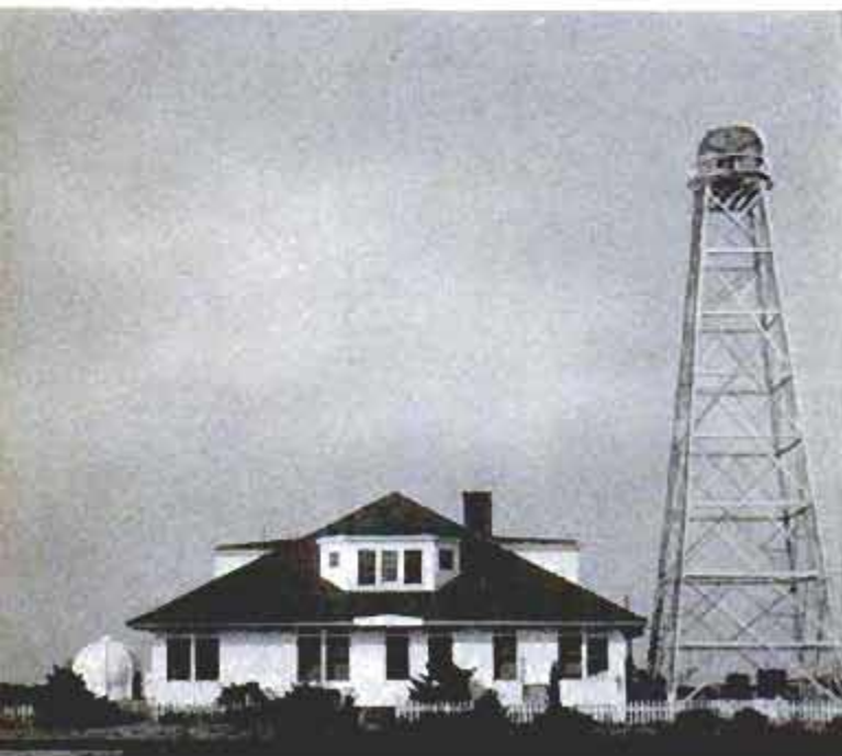
Below, long-range-radar station at Hatteras is an important link in chain. Dome houses instruments
