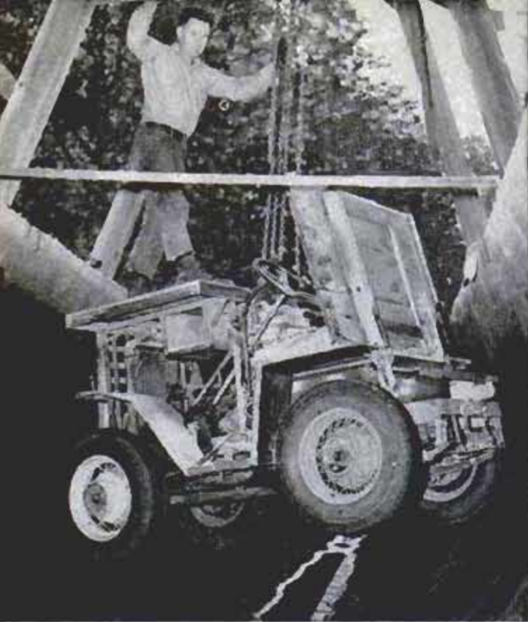
Car is hoisted to the widest point in the tube and turned around with aid of A-frame, block and tackle
