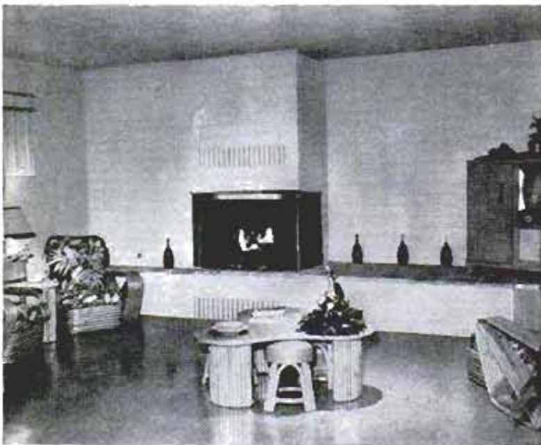
This fireplace with its raised hearth was built around a metal form. Note warm and cold-air inlet and outlet in the masonry
