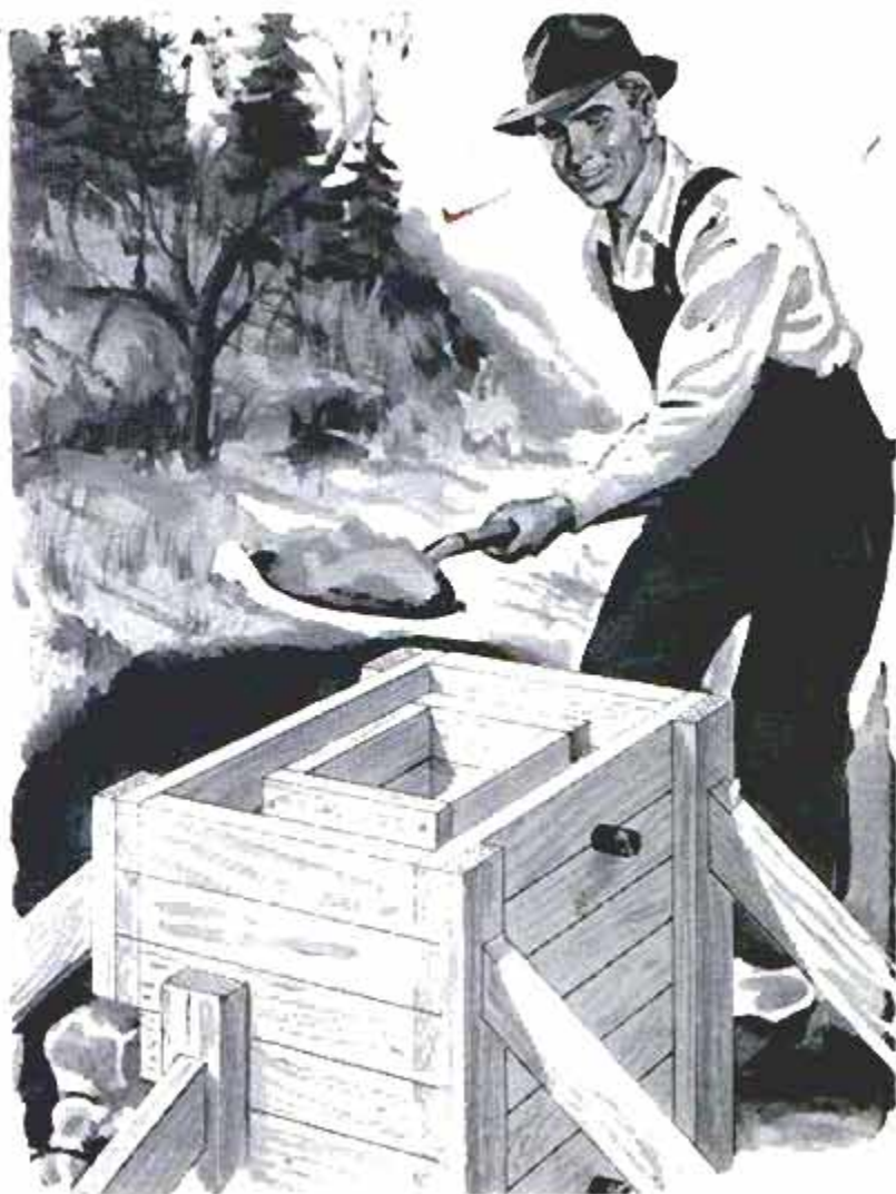
Nipples for the overflow and delivery pipes should be positioned in the forms at the desired levels before the concrete is poured
