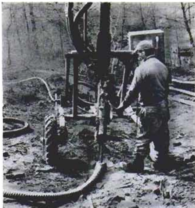
Drill rig, right, has hose leading to big "vacuum cleaner" above which packages dust for disposal
