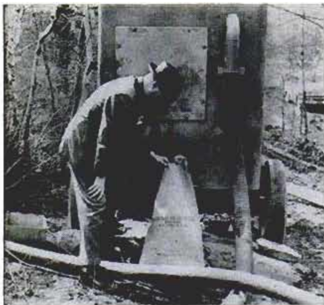
Drill rig, right, has hose leading to big "vacuum cleaner" above which packages dust for disposal
