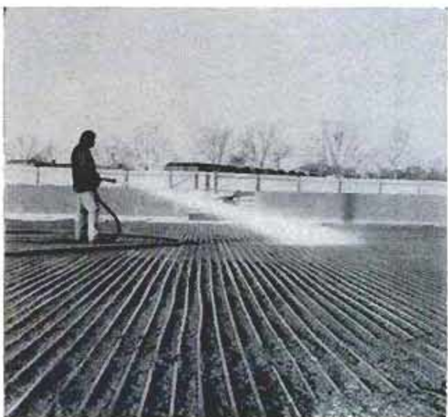
Above, truck carries four compressors to provide 140 tons of cooling for 85 by 185-foot rink. Below, after pipes are covered with sawdust, water is sprayed on to build a layer of ice three to four inches deep
