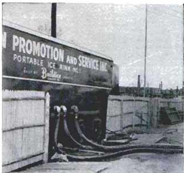
Above, truck carries four compressors to provide 140 tons of cooling for 85 by 185-foot rink. Below, after pipes are covered with sawdust, water is sprayed on to build a layer of ice three to four inches deep
