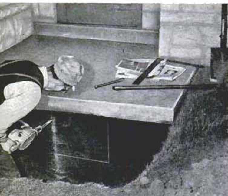
Above, cut manholes into any areas completely enclosed by concrete foundation walls. Remove all wooden form members. Below, after treating soil under floor, fit opening with grille to provide access
