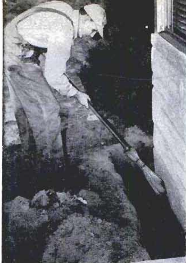
After trenching around foundation to depth of 12 to 30 in. earth is saturated with a special insecticide
