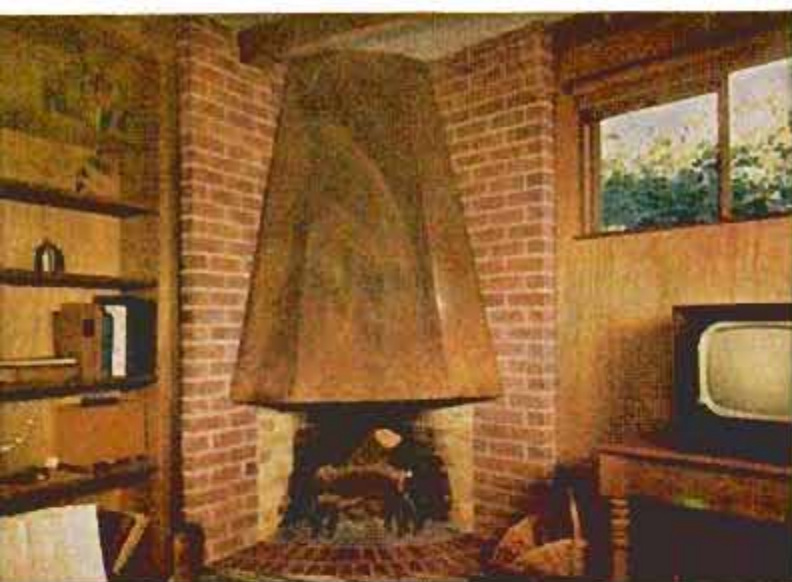
Above, copper hood replaces considerable brickwork in this corner-type fireplace. Below, this fireplace is part of a curved living-room wall of Arizona fieldstone. Shelf-type hearth is black marble
