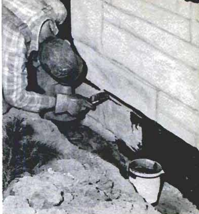
When applying hot tar to foundation walls be sure that coating is brushed to uniform thickness
