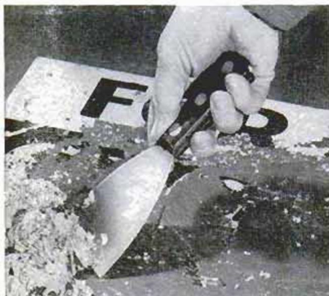
Above, when removing the paint film from a flat surface begin at the center and work out to the edges. Below, by working from the center out you avoid scraping loosened material over wet surface of work
