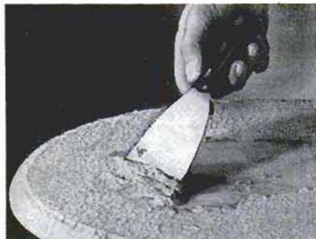
Above, when removing the paint film from a flat surface begin at the center and work out to the edges. Below, by working from the center out you avoid scraping loosened material over wet surface of work
