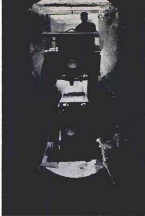
Jitney plunges into tunnel as it makes first canal inspection trip after fall water shutoff
