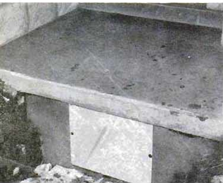
Above, cut manholes into any areas completely enclosed by concrete foundation walls. Remove all wooden form members. Below, after treating soil under floor, fit opening with grille to provide access
