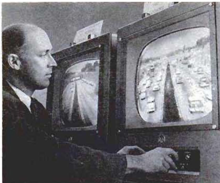
Above, a traffic engineer watches the screens of two television monitors, prepared to direct emergency operations the moment an accident or slowdown occurs. Below, in the tests cameras were mounted on towers to determine best height for observing Freeway traffic
