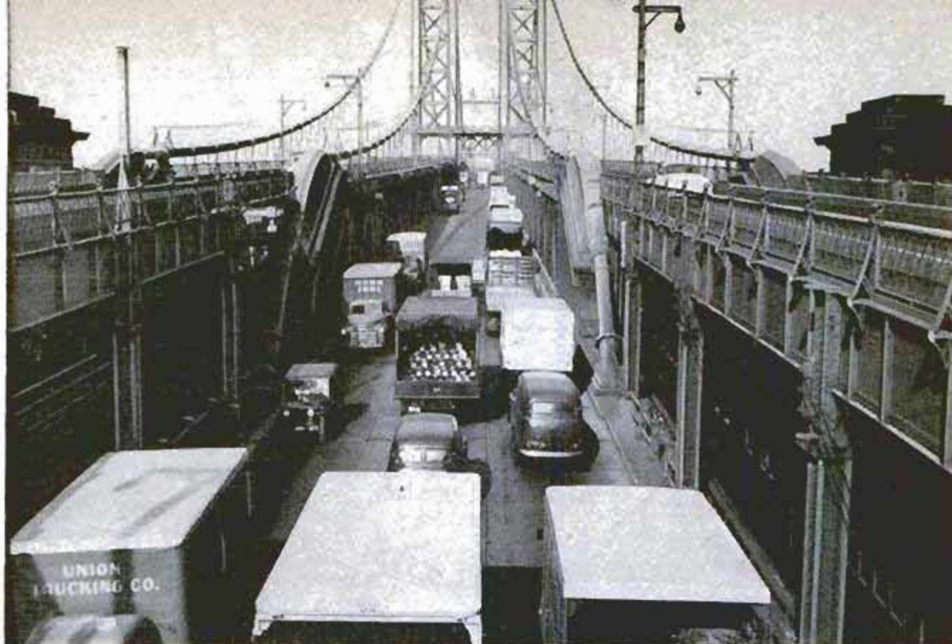
Automotive traffic rides on two decks of roadways. Double subway tracks flank each side of lower level
