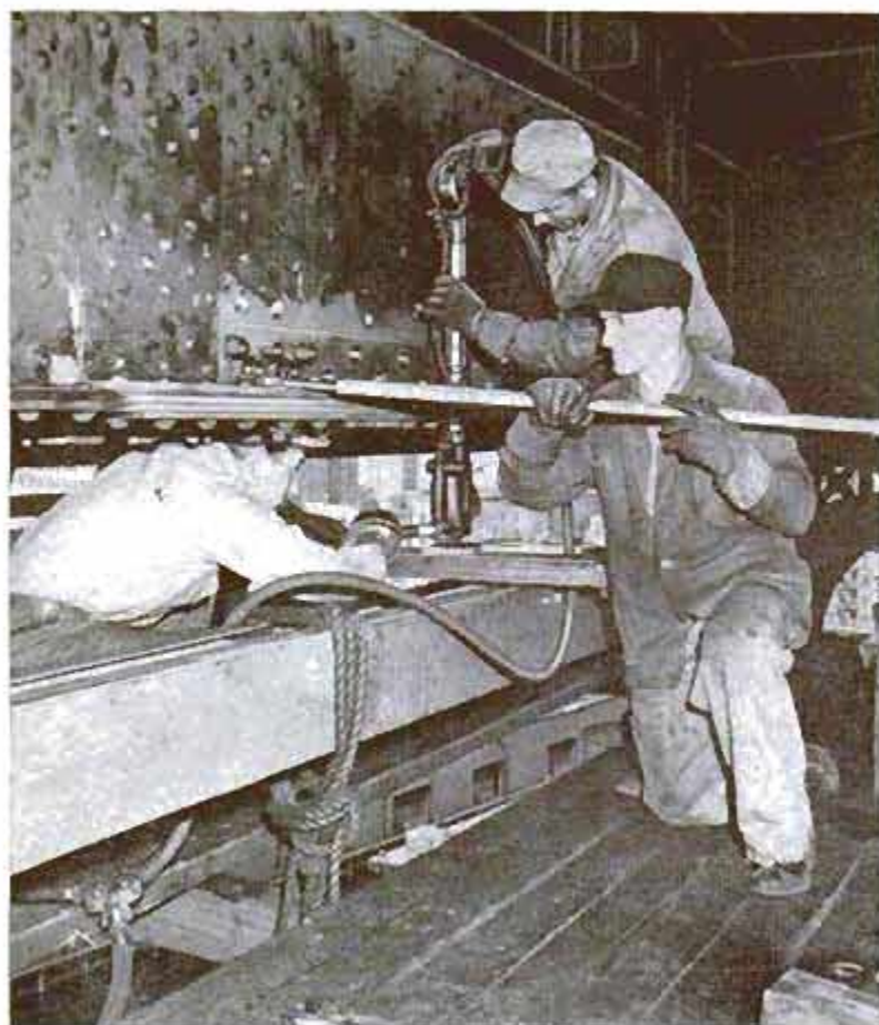
Bridge painter rides spider staging that carries him up and down. Below, plate is bolted into position to repair break in truss. Work is done at night to avoid disrupting traffic. The total revamping will take 2½ years and will cost $30,000,000
