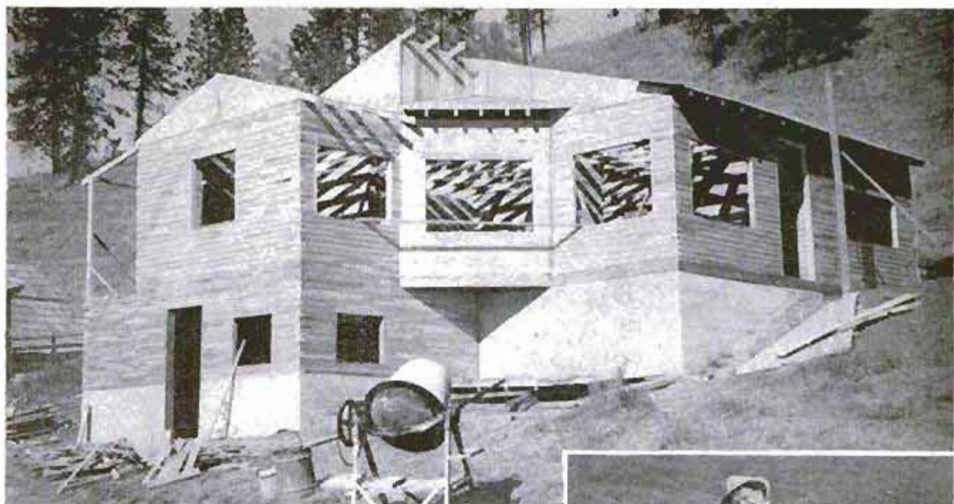
Shell of the house was made of scrap two by fours pinned together with nails. Right, interior walls were the same
