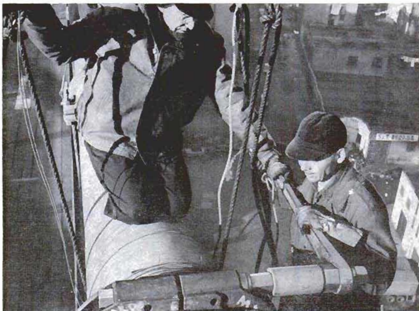
Workmen testing strength of the Manhattan Bridge tighten bolts of cable band in squeeze test of main cable
