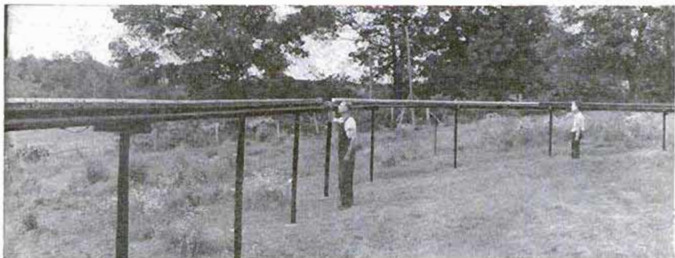
Trains run outside on this long trestle. Guard rail protects them from falling off in case of derailment
