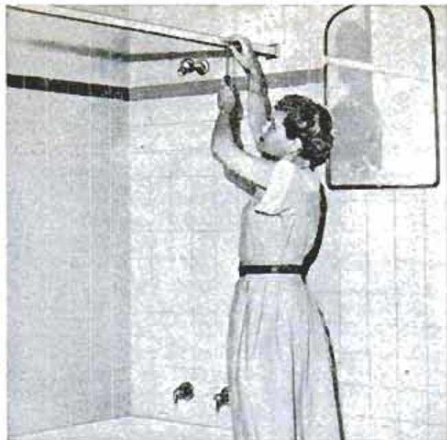
Screwdriver tightens adjustable track for snug fit
