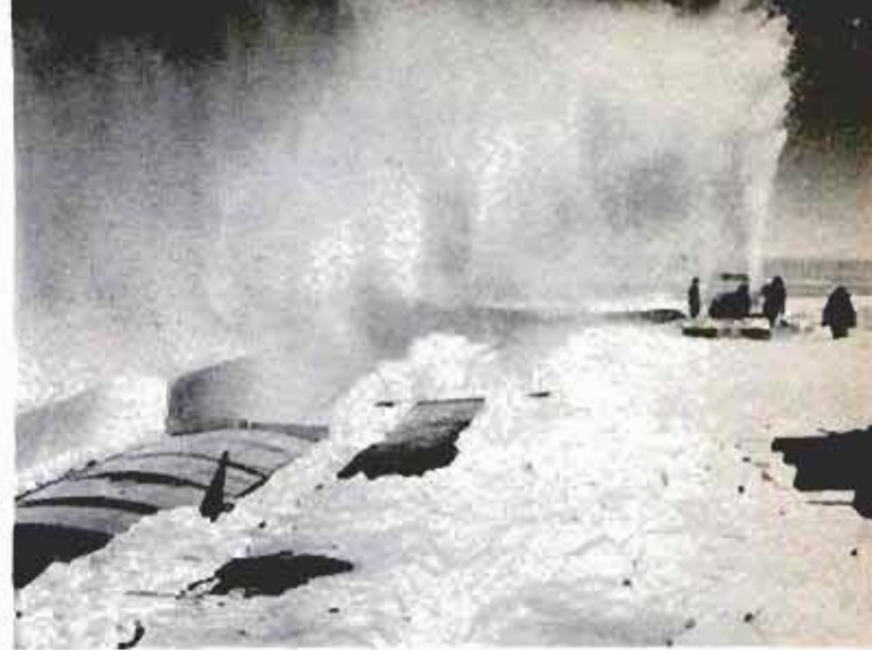
Mechanical snow blower follows alongside the trench after forms have been laid, covering them with snow
