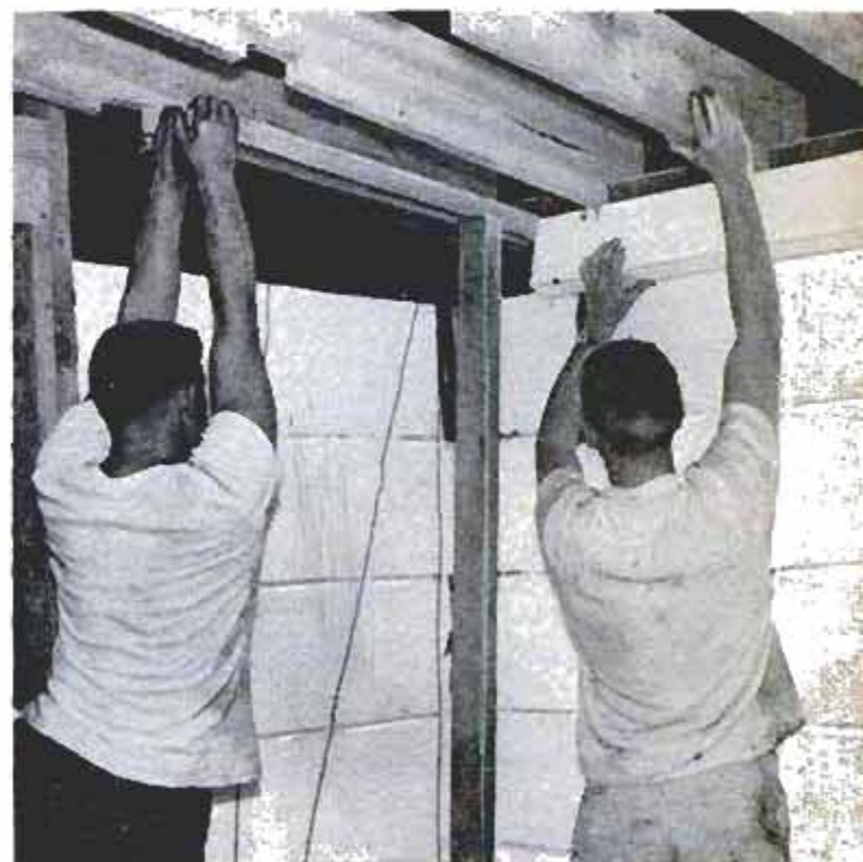
Workmen fit top board of Styrofoam into place as the last step before side wall is wired and sprayed
