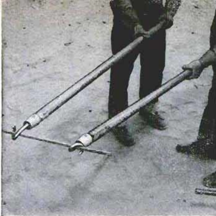
"Pigtail sticks" are used for holding, raising or moving hot 11,000-volt and 16,000-volt power lines
