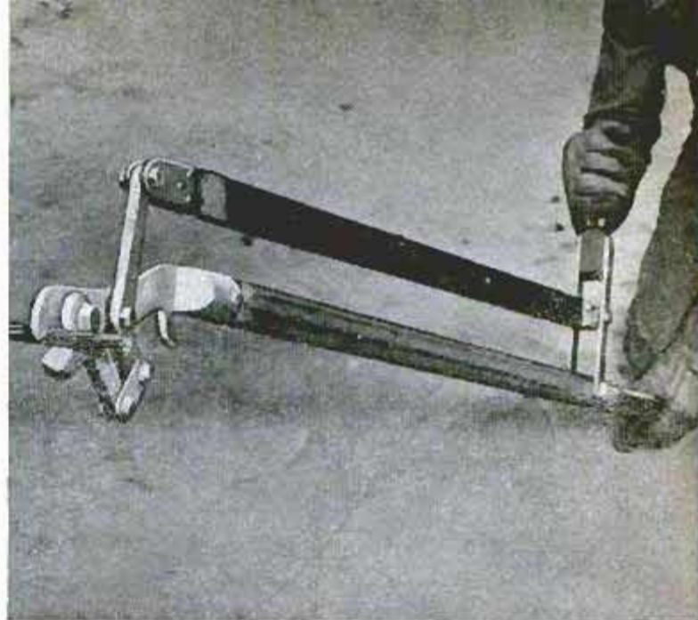
Hot-stick cutters can nip off heavy wire. Extremely heavy wire is usually sawed with hot-stick hacksaw
