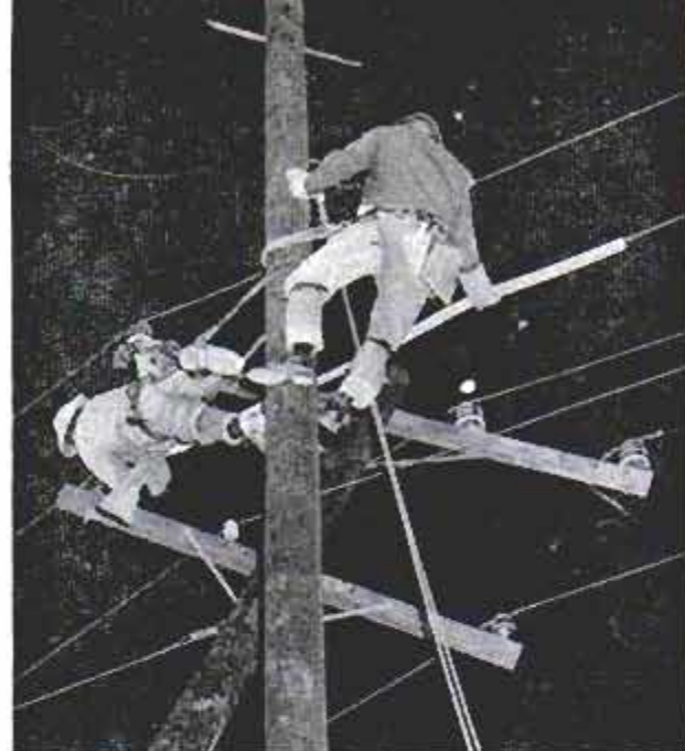
Linemen, above and left, take on job of transferring hot lines from pole snapped off at base to new pole
