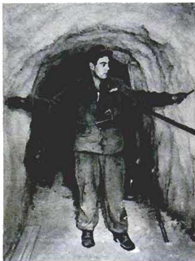
Experimental tunnel dug in ice at edge of icecap is four feet wide. It was dug by hand with picks
