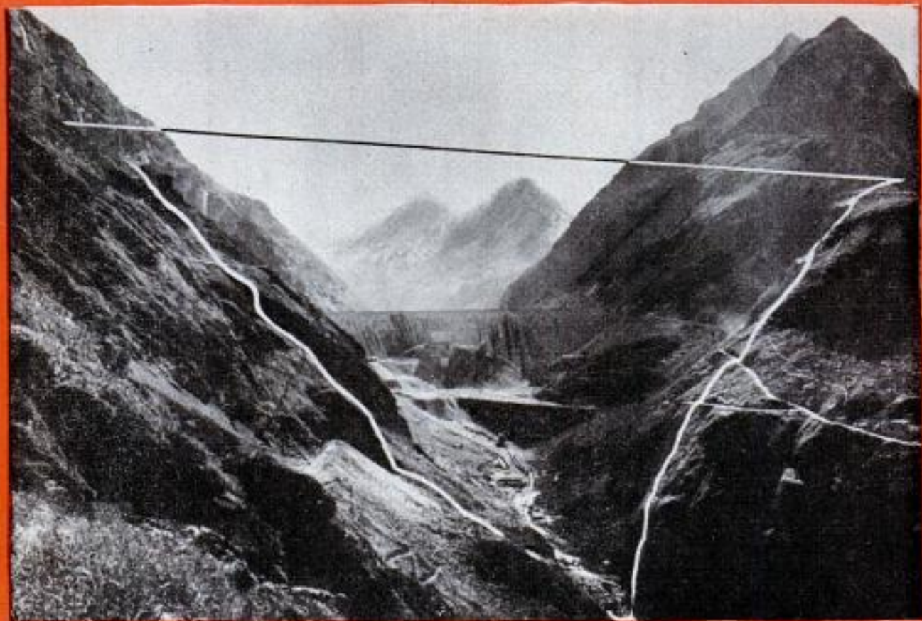
Outline of new dam is shown on picture taken of dam site before work began. Dam will be 2300 feet across top
