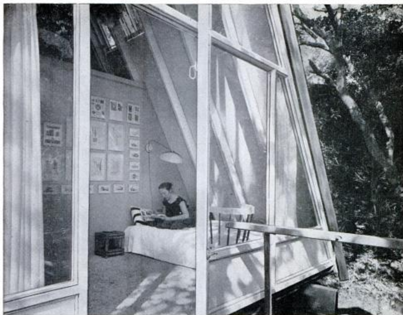
Bedroom was added to rear of basic precut house with two four-foot sections. Dimensions are eight by thirteen feet. Interior walls provide privacy but do not reach peak of roof. House has "tree house" effect
