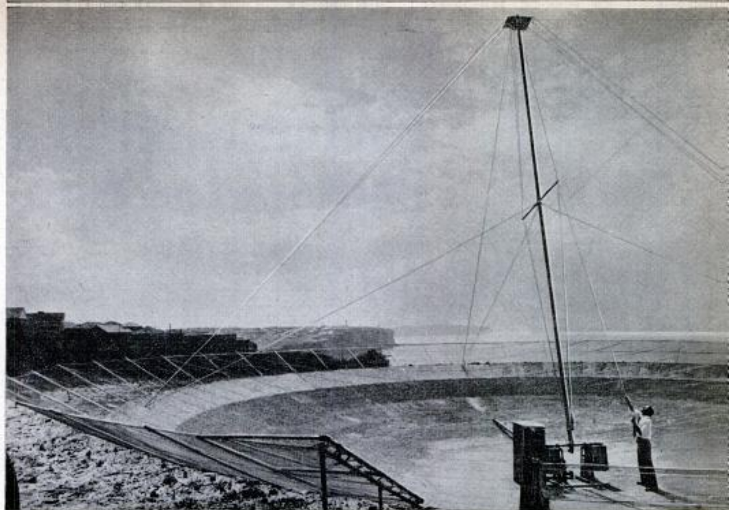
Radio telescope on cliff near entrance to Sydney Harbor is mounted in bowl hollowed out of the ground
