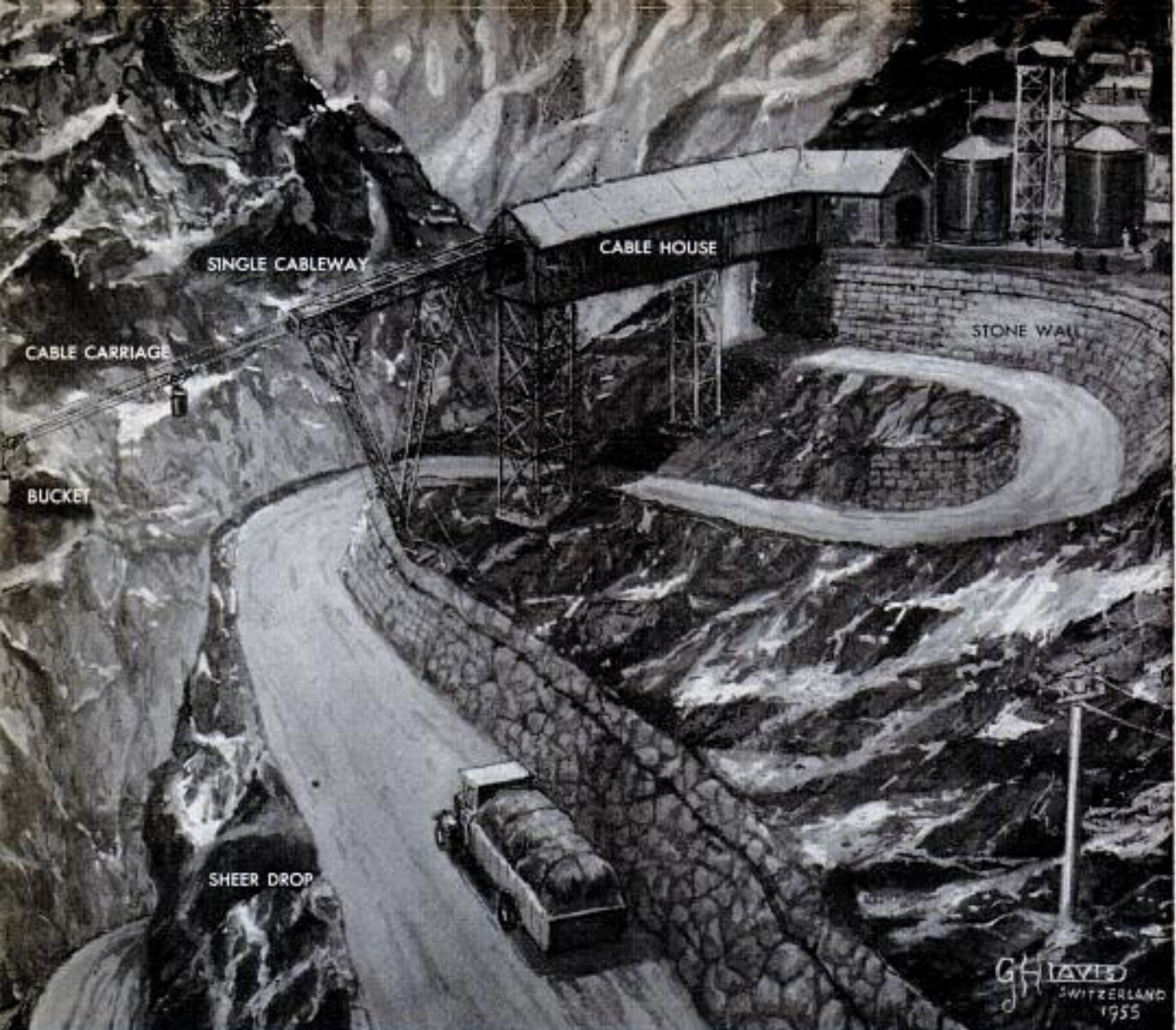
Thousands of tons of material must be brought up the side of the mountain from valley on this twisting road
