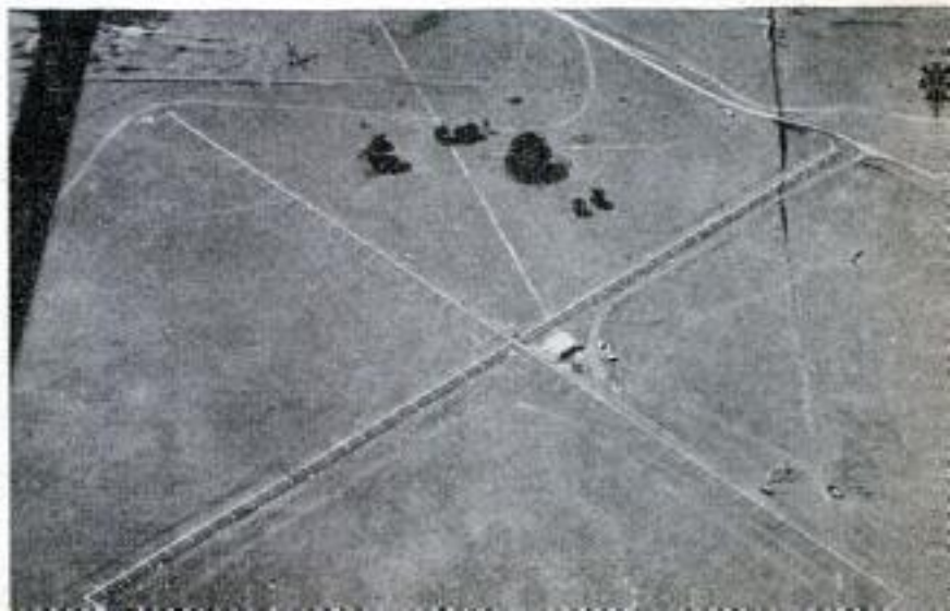
Arms of Southern Cross, Australia's largest radio telescope, are each 1500 feet long. Operating frequency is 85 megacycles
