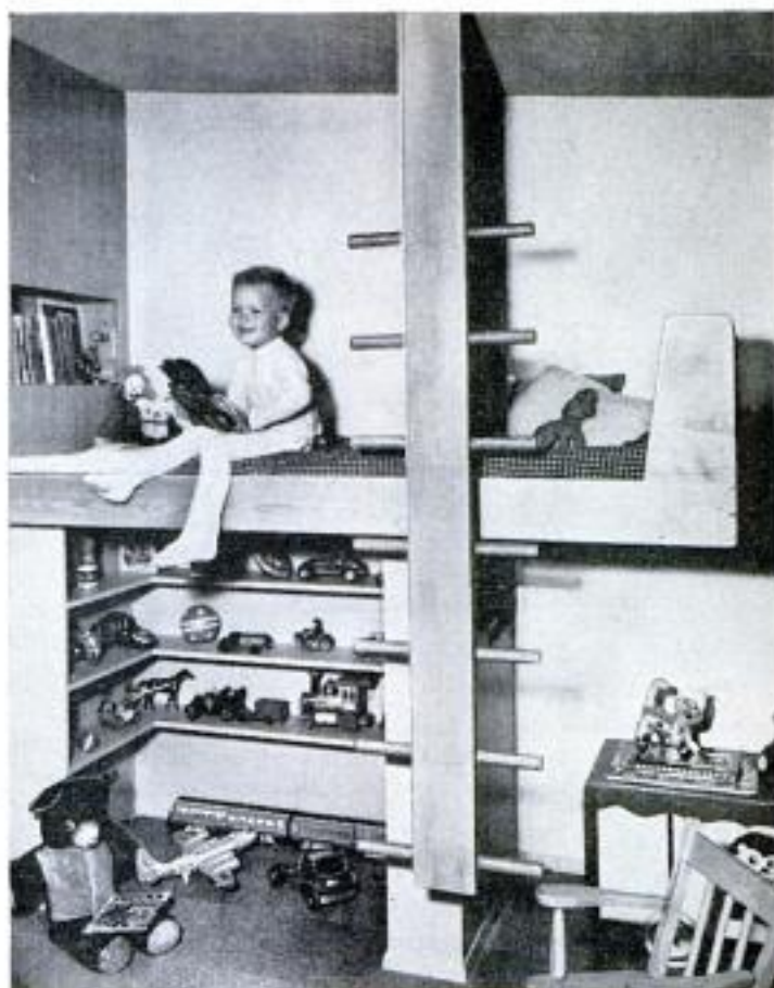
Dowel-rung ladder serves double duty in providing guard rail for bed. Note the bookcase that is built in at foot of bed
