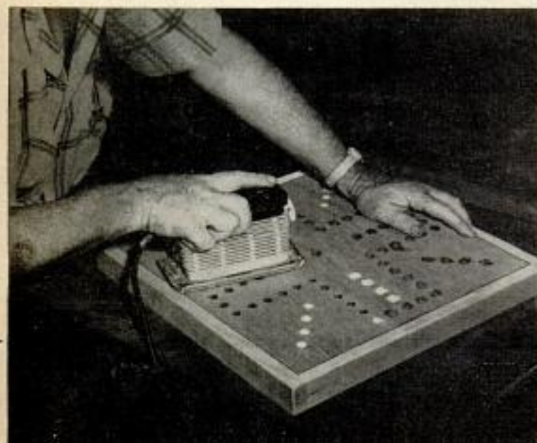
Above, holes are spotted 1 in. apart and drilled with \frac{1}{2} or \frac{3}{8} -in. bit just deep enough to retain marble. Board is sanded to remove pencil lines after drilling and again after painting holes, as below
