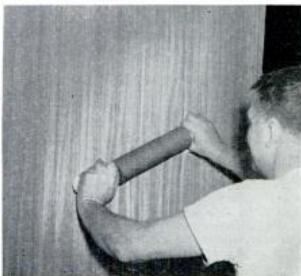
Laminate edges not covered with molding are smoothed with single-cut file, as above. After panel is in place it should be rolled with rolling pin or tile roller to assure a firm bond to the wall surface
