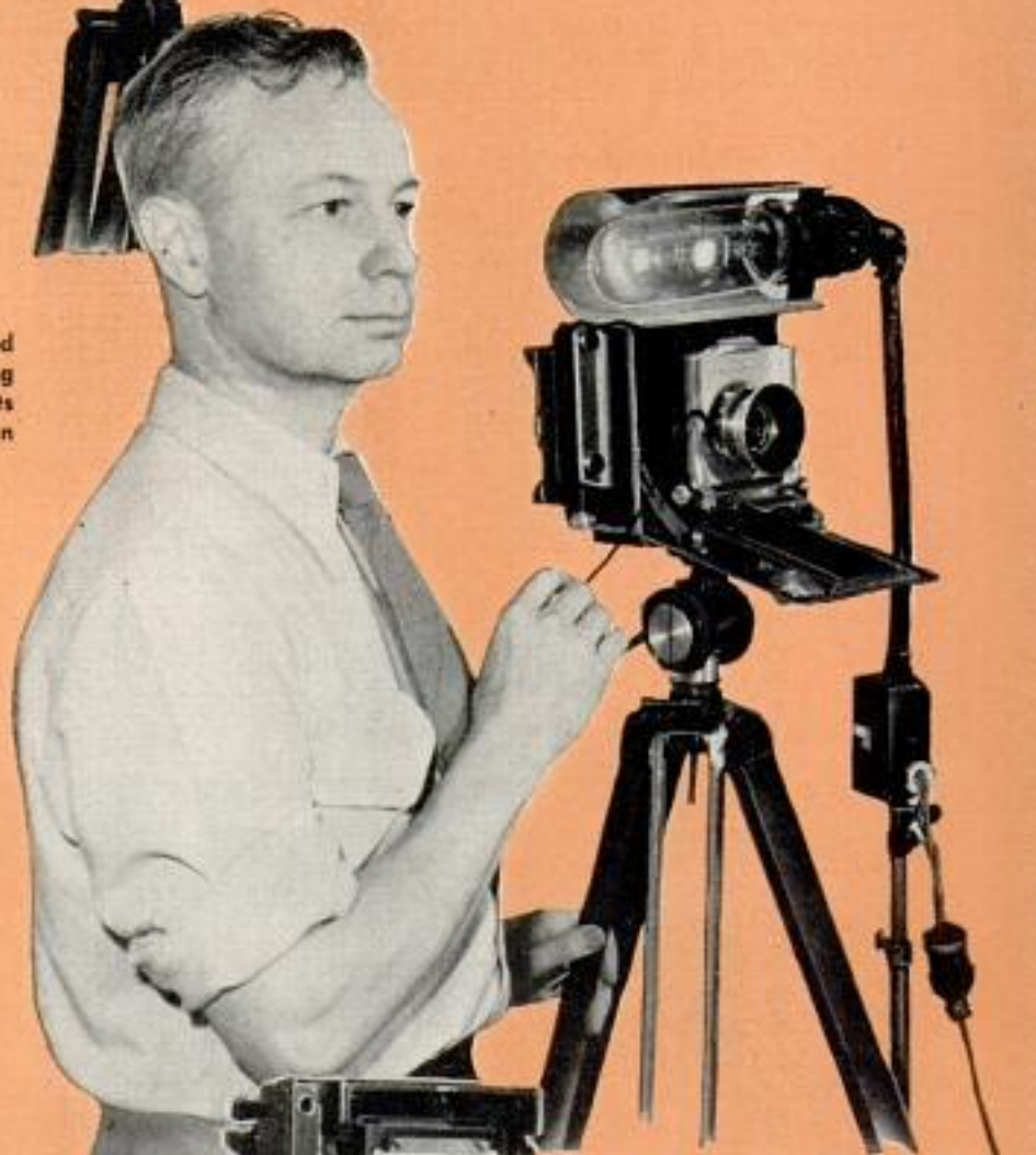
Hine shoots 4-by-5 stereo photos with standard press camera by using two lenses on board with rear divider
