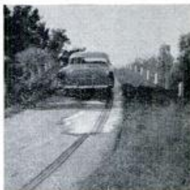
5 Car with new differential goes up hill without any hesitation. Closeup, below, of tire tracks is proof wheel did not slip on soap
