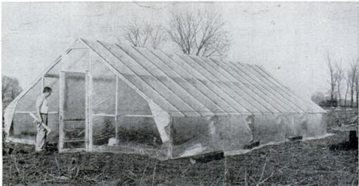
Purdue expert erected this plastic greenhouse on his farm. Structure half this size can be built for $75
