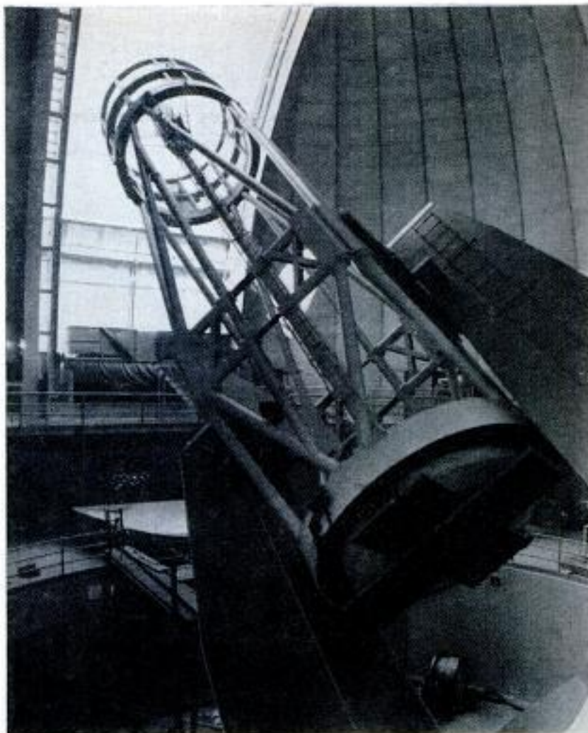
Open-framework section of the telescope is 53 feet long. Below, Dr. C. D. Shane, director of Lick Observatory, and a technician inspect a working model of the new instrument. The 120-inch telescope will be the second largest in the world and will have a range of 900 light-years
