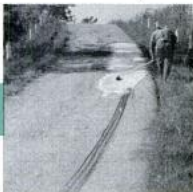
4 Strip is "re-iced" to duplicate original conditions. Soap is so slick, workman can't walk on it
