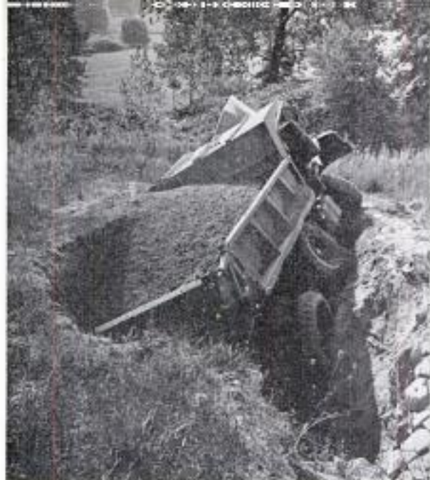
Truck with capacity load of soil ended up in this gully after its brakes failed. Accidents are few
