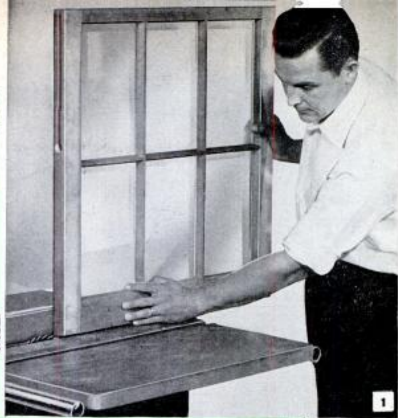
Circular saw makes easy work of grooving each sash
