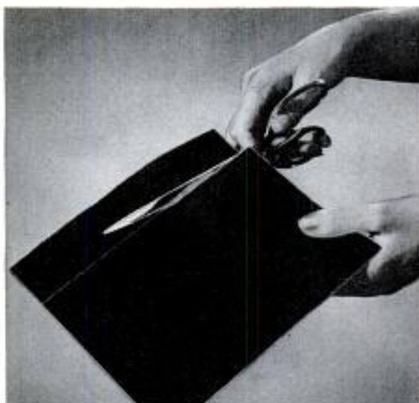
Above, cardboardlike tile is easily cut with regular scissors, cutting through from rear side. Below, paste filler, same color as tile, is used to fill any tile joints that might not be tight-fitting
