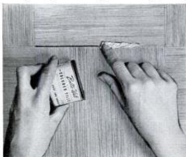
Above, cardboardlike tile is easily cut with regular scissors, cutting through from rear side. Below, paste filler, same color as tile, is used to fill any tile joints that might not be tight-fitting
