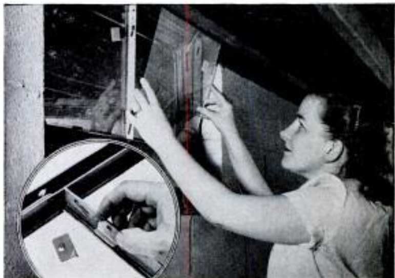
NO-PUTTY WINDOW has a new-type clip centered at the bottom of each pane and two on each side. A tight joint is maintained between glass and sash with felt gasketing. Requires no special skill to install The Donley Brothers Co., Miles Ave., Cleveland 5, Ohio
