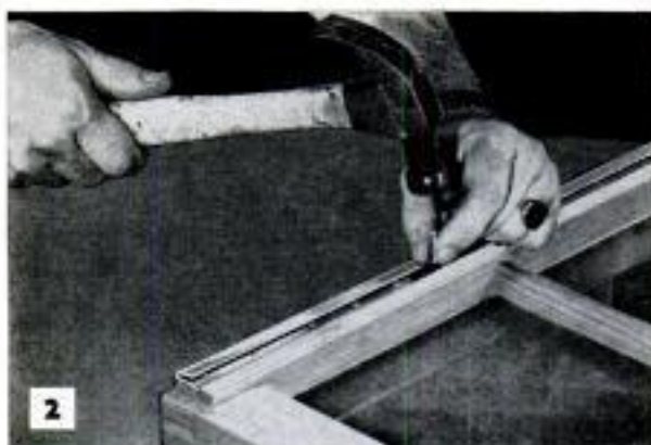
2 Interlocking hook strips are nailed to beveled check rails to seal opening between upper and lower sash
