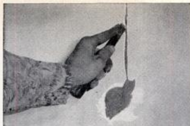
1. Use a chisel to open crack slightly, insuring good bonding surface, before applying Spackling compound
