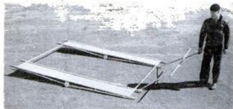
Helicopter settles to rest on canvas "bed" without damage to pontoons. Below, wheels permit landed helicopter to be towed
