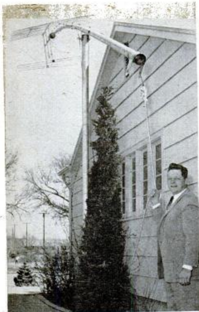
One hand on rope, Orlin Trego, owner of Razien mast, shows how easy it is to balance the 800-pound load
