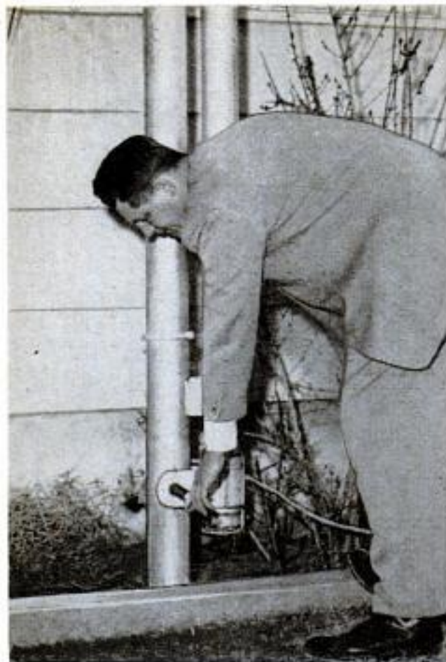
Pin in base is removed so mast can be tipped over for repairs. High winds may necessitate adjustments
