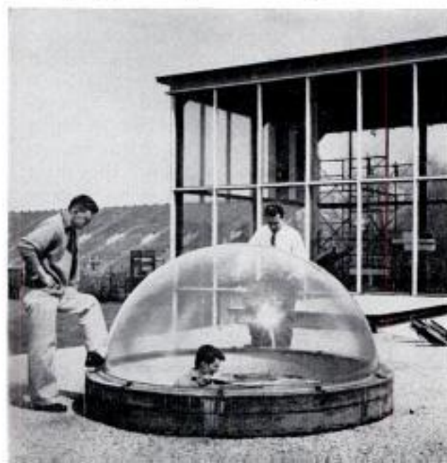
Panels of shading material close off a model room. Cardboard man shows how sun would strike human in the full-size room. Below, plastic bubble in roof offers plenty of sunlight for checking a house model
