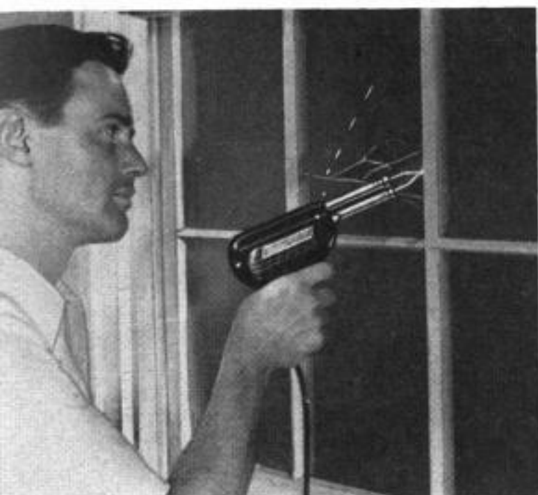
Cutting tip also is useful for softening hardened putty. Removes putty quickly without damaging wood
