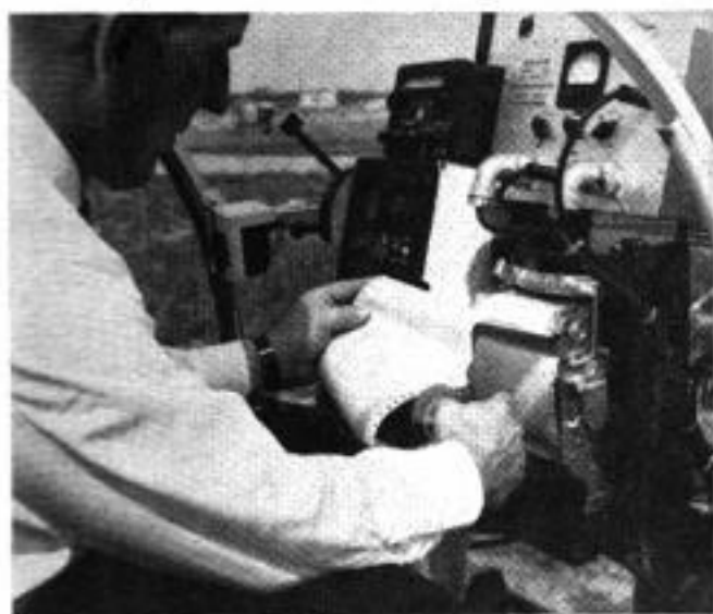
Graph paper rolls out of a recorder in the helicopter. Peaks in graph line indicate increased radioactivity
