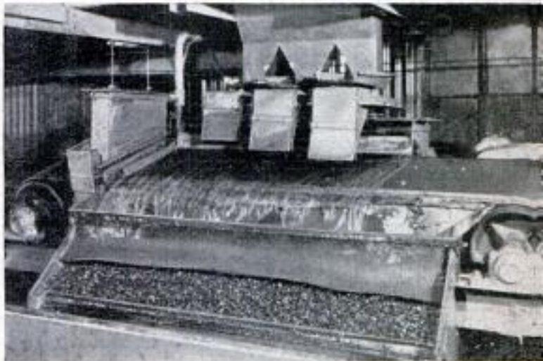
Gravel suspended in heavy liquid washes across grease belt. Diamonds sink, stick to belt. Electrostatic separator, below, relies on conductivity differences
