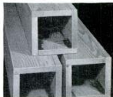
New square columns to replace round ones are made as above
