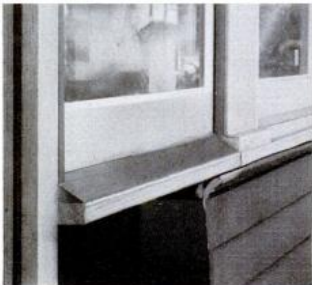
Photo below shows how sills directly above compartments are fitted with triangular-shaped blocks to drain water away from compartment door. See Fig. 7
