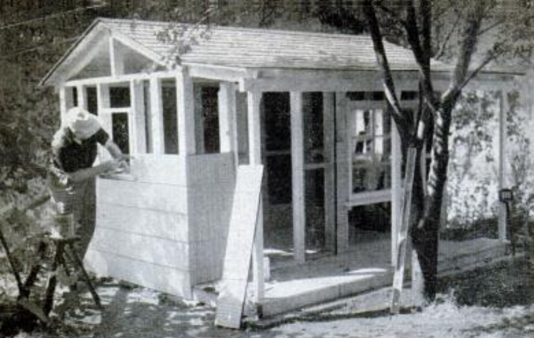
Using insulating siding saves both money and installation time because it forms the outer weather-resistant surface and the exterior wall at one time
