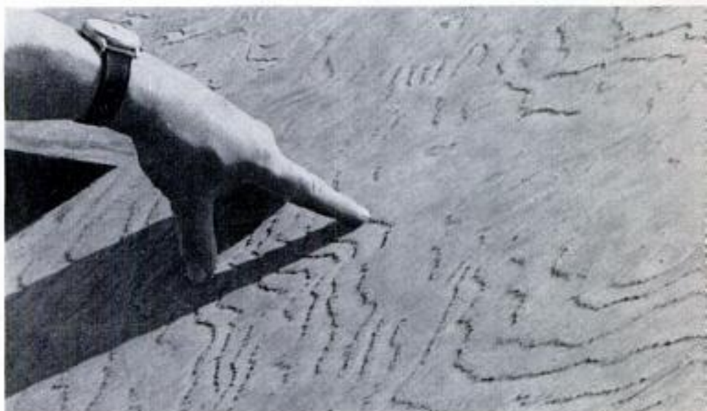
Etched plywood is used for the concrete forms of the lodge. Concrete takes on the wood's grain pattern. Texture is enhanced with special stain
