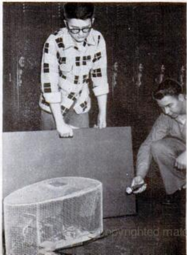
The Snail, a mobile wire-caged machine, follows a light beam. Inventor Versal Cross holds flashlight
