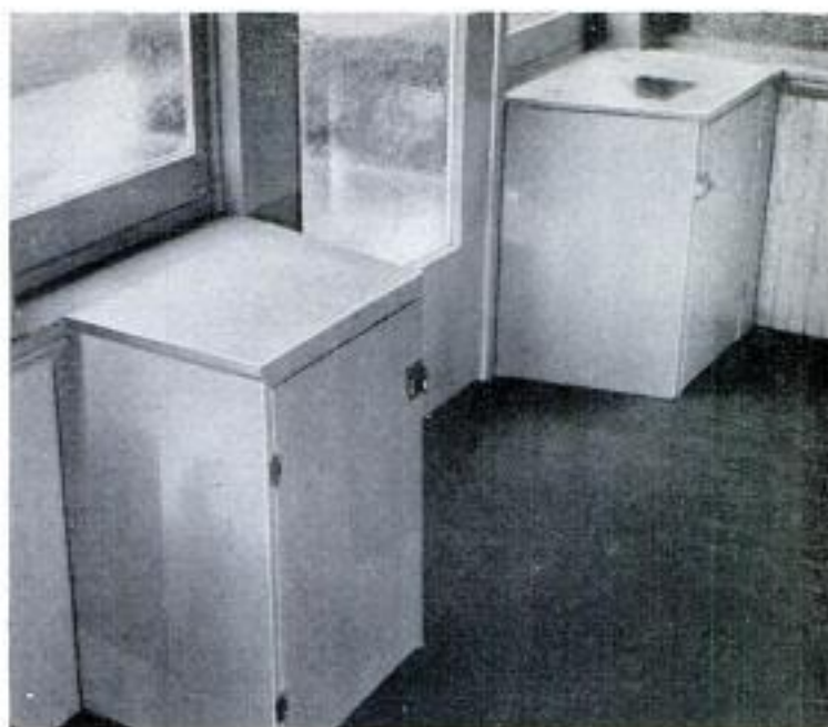
Partially finished newspaper-milk compartment is shown at left. Photo at right shows finished compartments
