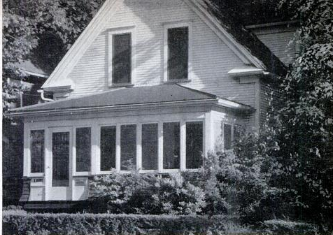
Here's how newly enclosed porch looks from the outside. Compartments flanking door make neat arrangement
