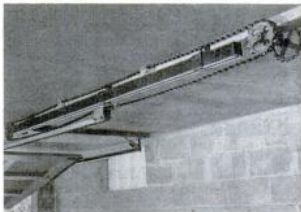
The completed lifting unit is shown here ready for installation of the power drive. Door is nearly open
