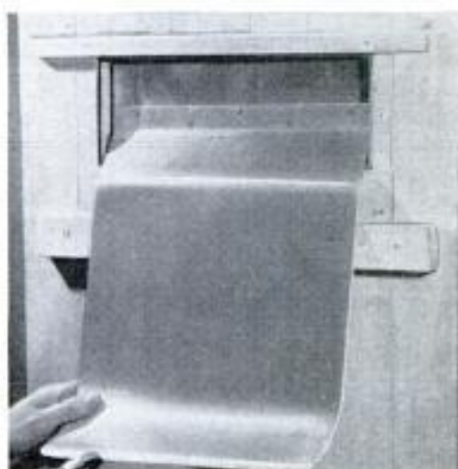
Sheet-metal mail chute is formed as above
