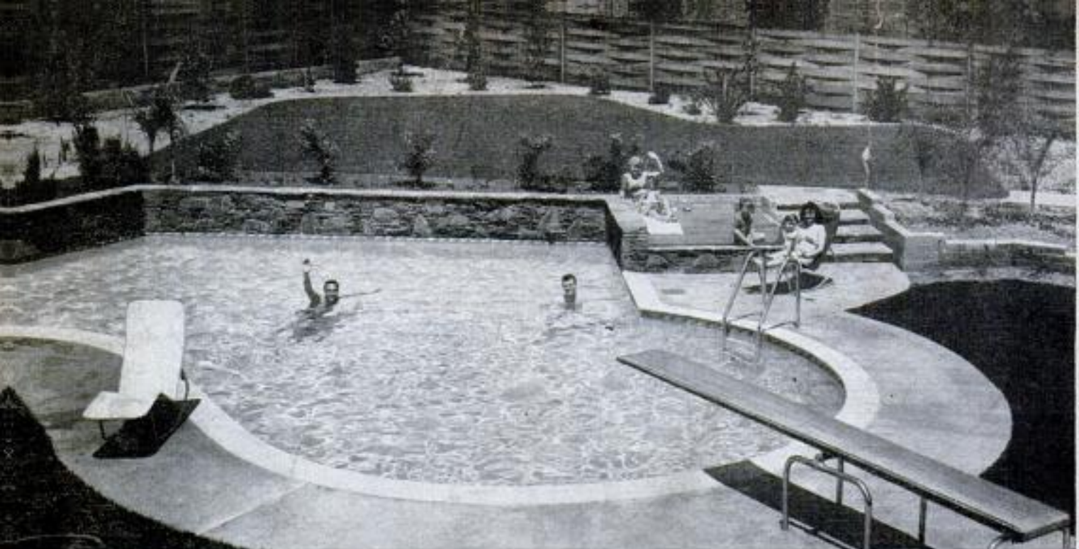
Gunite pool fits beautifully into grounds. Back wall of the pool forms a terrace at the rear of the home
