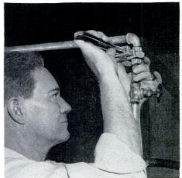
Above, a 2-wire conduit from the control panel is connected to the air conditioner at a junction box. Below, delivery water line to conditioner should have a valve to control the flow of water as desired
