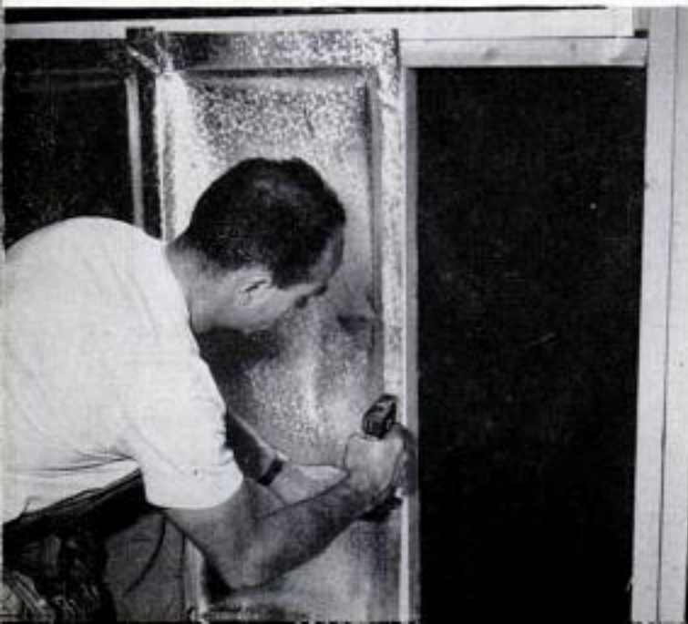
Short blocking between partition studs provides nailers for wooden wall panels. Insulation is reflective type, applied with a rented stapler, below
