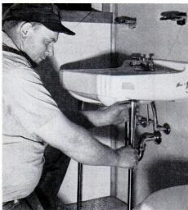
Fixtures in plumbing kit for this house are designed for amateur assembly. Kitchen sink, above, is fastened to the counter top with simple ring and clamps. Lavatory legs, below, are adjustable
