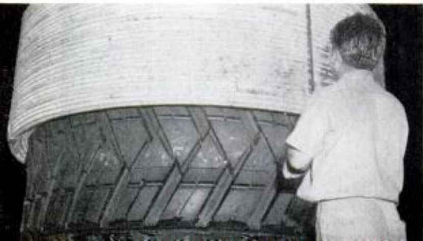
New tread is formed in a big mold, shown under man's right foot. Below, the mold is pulled upward, exposing "new" tire
