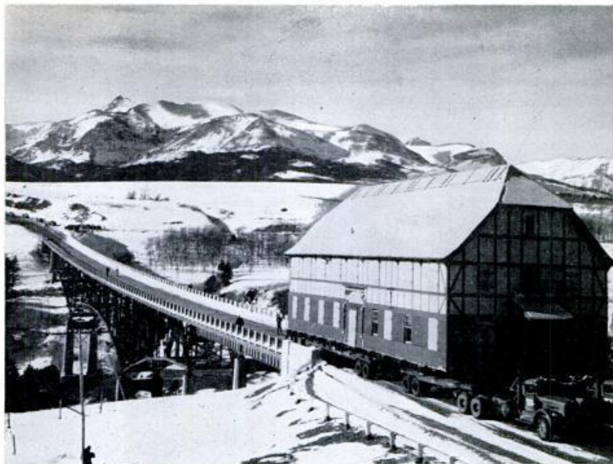
"Restless" dormitory starts across bridge. Two tractors in photo push in reverse while two others pull
