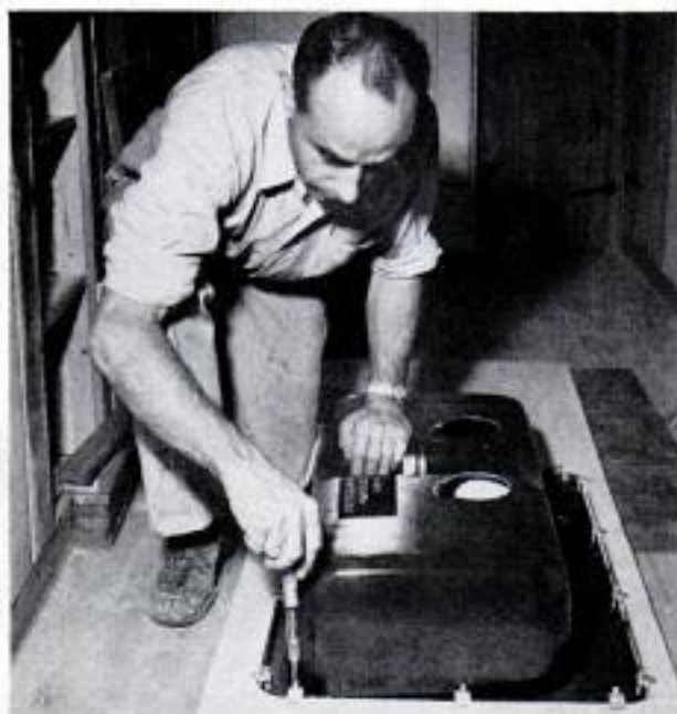
Fixtures in plumbing kit for this house are designed for amateur assembly. Kitchen sink, above, is fastened to the counter top with simple ring and clamps. Lavatory legs, below, are adjustable
