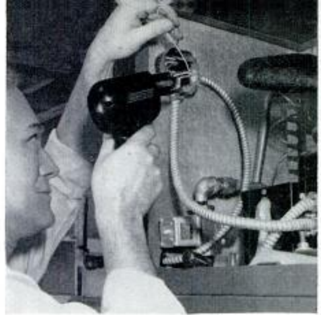
Above, a 2-wire conduit from the control panel is connected to the air conditioner at a junction box. Below, delivery water line to conditioner should have a valve to control the flow of water as desired
