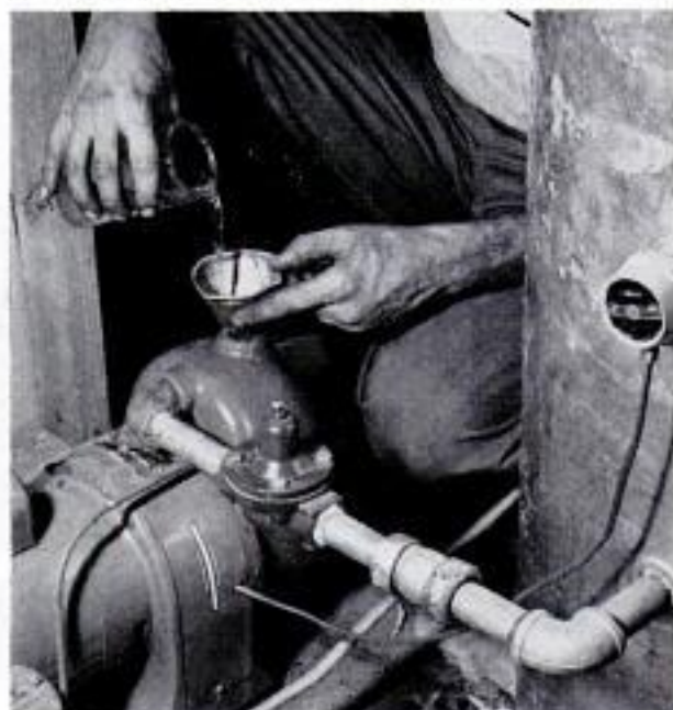
Water for the test house is pumped from private well by a Myers jet pump that is easily primed and drained for seasonal use. Below, closet and pass-through closures are Novafold sliding bamboo doors
