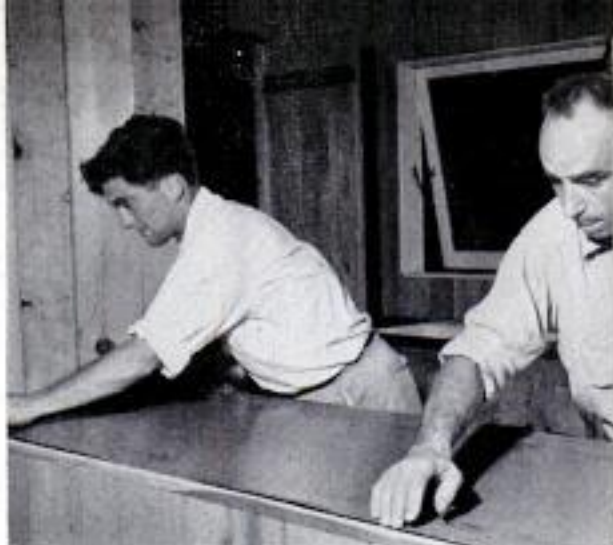
Counters are designed to make standard-size plastic top easy for amateurs to apply, like this Formica
