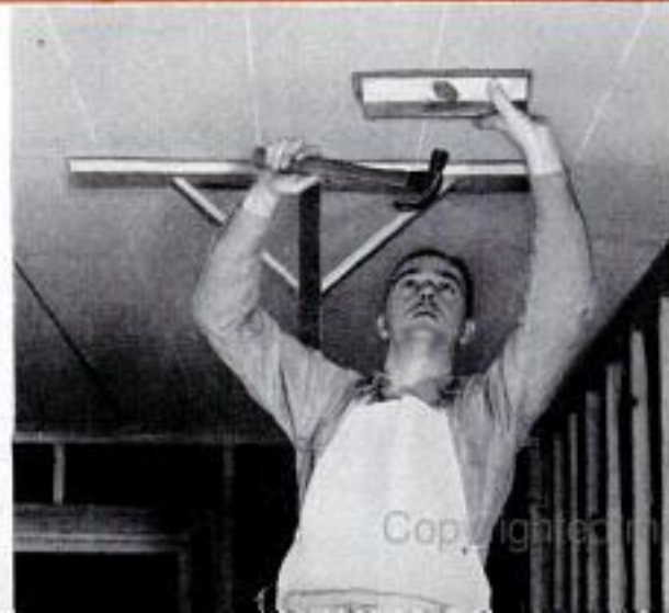
Ceiling fasteners are clinched in rear side of wallboard panels with hammer and padded block
