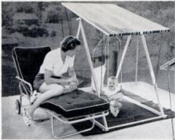
Photo above and the detail below show attachment of swing. Awning frame pivots at center. Right, standard playpen fits inside uprights
