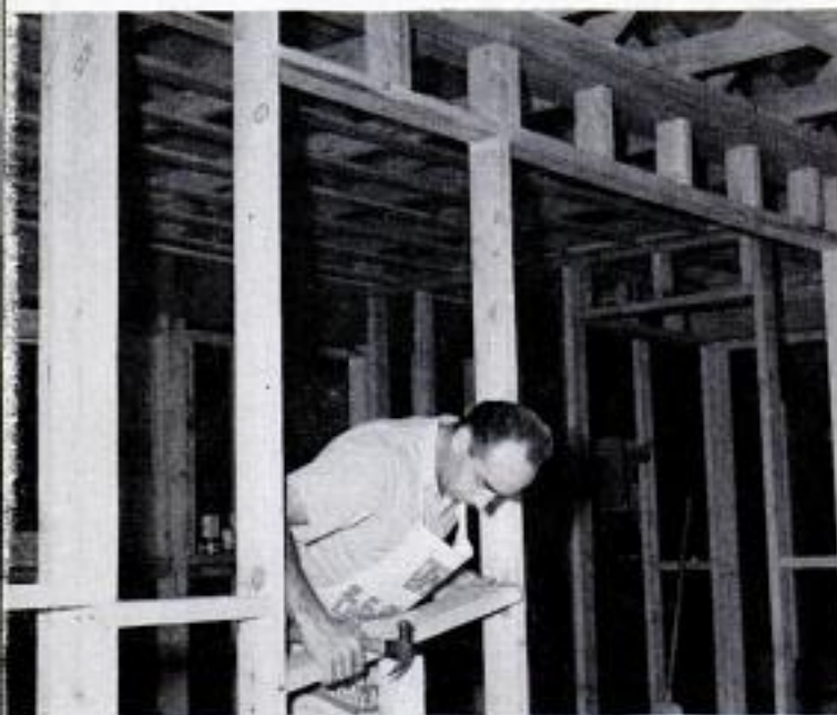
Short blocking between partition studs provides nailers for wooden wall panels. Insulation is reflective type, applied with a rented stapler, below
