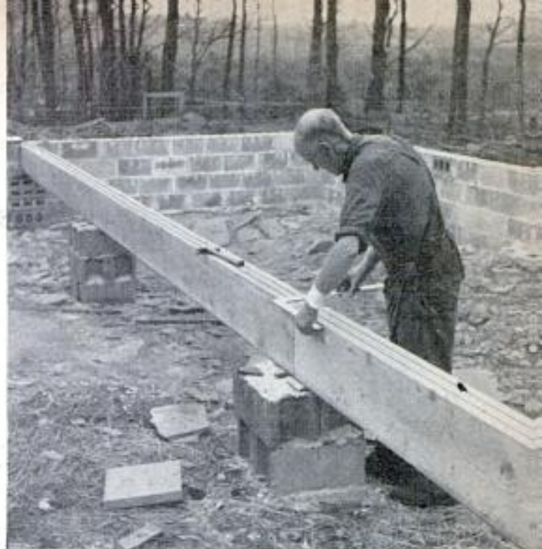
Center girder of spliced 2 x 12s rests on concrete-block piers. Joists are toenailed to sill and girder
