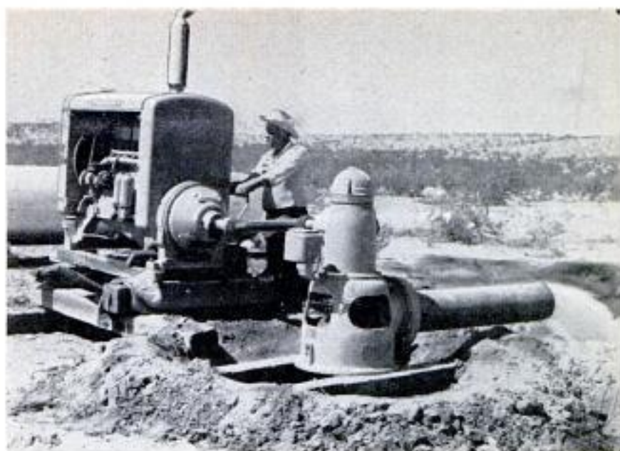
Water flows from pumping unit to fields at 2500-gallon-per-minute rate
