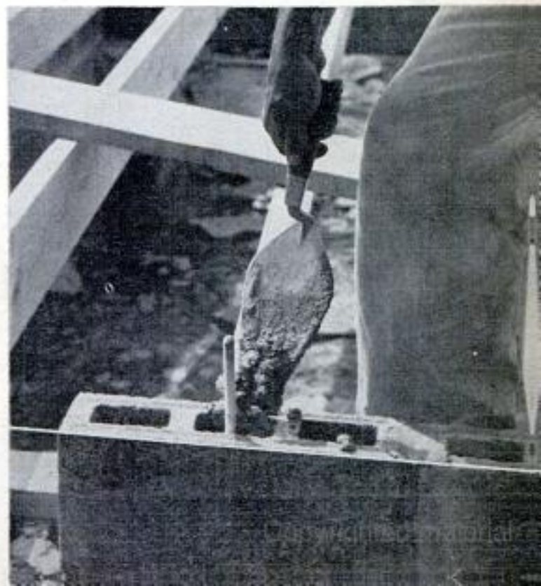
Long anchor bolts, spaced 4 to 6 ft. apart, are set in mortar when the course of 4-in. block is laid
