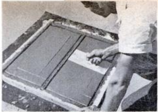
When water forms sheen on top of concrete, blocks are edged to separate them from form. Then surface of concrete is smoothed carefully with a steel trowel
