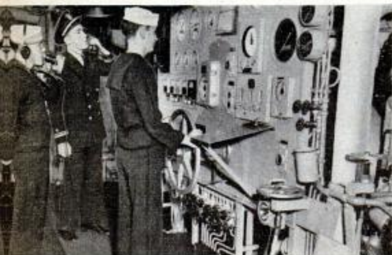
Engine room on USS Dealey has less machinery than old DEs but increased horsepower from 12,000 to 20,000. Left to right, talker, chief engineer and throttleman. Below, gun crew at enclosed 3-inch
