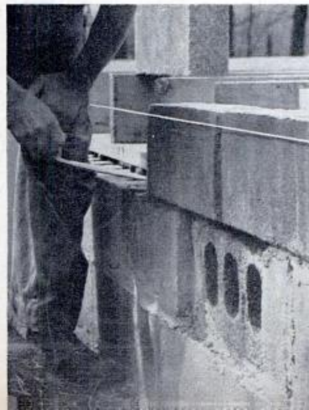
Blocks turned sideways in wall provide crawl-space vents. Recess to receive screen-covered frames
