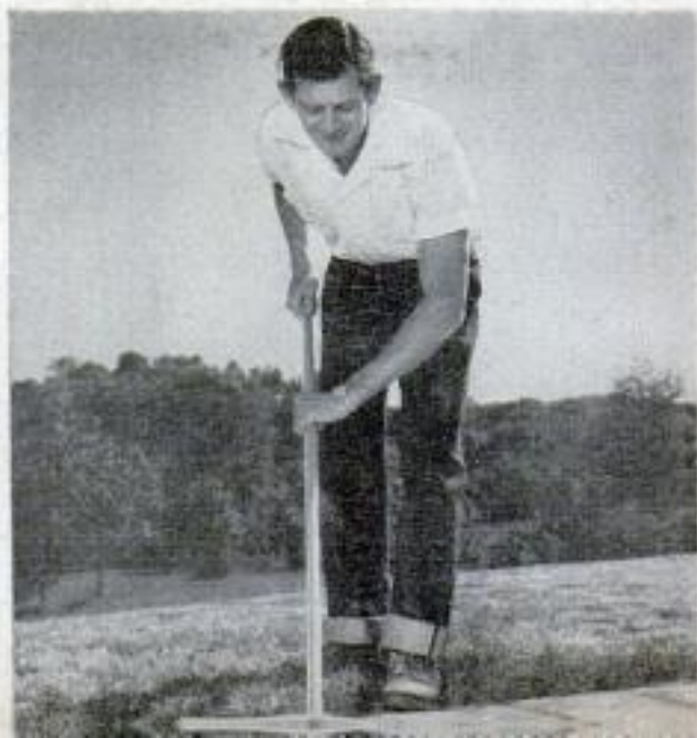
Form is removed from block by pulling apart the half-lapped corner joints with hammer as above. Finished blocks are set in walk about 2 in. apart and sand is swept into joints to prevent frost damage
