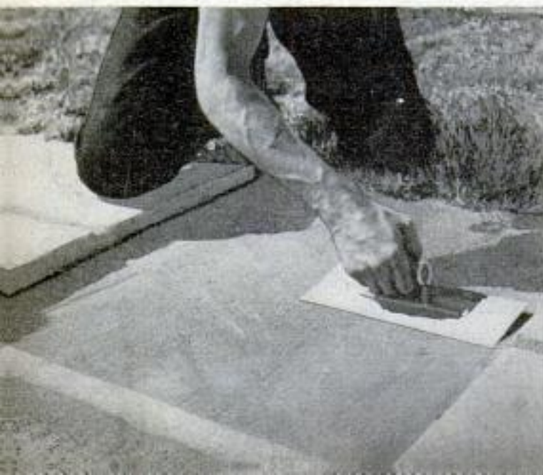
When block is cured, edges of cutouts are freed with knife blade and cutout is pulled out, leaving impression as above. Photo below shows sand, which is used for the base of the walk, being leveled with trowel
