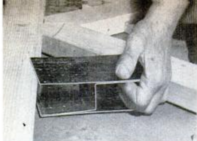
H-braces of prepunched, heavy-gauge steel make it possible to build flat truss with no lapped joints
