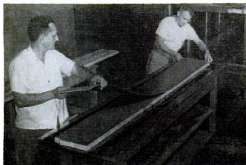
Press, below, puts uniform pressure on planks while glue cures at room temperature. Wood preservative, below right, is squirted into bolt holes to protect wood from decay in tests of stadium planking
