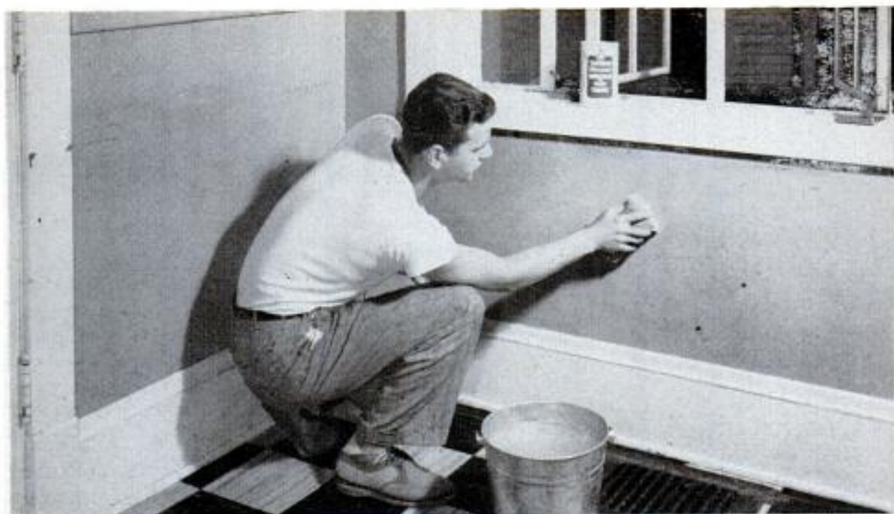
Use a sponge dipped in household cleaning solution to wash off grease and dirt. Give solution time to work, then wipe wall with clean water
