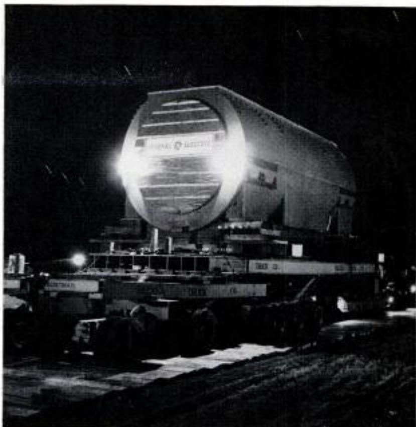
Moving the huge generator the last nine miles was a round-the-clock operation. A total of 550 planks, each 20 feet long, 12 inches wide and 3 inches thick, was used to protect the pavement from the load
