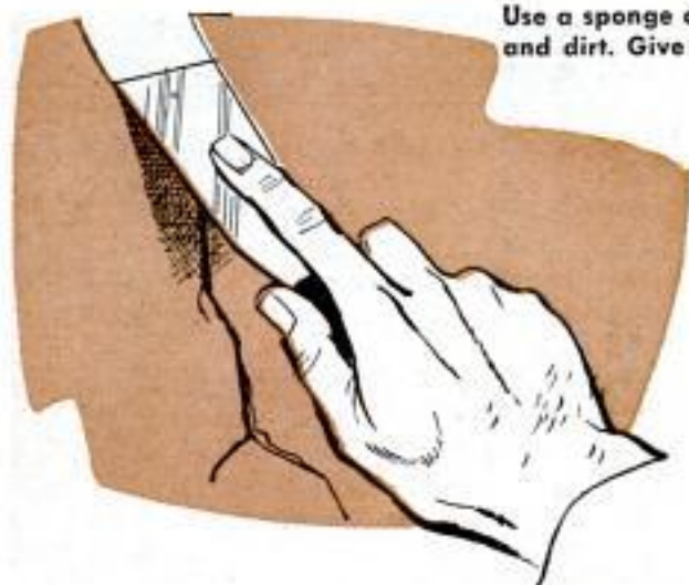
Plaster cracks should be filled before painting with Spackle. Trowel marks should later be sanded smooth
