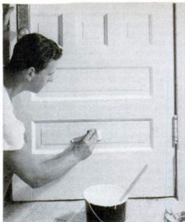
In painting paneled doors, coat the molding and panels first, then do the rest. Brush with the grain
