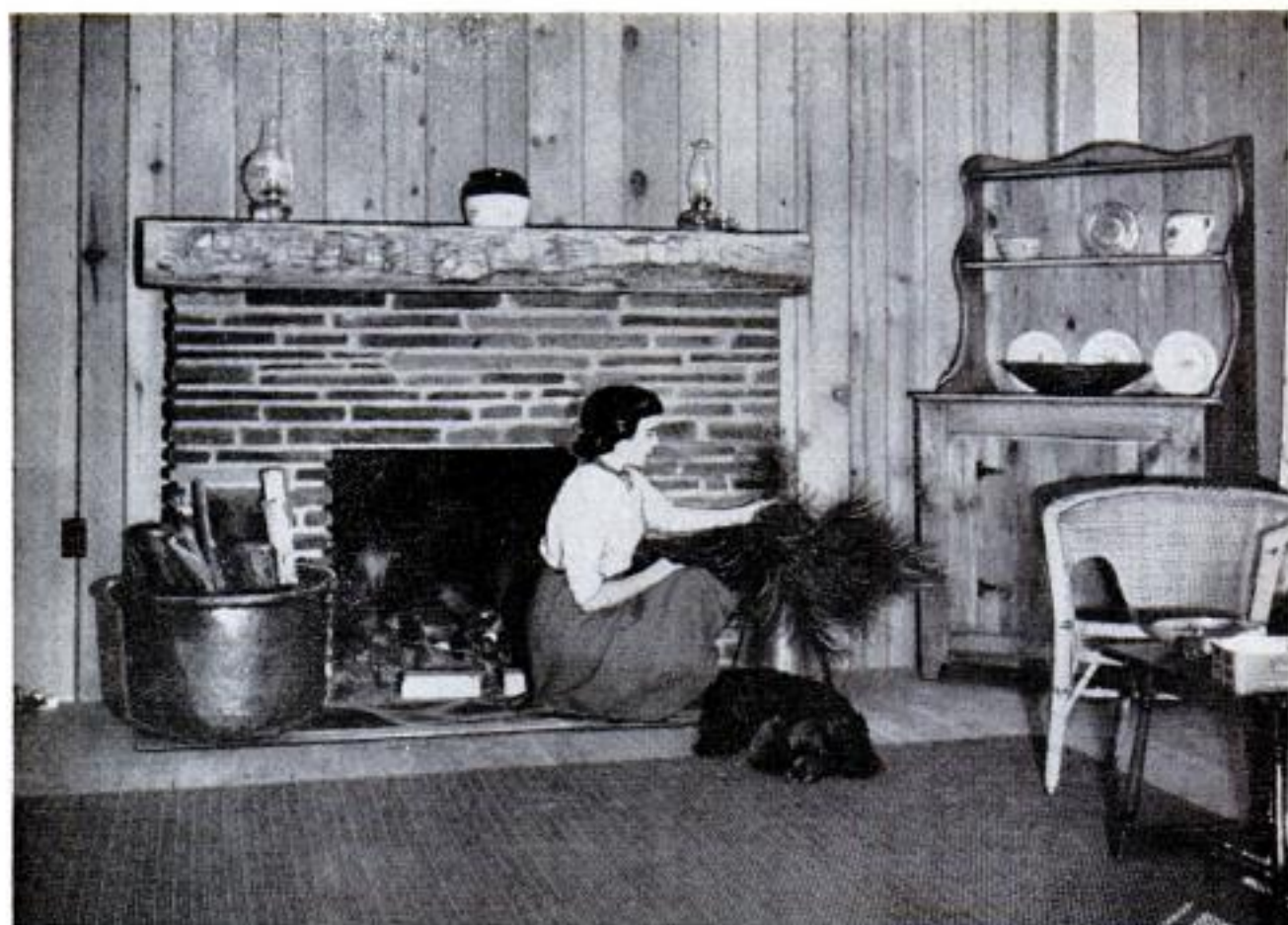
The Dempewolffs raided a stone pile to make this fireplace. Its total cost, including Heatilator, was $325
