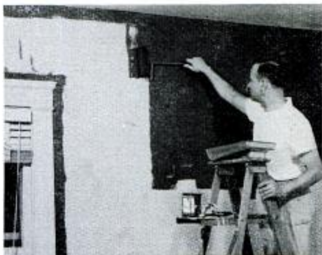
Above, ceilings are always done before the walls. Below, deep-tone colors must be applied evenly to produce a uniform coating. Here a good-quality lamb's-wool roller should be used to apply the paint. Note that a brush has been used first to cut-in around doors and windows, and along ceiling line
