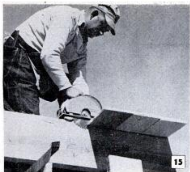
Portable electric saws are favored by many builders. They can be used with nearly all types of blades
