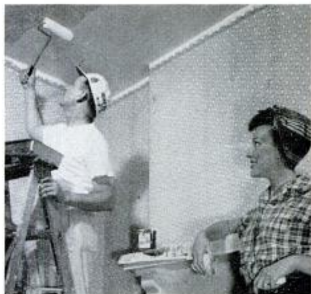
Above, ceilings are always done before the walls. Below, deep-tone colors must be applied evenly to produce a uniform coating. Here a good-quality lamb's-wool roller should be used to apply the paint. Note that a brush has been used first to cut-in around doors and windows, and along ceiling line
