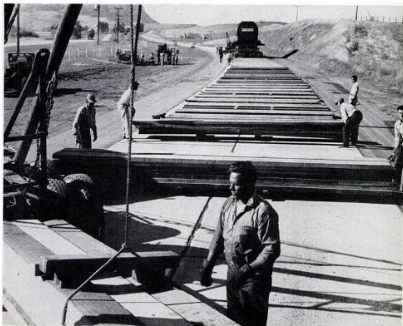
Moving the huge generator the last nine miles was a round-the-clock operation. A total of 550 planks, each 20 feet long, 12 inches wide and 3 inches thick, was used to protect the pavement from the load
