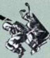
Belt, shoulder harness and leg-strap release automatically two seconds after ejection. As man leaves seat, parachute is armed
