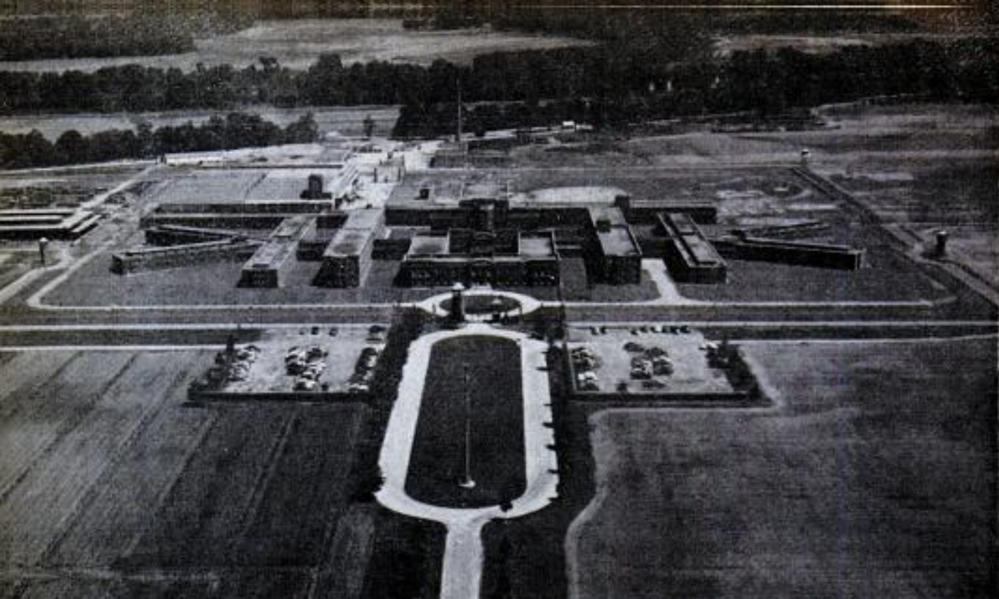
Aerial view of the Department of Justice's newest institution, the U.S. Penitentiary at Terre Haute, Ind.
