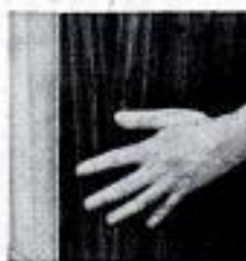
Brush Weldwood Contact Cement on studs and panel backs at points of contact. Let dry 1/2 hour and repeat. When dry, position panel; tap with hammer and wood block — job's done!
