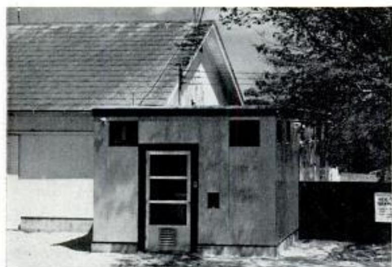
Without leaving his swivel chair in the pit, farmer can milk from 25 to 30 cows per hour. Below, the little steel building, measuring 11 by 26 feet, can be attached to an existing barn
