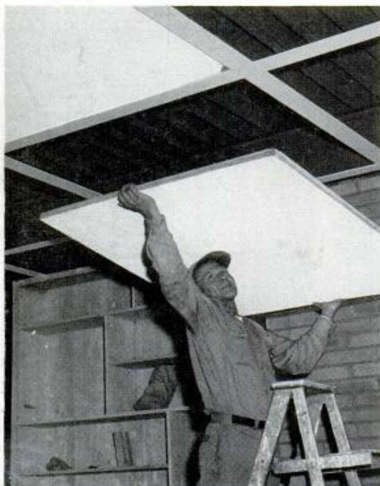
Wall panels only 1½ inches thick have insulating value of 25 inches of masonry. Below, ceiling panels rest on metal straps
