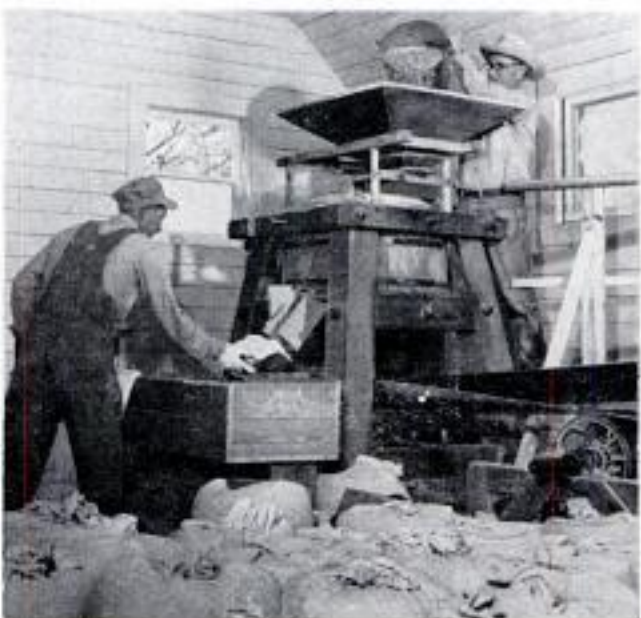
Infrared lamps around belt continue drying process Corn trickles slowly between stone grinding burrs
