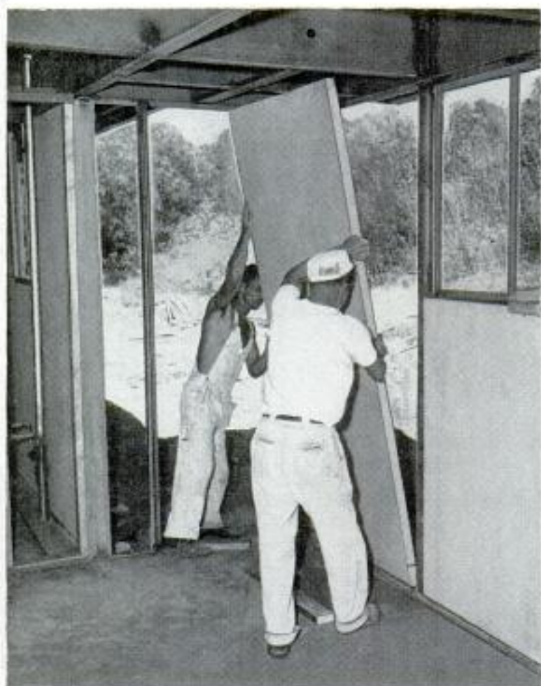
Wall panels only 1½ inches thick have insulating value of 25 inches of masonry. Below, ceiling panels rest on metal straps
