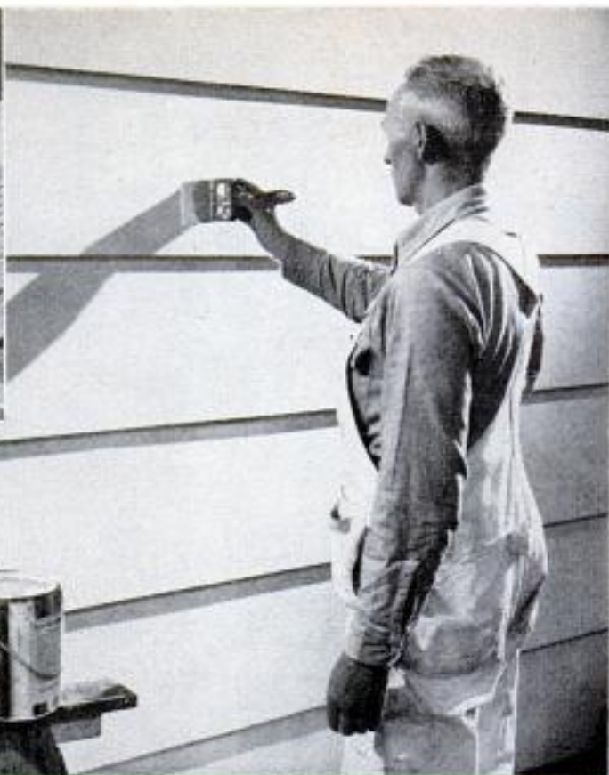
Exterior-grade fir plywood can be sealed with clear primer-sealer. A more common procedure is to use a regular grade of exterior primer thinned with 1 pt. of raw linseed oil per gallon of house paint
