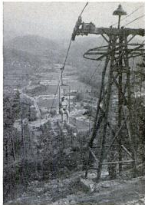
Cable anchored by five-ton weight keeps tension on pulley tower
