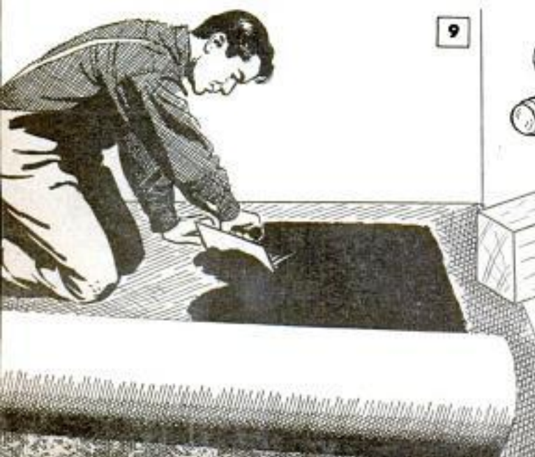
Above, when patterns are used to cut cove, allowance must be made for fitting under cap molding and corners
