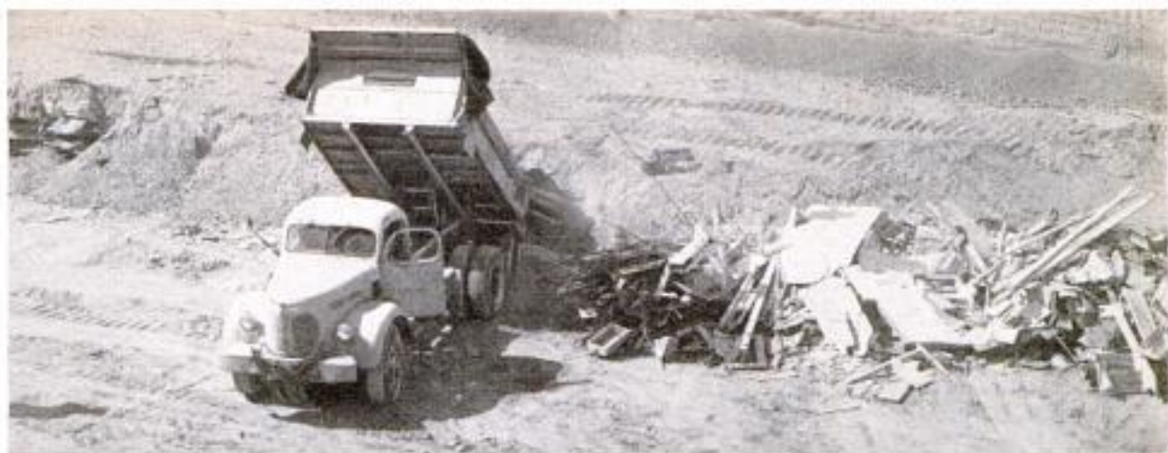
Truck dumps remains of radioactive building in 600-foot-long "grave" a safe distance from the laboratory
