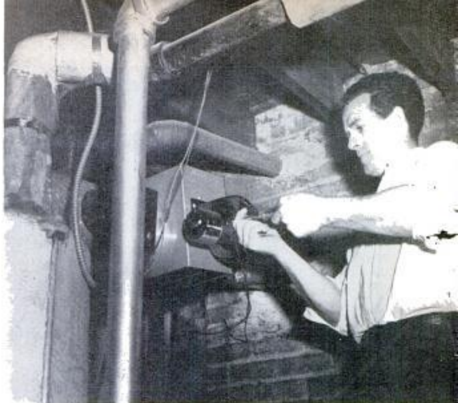
Above, the Free Heater can be installed in fairly limited space, either horizontally or vertically. Below, typical installation showing Free Heater, blower and thermostatic control for motor
