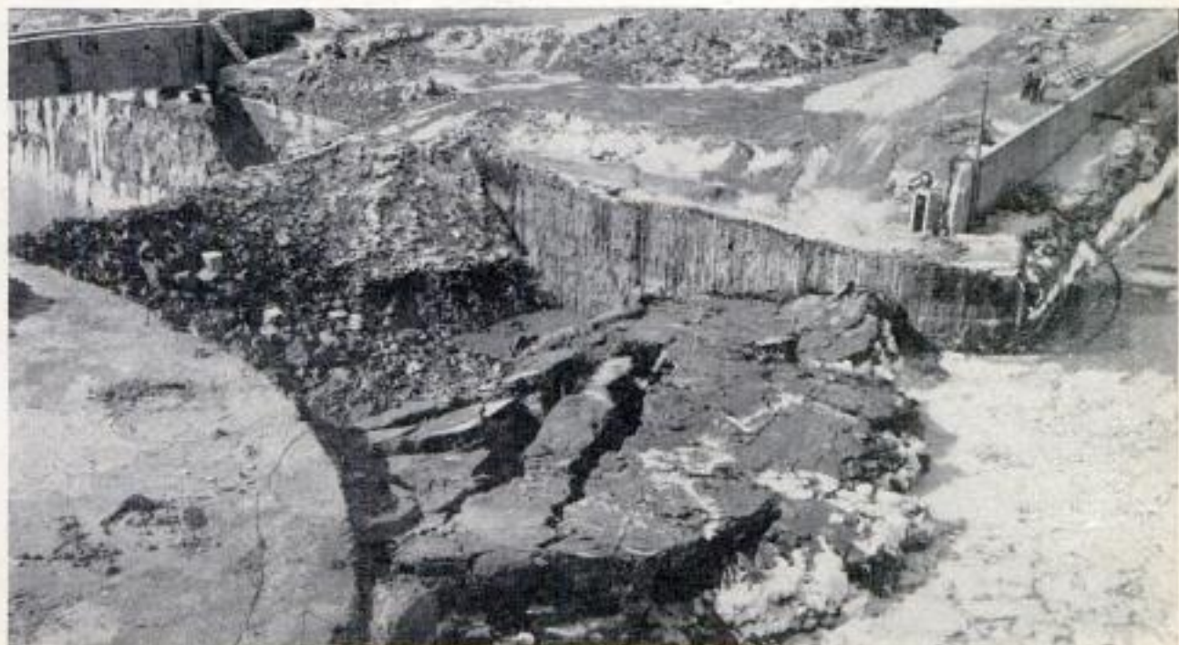
Huge wave was created by blast, but air curtain absorbed shock waves. Only a tremor was felt at powerhouse. Below, rock barrier was completely shattered by massive charge of explosives. Cost of project was $2000
