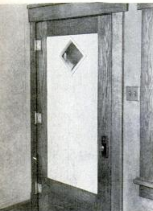
Above, assembly before refinishing. Below, door is filled, sanded, painted white
