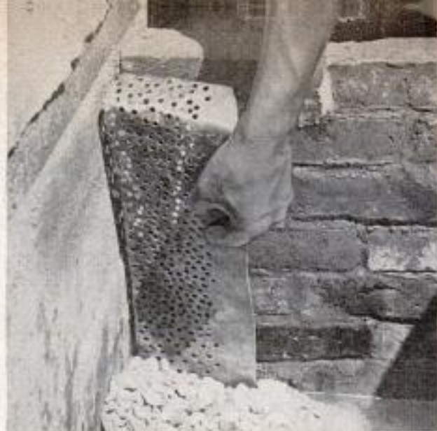
Several bricks are left out of one end of each baffle (on opposite sides of tank) so water can circulate through them. Opening to water storage compartment is covered with perforated sheet of copper
