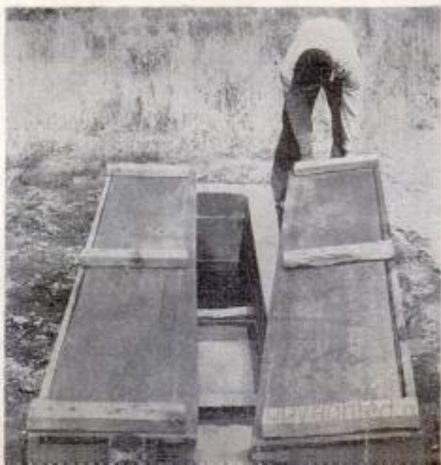
Either half of finished lid can be removed, as below, to permit access to filtering tank. Two standpipes in foreground should be covered to keep out debris, inverted coffee cans serving the purpose
