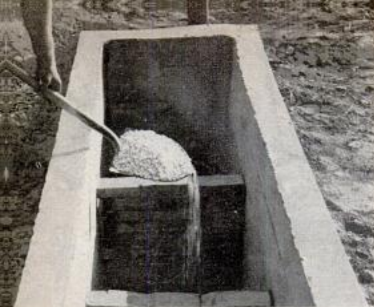
Limestone is poured into two of the three filtering-tank compartments, in this case, forming a filtering bed 33 in. deep. Limestone compartments are 30 in. long and water-storage section is 27 in. long
