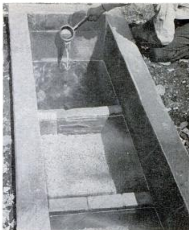
In the photo above third compartment of filtering tank contains clear water hardened by limestone
