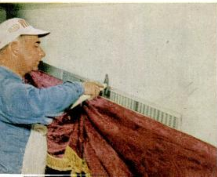
Heating and air-conditioning outlets, installed to preserve the home, are cleverly hidden behind cornices
