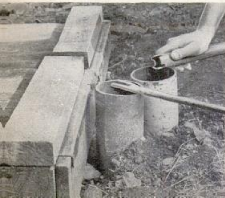
Photo below shows control rods for reaching valves used in this installation. End of lower rod engages standard handle on water-line gate valve. Upper rod is notched for wheel-type handle on bypass valve
