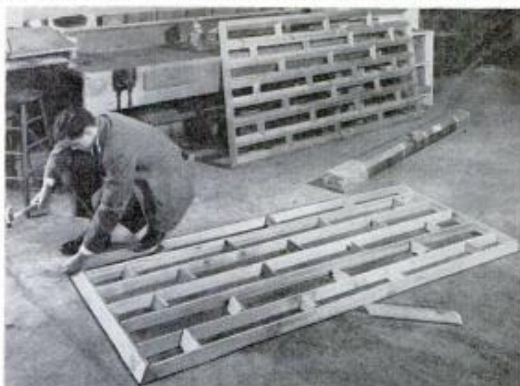
Each package of fencing contains all parts needed for an eight-foot length of fence four feet high. Below, fence installed
