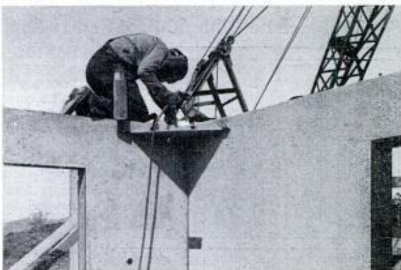
Above, workman is welding a corner joint in the upright walls. The walls are also welded to steel base plates set in the concrete pier-type foundations. Below, as roof panel is lowered by crane, two men ease it into proper position. These roof slabs are six inches thick and are welded to the walls and to each other to form a sturdy home
