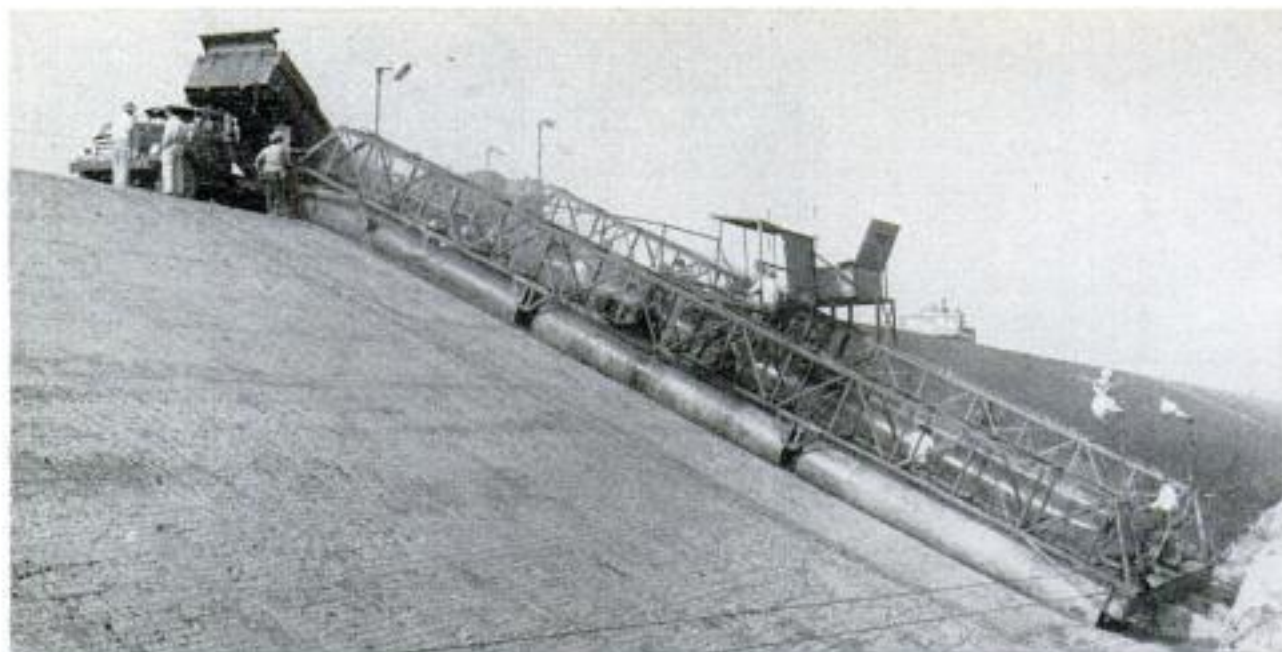
Dump truck unloads hot asphalt into side hopper of paving machine. Up to 800 tons of asphalt are laid per day
