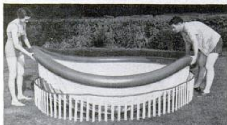
Two-foot depth allows shallow diving by small children. Air from vacuum cleaner, above, inflates liner. Installing the pool, left, requires no tools and little time. Protective bumper overhangs circular side wall of wooden stakes that upholds pool
