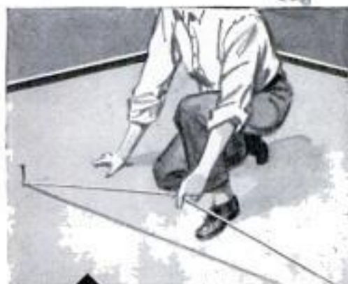
1—Mark straight lines through the center of the room in both directions, using a chalk and line.
