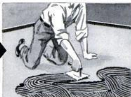
2—With a notched trowel, spread adhesive evenly over floor and allow to "set."
