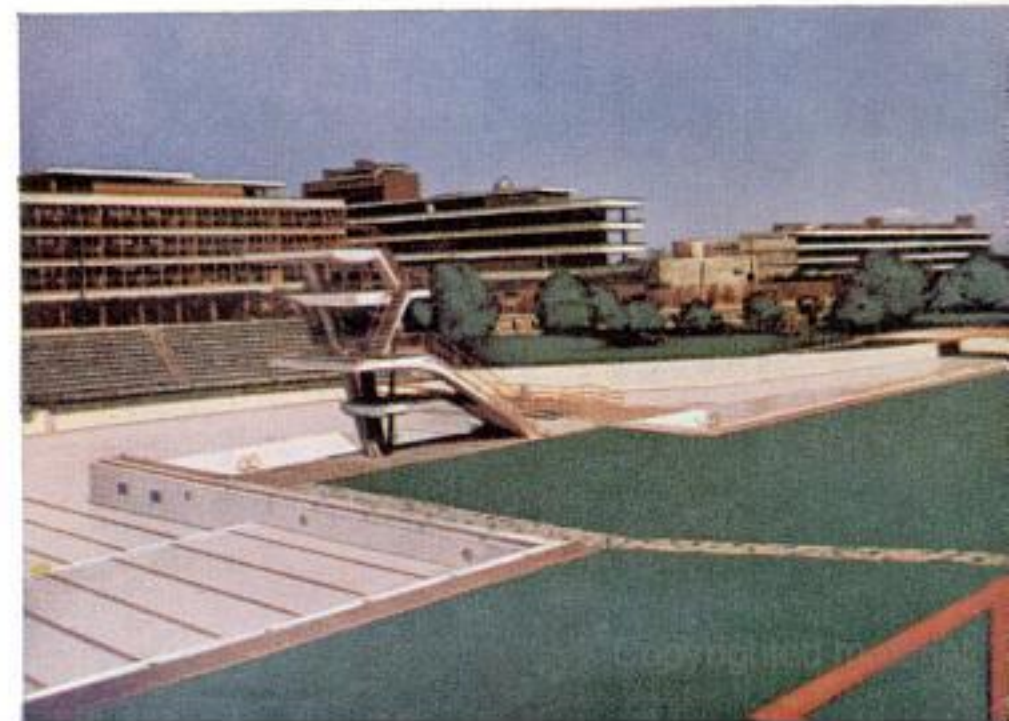
Seating areas are reached through 48 tunnels. Running track of the stadium is surfaced in black volcanic crushed rock. Below, three swimming pools are interconnected so casual swimmers can wander from one to another. Underwater windows help the coaches train their student swimmers
