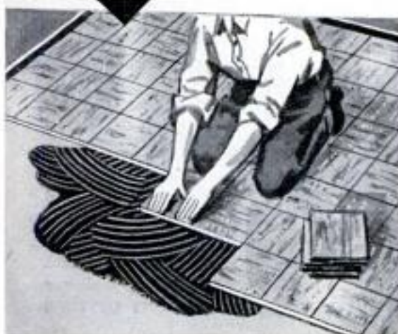
3—Press tiles into position. You can walk on MATICO as soon as floor is in place.
