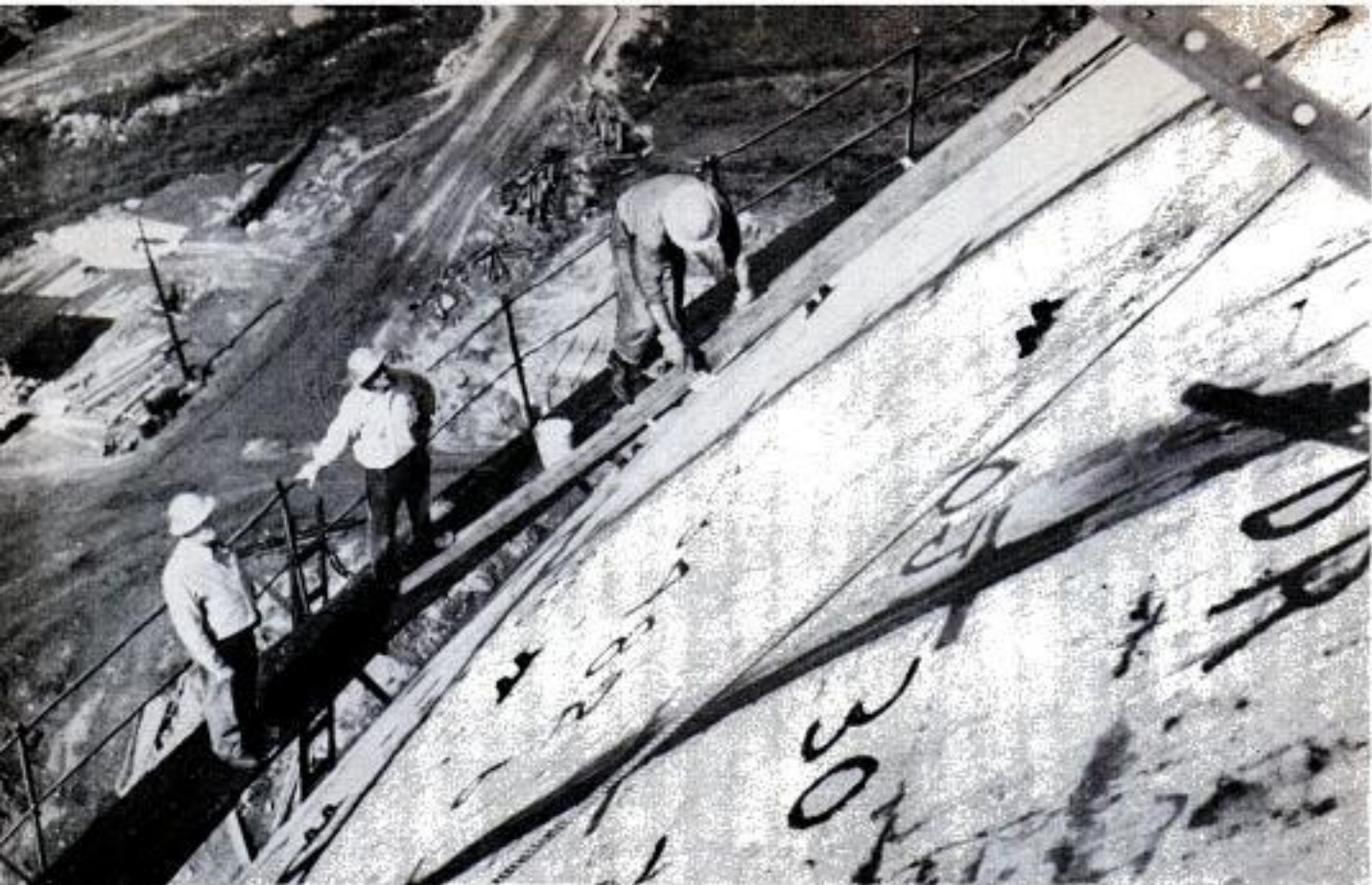
Five miles of welds on exterior of steel sphere were brushed with a soap solution to test for air leaks
