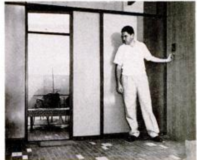
Below, remote-control panel in master bedroom. Above, sliding front door opens when key is placed in lock
