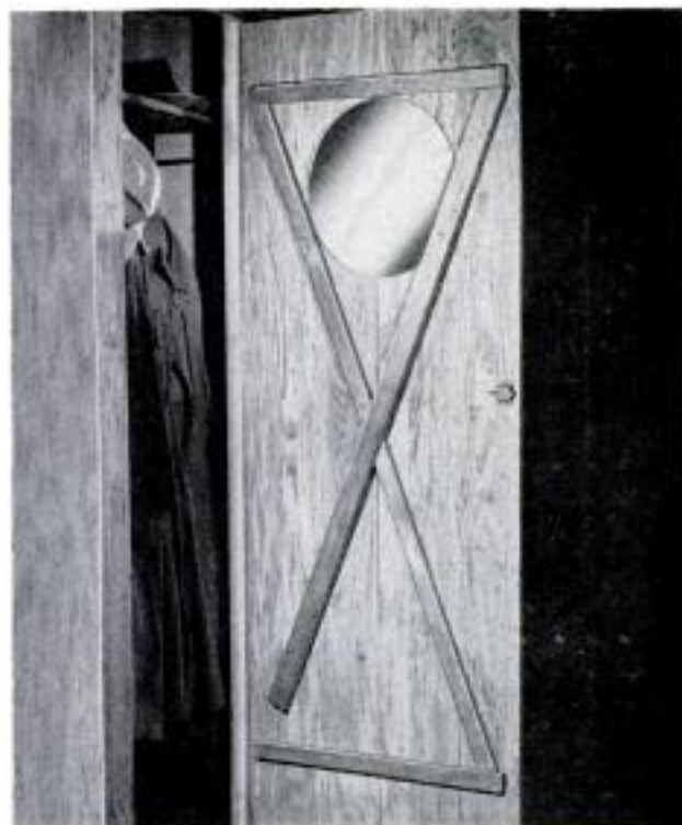
Above, crossed braces are applied to the inside of a warped closet door. Outermost brace exerts pull on top outer corner and bottom inner corner of door
