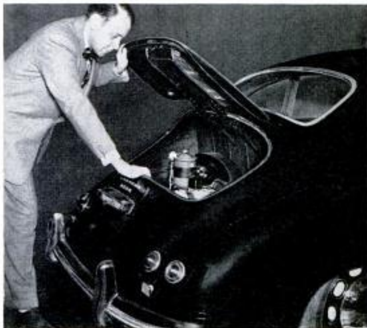
Four-cylinder, air-cooled Porsche engine fits neatly into the "trunk." It has two carburetors, gets expert factory tune up. In front is spare tire, gas tank and little luggage space
