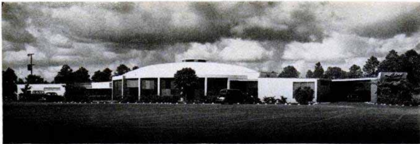
Saucer roof of theater rests on ring of steel posts around its edge. Workshops and offices are housed in wings
