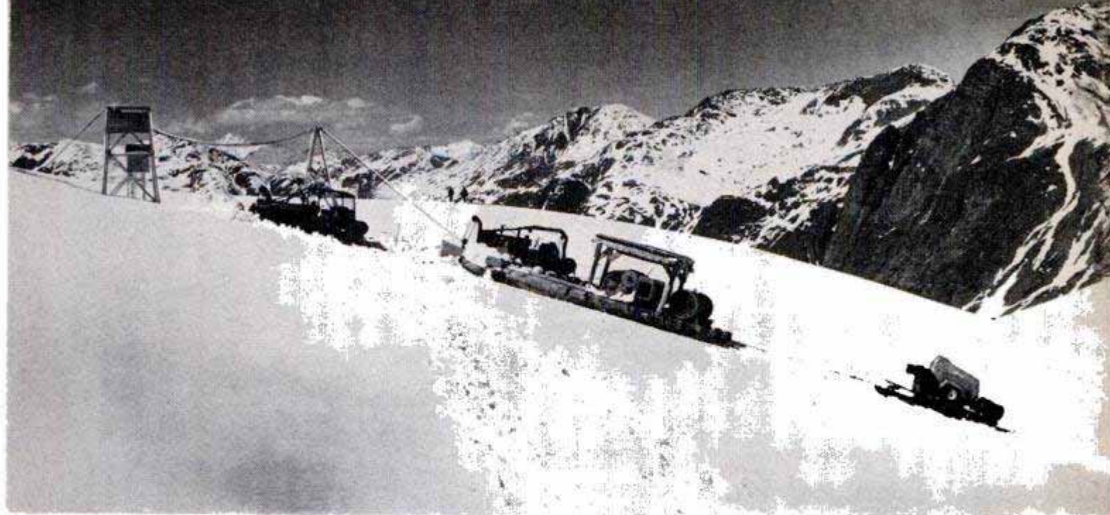
Tractors were the workhorses of the projects. Here one drags ski-mounted machinery to a 5300-foot summit
