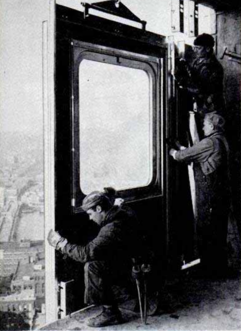
Six-by-twelve-foot exterior panels already fitted with windows are bolted to metal brackets by crew inside the building. Workmen on floor above position the panels. No taping or caulking of joints is needed
