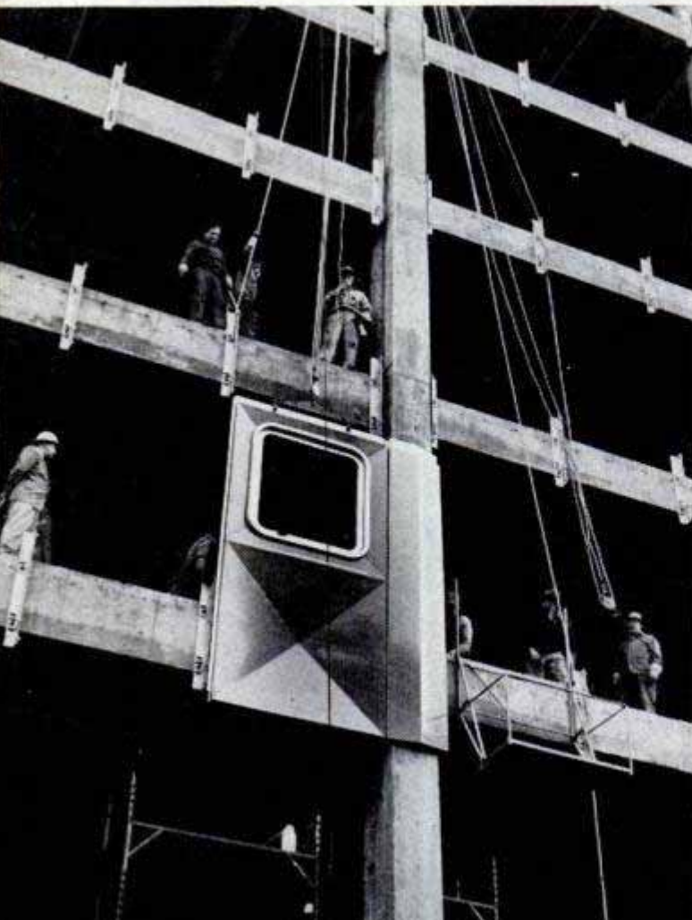
Six-by-twelve-foot exterior panels already fitted with windows are bolted to metal brackets by crew inside the building. Workmen on floor above position the panels. No taping or caulking of joints is needed
