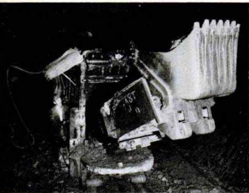
Mucker working its way through the tunnel. Below, dozing rocks inside powerhouse cavern. The exhaust "scrubber" unit shown eliminates most harmful gases
