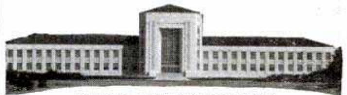
EZEKIEL W. CULLEN BUILDING
