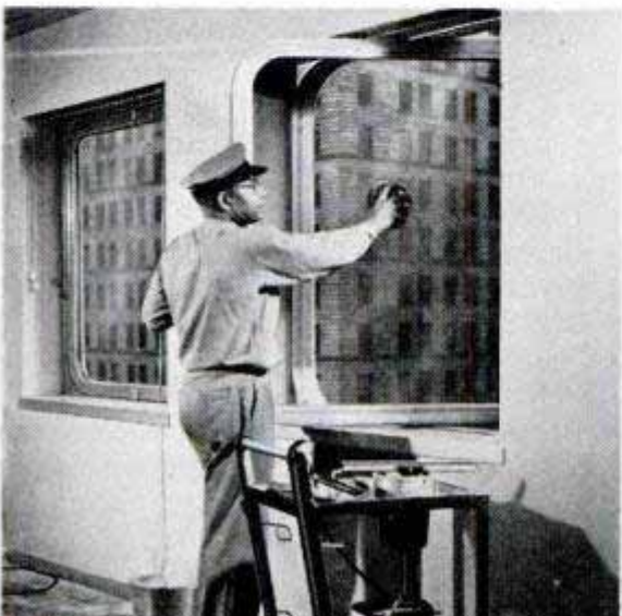
Y-shape tool deflates and inflates a rubber gasket before and after cleaning. Key at right locks window. Below, window is reversed for washing. Compressor on cart supplies air hose
