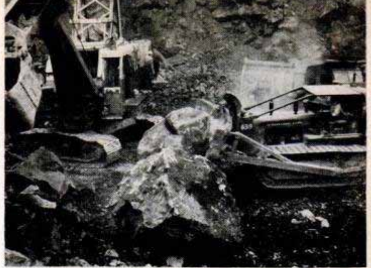
After being positioned for the shovels by TD-24s, the huge rocks were dumped into big Euclid trucks like the one in the background and scooted away to the quarry
