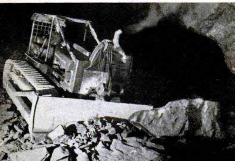
Mucker working its way through the tunnel. Below, dozing rocks inside powerhouse cavern. The exhaust "scrubber" unit shown eliminates most harmful gases
