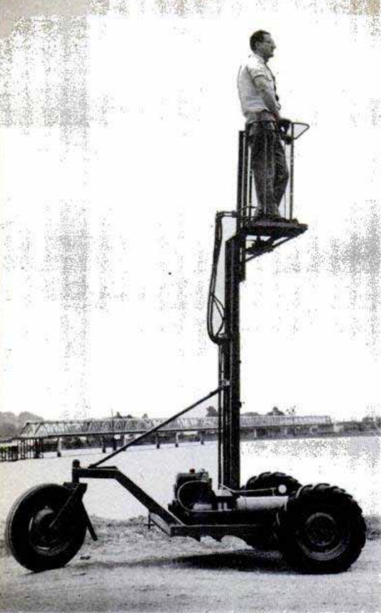
"Steel squirrel" is a self-propelled perch for orchard workers. Below, it's small enough to move easily between trees. Operator guides it by foot and hand controls, has compressed air at hand for pneumatic tools
