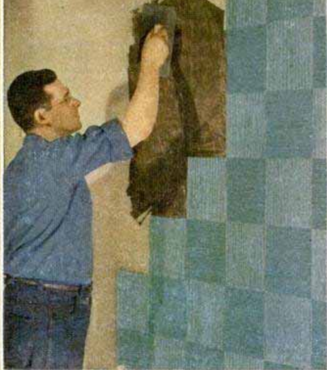
Placing ribbed texture of "bamboo" tile at right angles to each other produces pleasing basket-weave effect. Irregularities in tile joints are concealed with special colored filler
