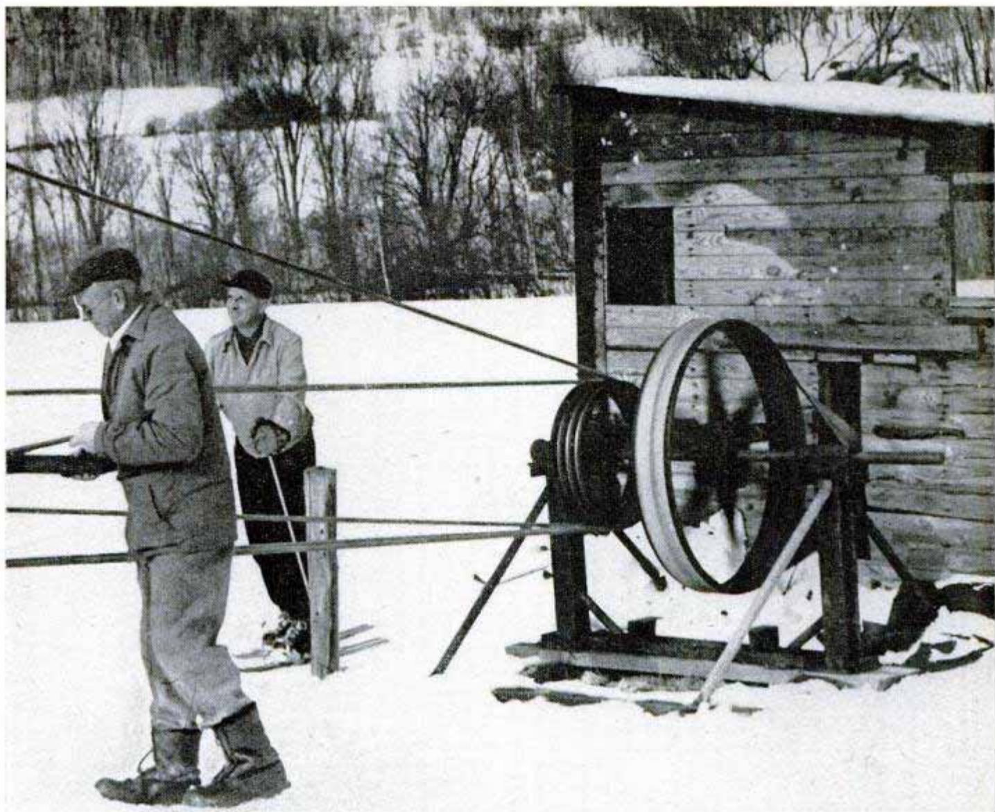
Enterprising farmer oils idler pulley while two skiers await a fast trip to the top of the ski slope. ↓ Operating captive tractor, Greene watches through window of old chicken house as skier traffic moves uphill
