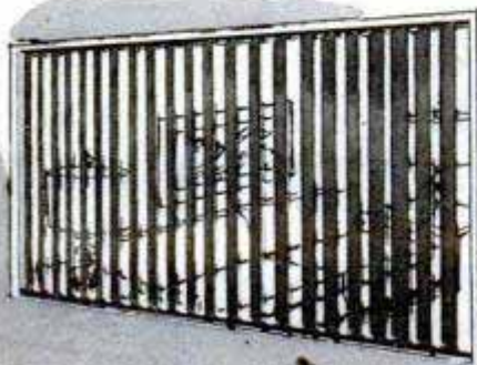
When a partition cuts off light—often a problem in older homes—defect can be corrected by installing a vertical jalousie unit that opens and closes
