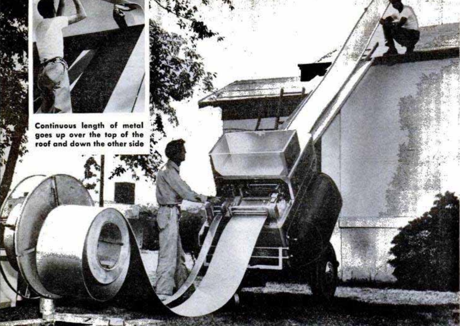
Rolls of sheet aluminum feed machine, which turns them into battens and roofing panels cut to desired size
