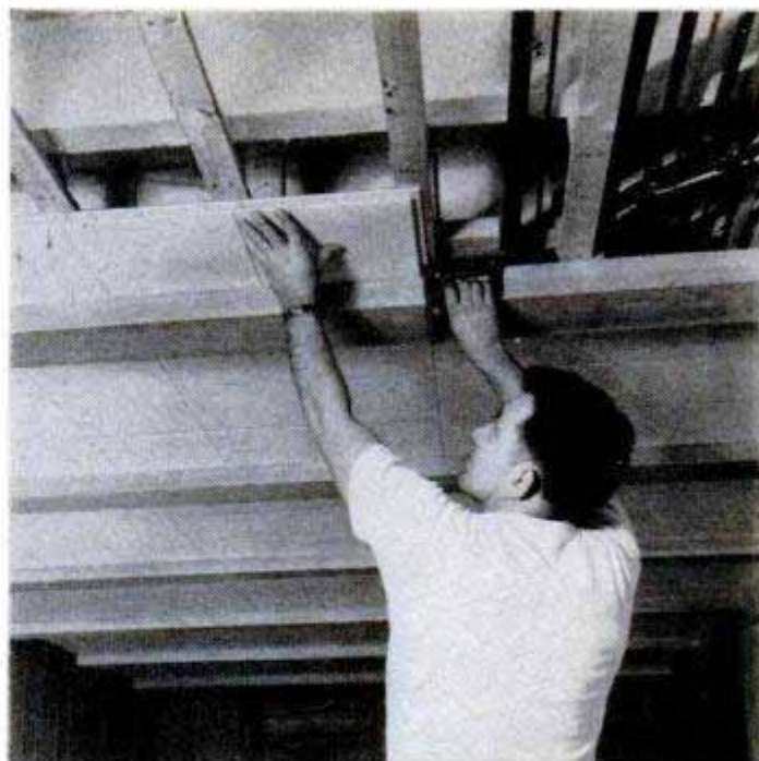
"Lok-Bevel" joint on Temlok Tile speeds application
