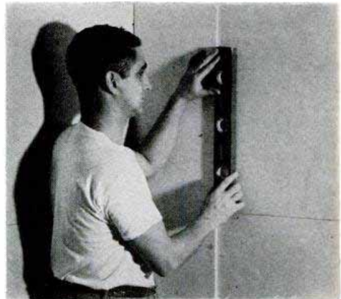
Above, place the first panel at a corner and plumb it with a carpenter's level. Press board lightly against surface to assure even adhesion. Below, succeeding panels are kept snug by tapping with 2 x 4
