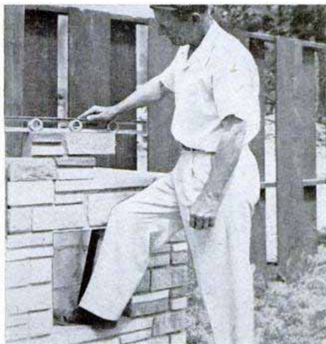
Mold has surface texture of real stone. Right, ends of each section are lapped, making them easy to lay
