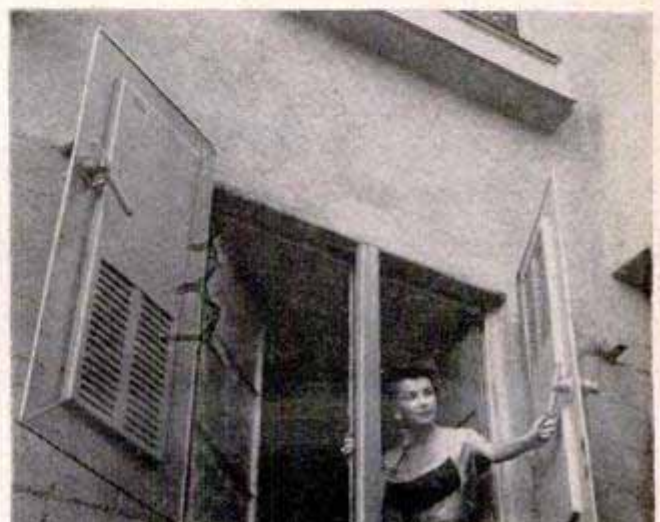
Bomb shelter in the house itself has strong steel shutters which can be closed in case of air attack
