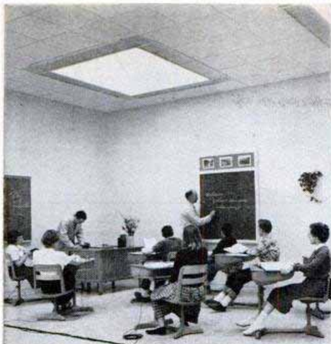
Skylight distributes light evenly throughout room, provides proper illumination on cloudy or sunny days
