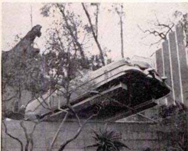
Car is parked on cantilevered steel tracks which overhang cliff below house. Space is at a premium
