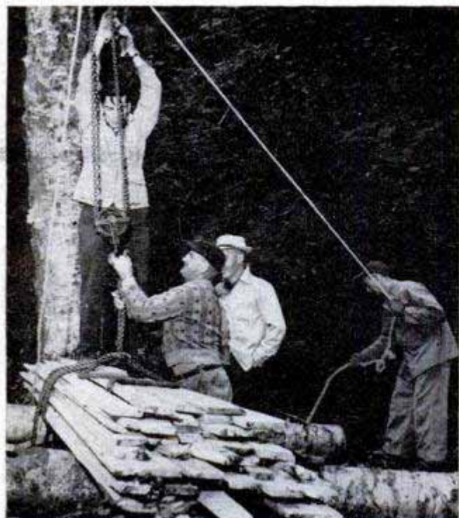
At anchor tree, lumber is bundled and attached to carrier which takes it for “ski tow” ride up the hill
