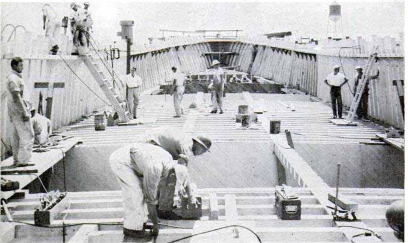
Preassembled transom is fitted to stern. Below, construction scene inside hull as wooden mine sweeper moves to completion
