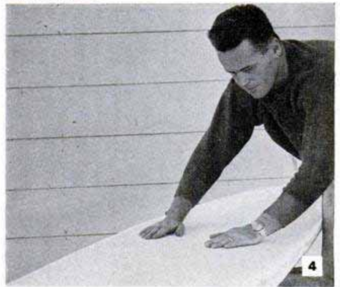
After applying sealer, spread muslin and impregnate with sealer. Apply to one side only and allow to dry before applying sealer and fabric to opposite side
