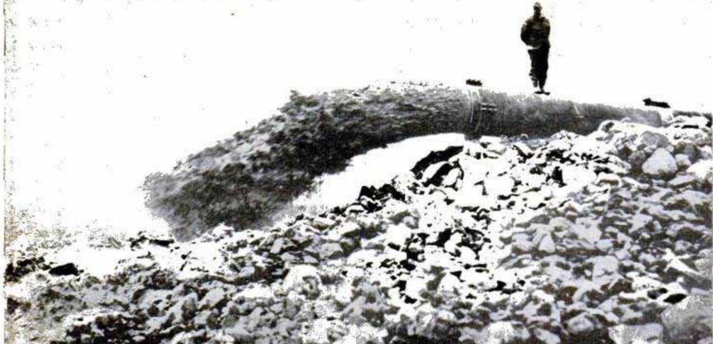
Boulders, clay, water can be carried over a mile in this dredge's discharge line, which is 36 inches in diameter
