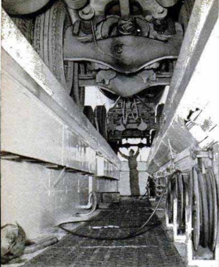
Left, truck and trailer are lubricated in 30 minutes. Right, tire repairing is done by full-time specialists
