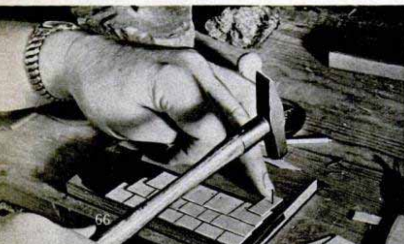
Postage-stamp-size shakes, split with a razorlike tool, are carefully nailed to a small wall section
