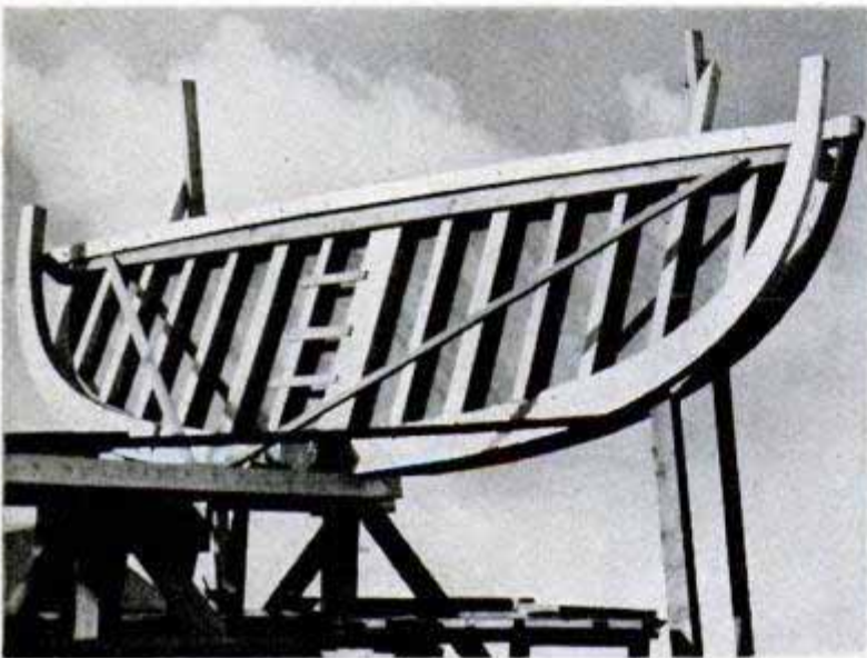
Preassembled transom is fitted to stern. Below, construction scene inside hull as wooden mine sweeper moves to completion
