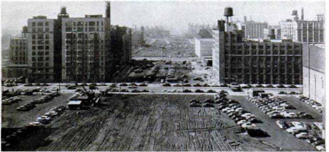
To make room for the highway, a swath one block wide was cut for eight miles through heart of the city. Huge clover leaf will siphon off Loop traffic. Motorists will drive through center of post-office building
