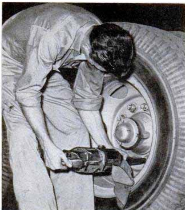
Lug nuts are quickly removed with pneumatic wrench
