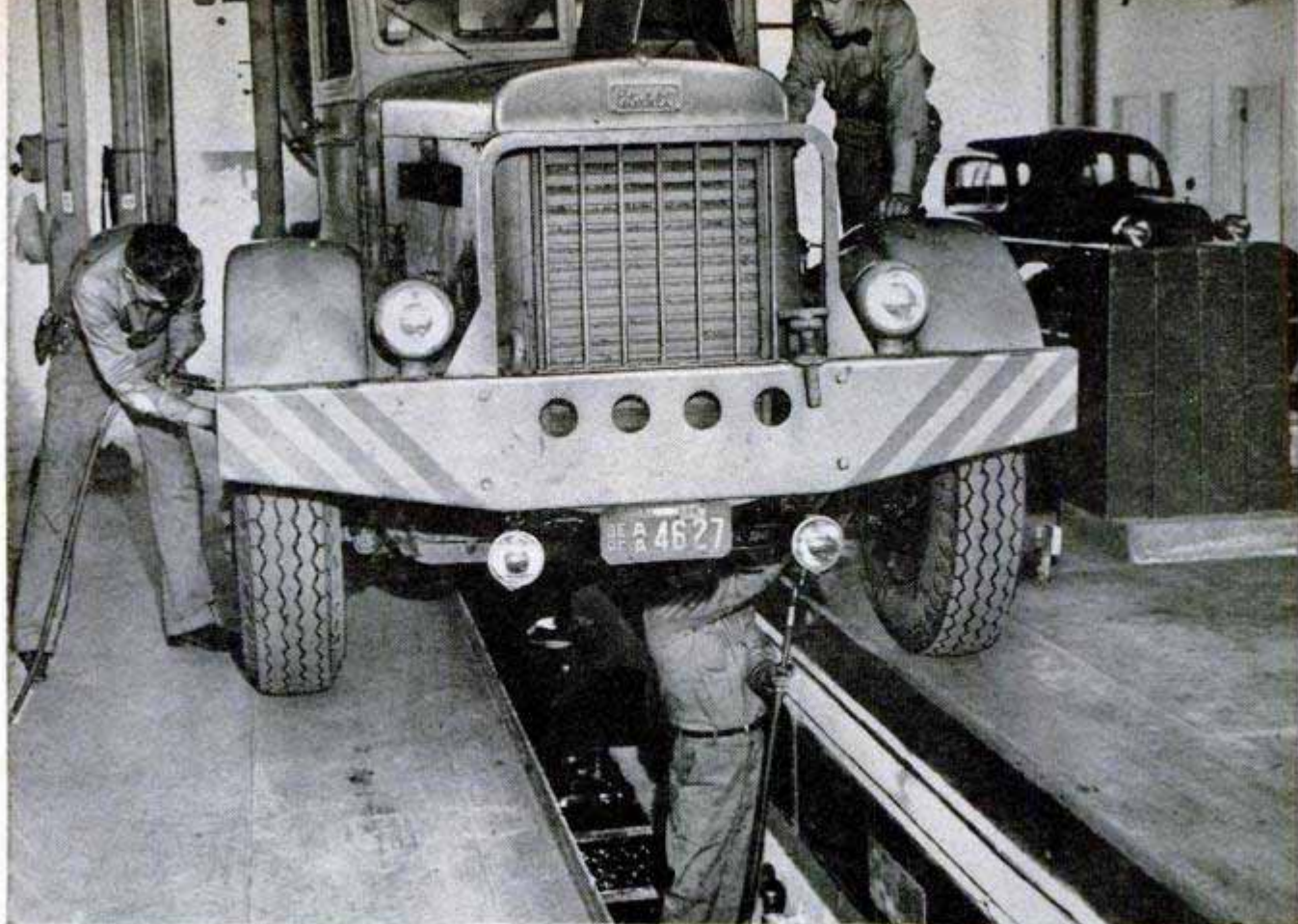
Lubrication is done without delay on 70-foot-long pits which, like the fuel pumps, are open 24 hours a day
