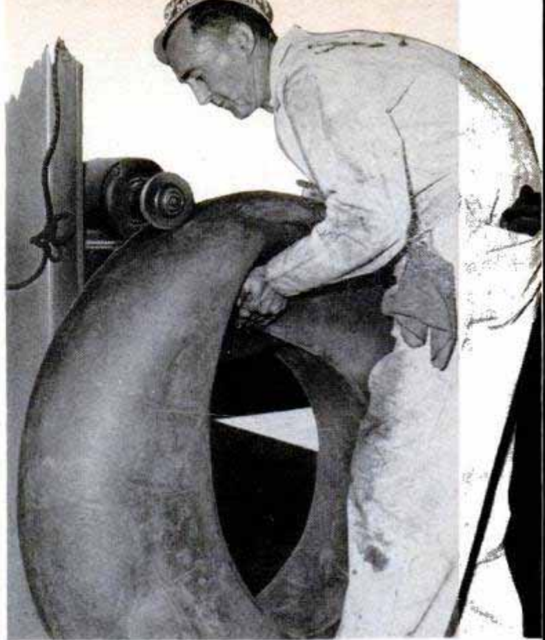
Left, truck and trailer are lubricated in 30 minutes. Right, tire repairing is done by full-time specialists
