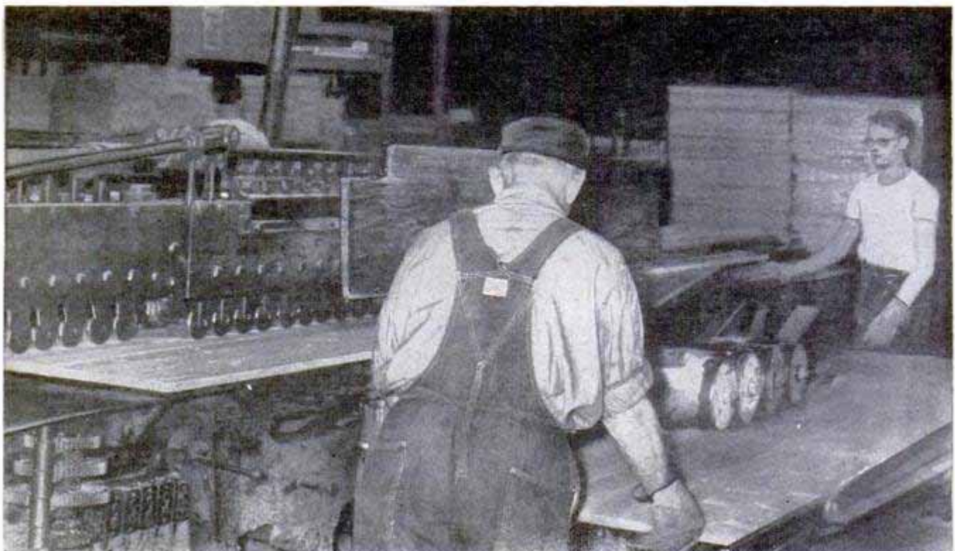
Unique machine cuts dovetail joints in edges of slats, then glues and joins them to make a panel of wood
