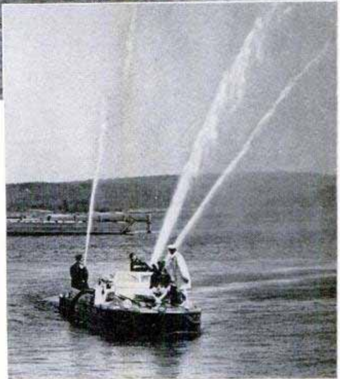
"Duck" takes to the water for a test run. Three hoses can throw hundreds of gallons per minute on a fire
