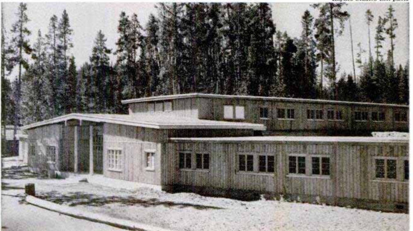
Factory-made dormitory is built from the straight logs tongued and grooved and set vertically on a foundation Haynes Studios Inc. photo
