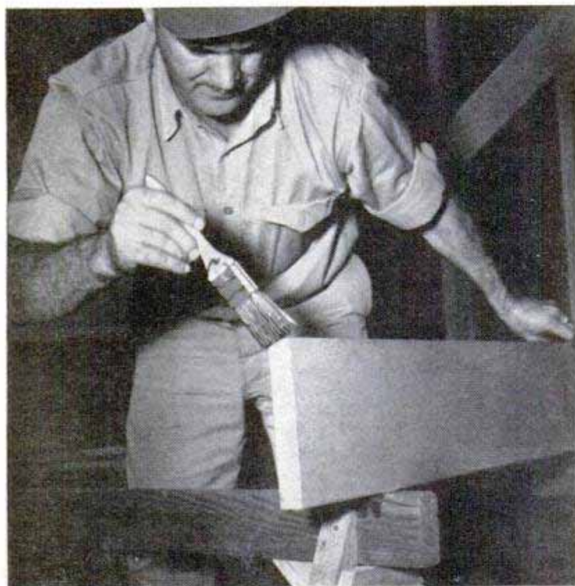
Below, sawed ends of treated lumber are re-treated to protect exposed end grain
