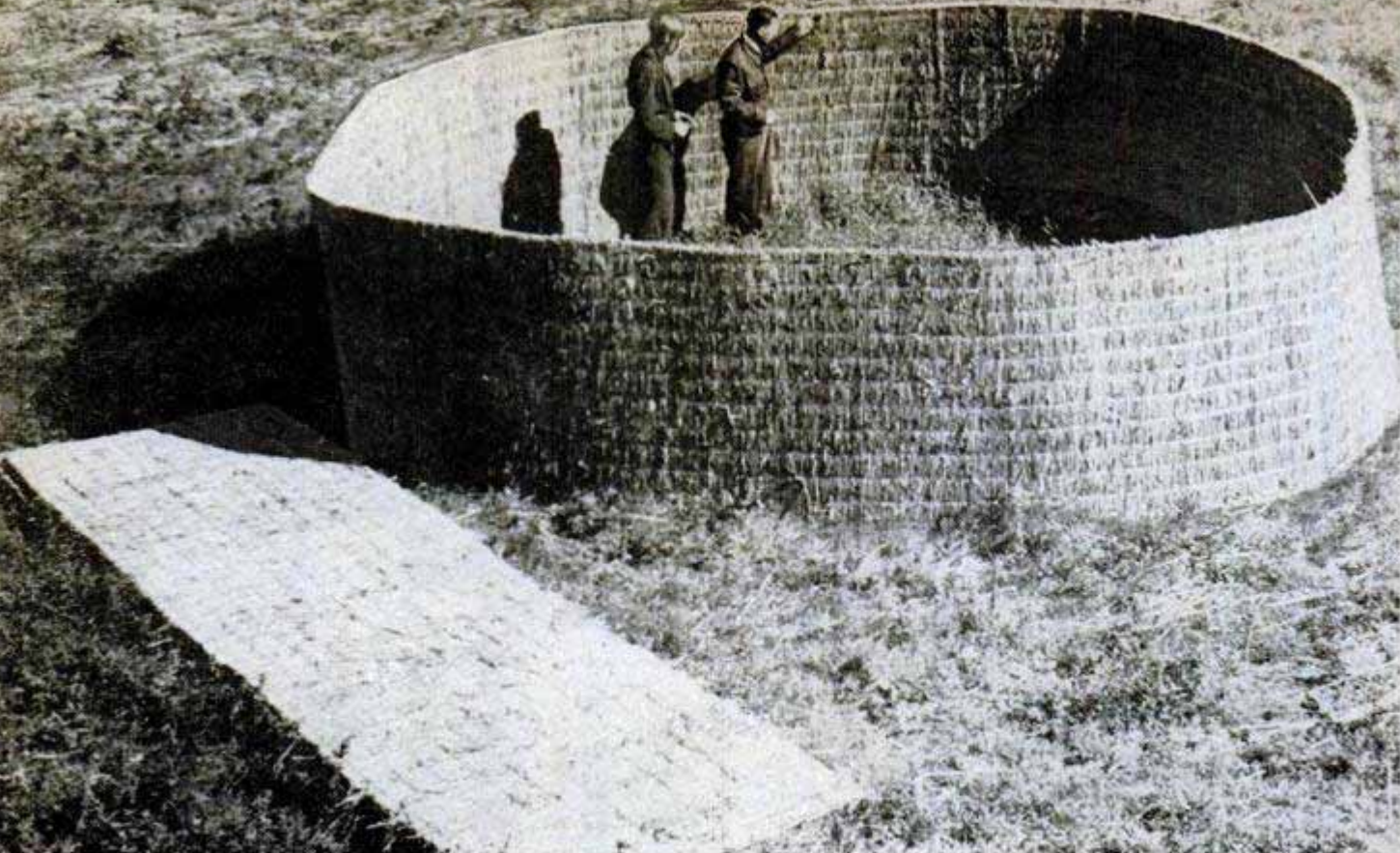
Paneling can be of any desired length. This 64-foot section forms the entire wall of a field granary
