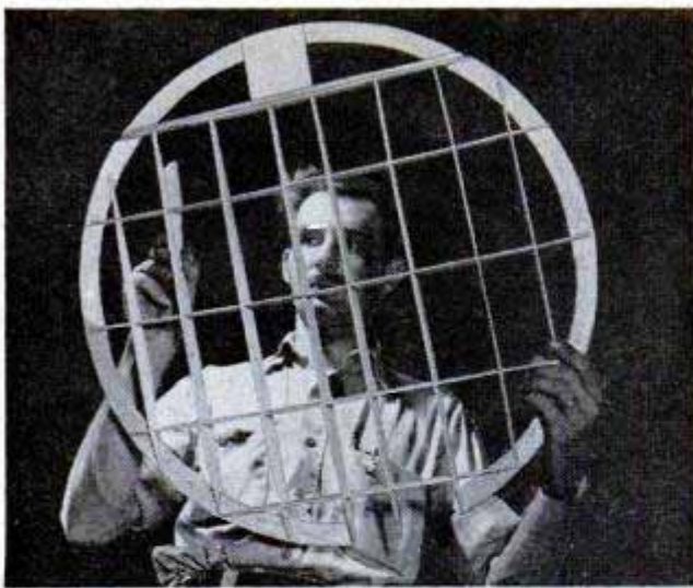
Inventor Wood shows the egg-crate-type framework of newest flying disk which is made of balsa wood
