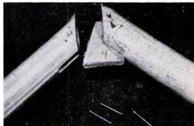
Ends of coffee-table legs are bolted to the lower sections of the table-top frame, as pictured below
