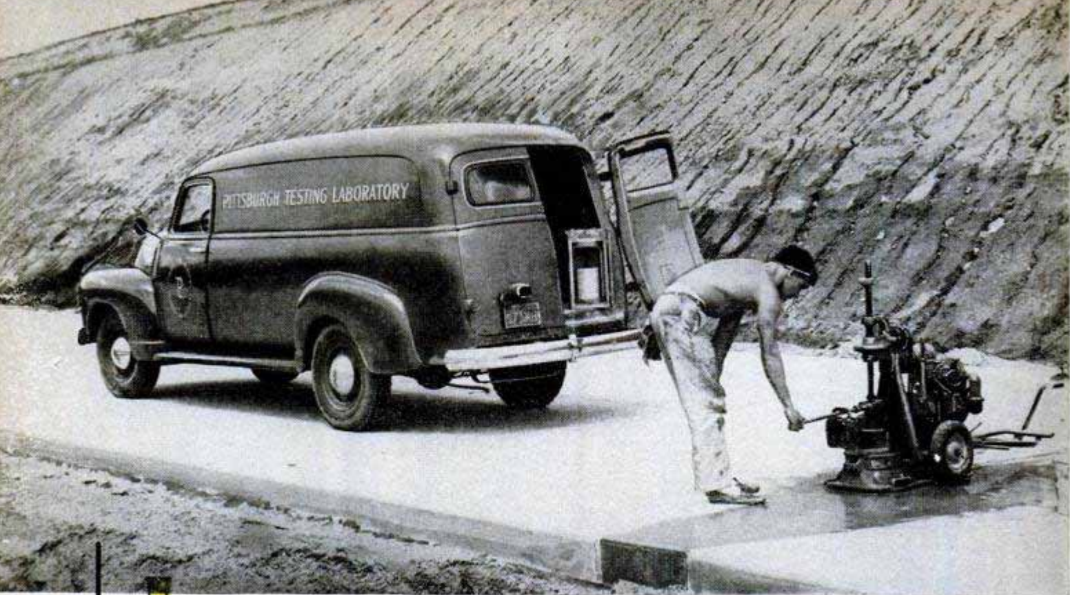
Core drill obtains sample of new pavement. Contractor is paid on basis of thickness and quality
