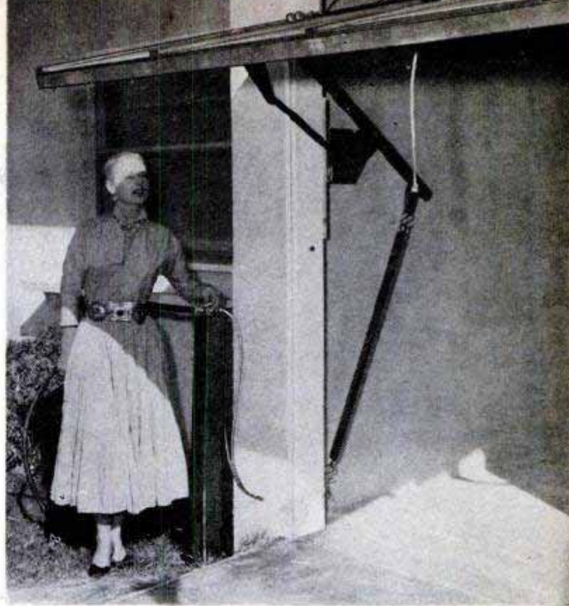
Valve on top of post beside entrance is turned to open or shut door. Another valve is situated in house
