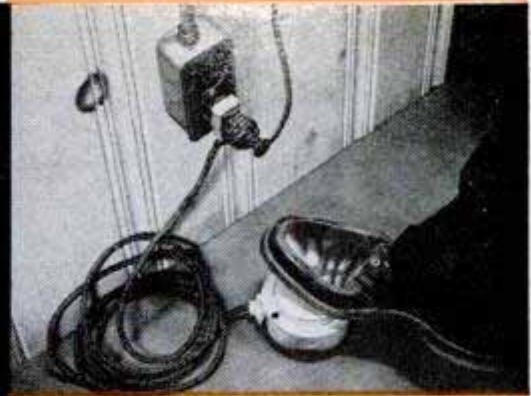
The appliance is plugged into the converted three-way plug which in turn is plugged into wall receptacle
