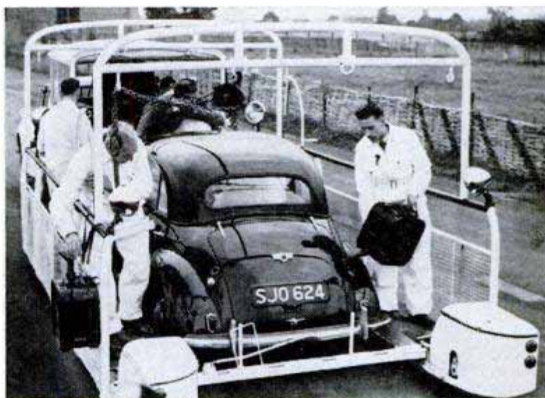
Refueling in motion. A positive thrust against the trailer of at least 10 pounds was maintained by the car during servicing
