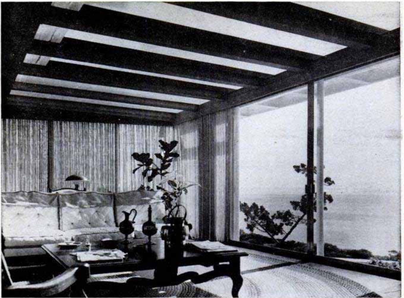
Retracted roof panels transform living room into a sunny, open-air patio. Single electric motor does the work
