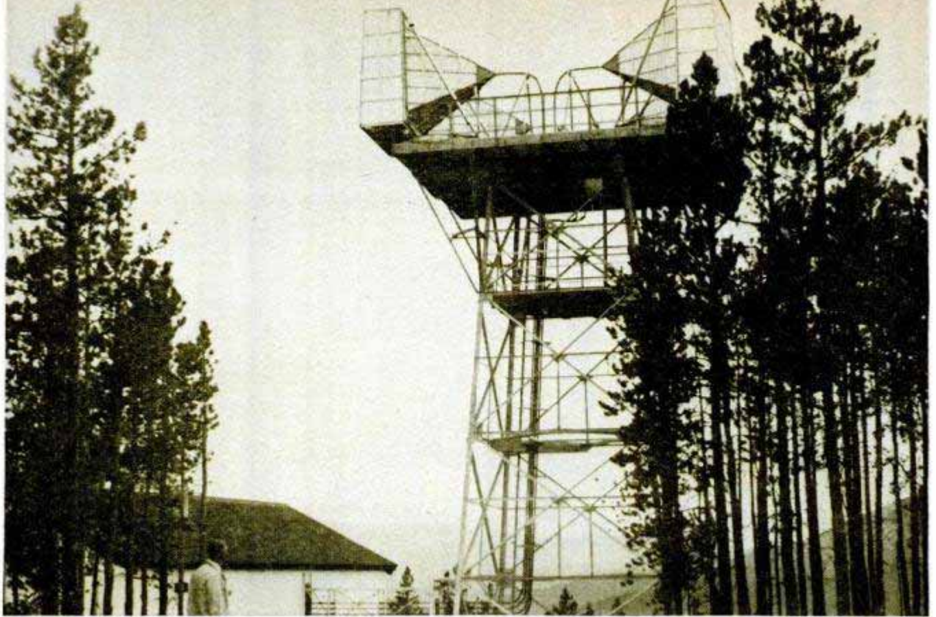
Huge electronic lenses of Buckhorn tower connect to microwave pipes that carry impulses to and from station
