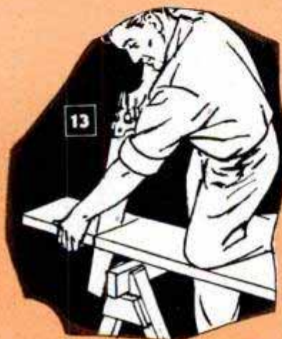
HOLDING WASTE END TO PREVENT SPLINTERING AT FINISH OF CUT
