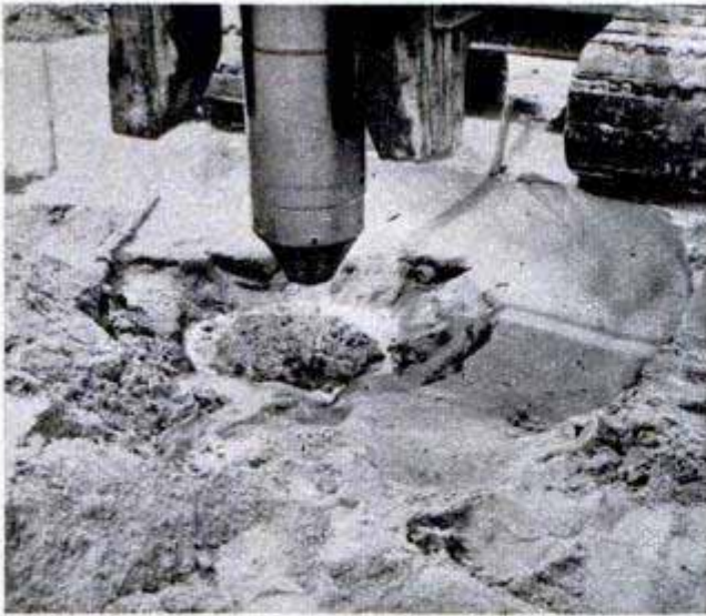
Water jet saturates sand beneath vibrating packer. Right, big tube on crane packs column 12 feet deep
