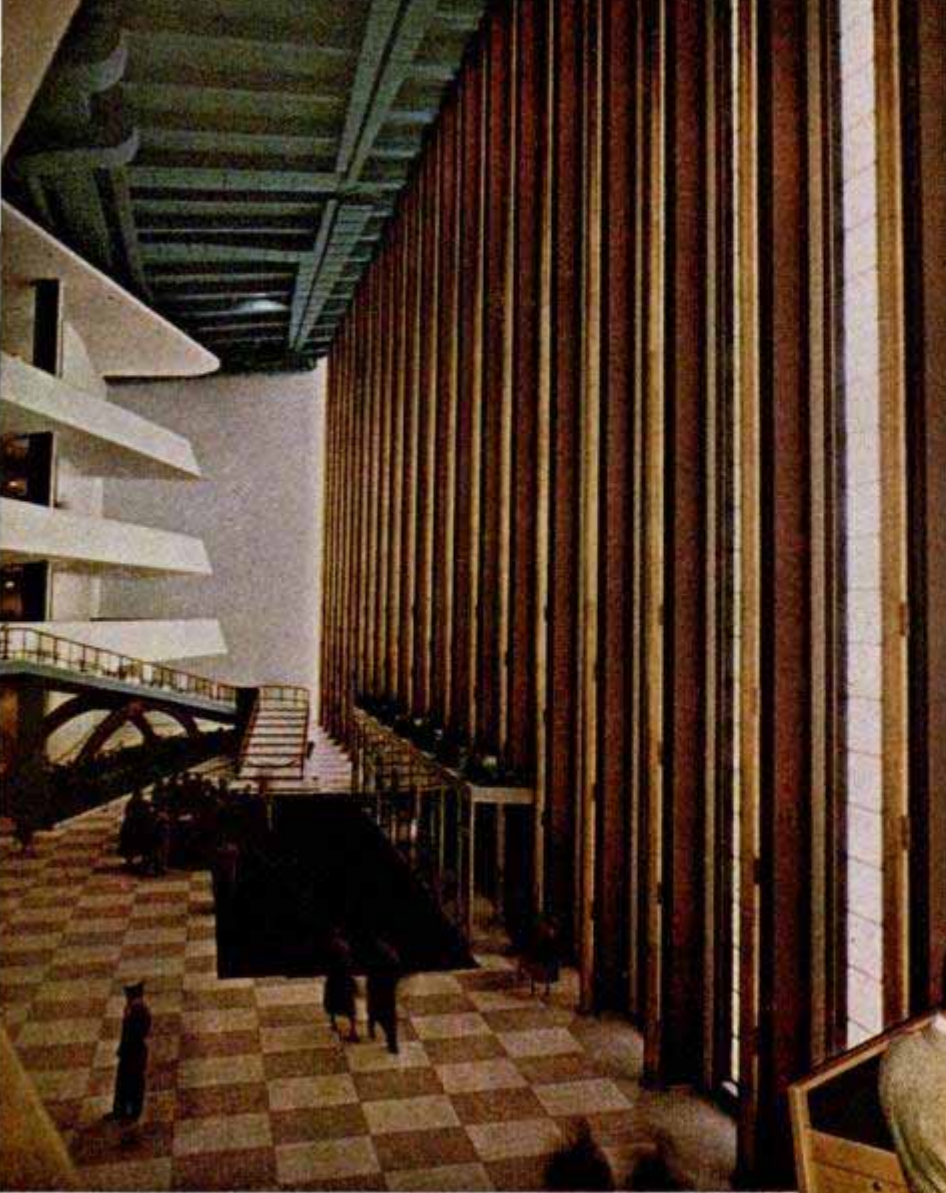
Cantilevered balconies jut out over lobby, which is 75 feet high. Beams and girders become part of decor
