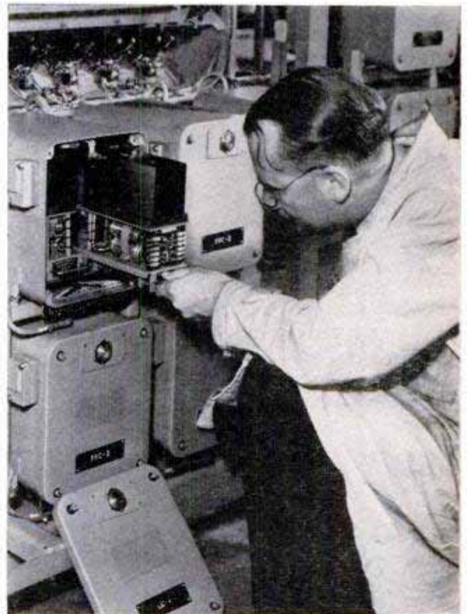
Technician watches windows, controls operations in plant with hand switches. Below, units slip out for repair
