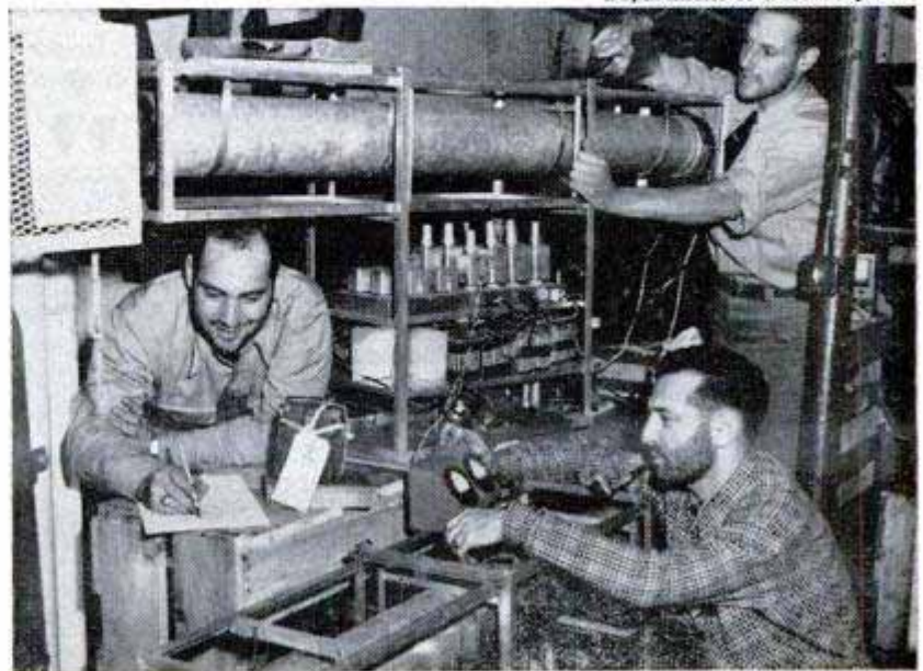
For altitudes up to 90,000 feet, big balloons carried long trains of antennas, radio gear, Geiger counters and other instruments. ↓ Bearded scientists make last-minute check of equipment for measuring cosmic rays before attaching it to a rocket or balloon train
