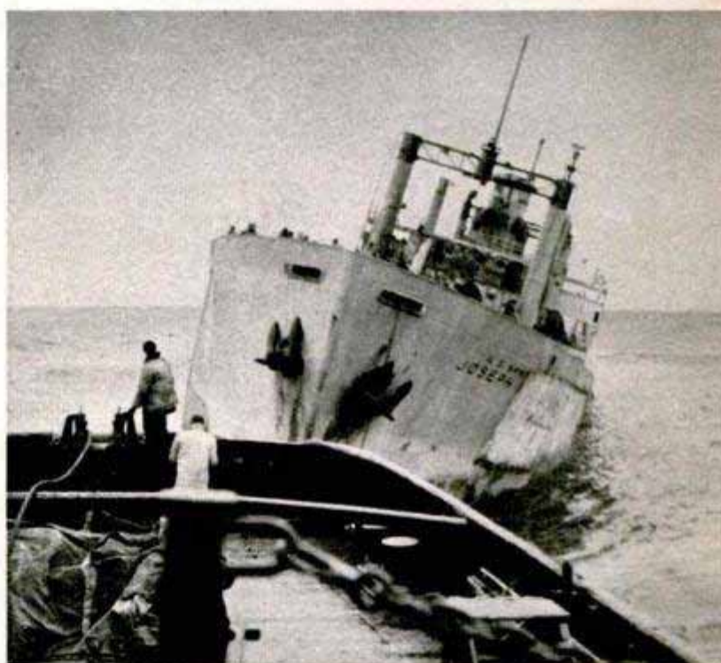
Big tow cable, fed over spools on Curb to prevent chafing, is made fast to a ship wallowing at sea
