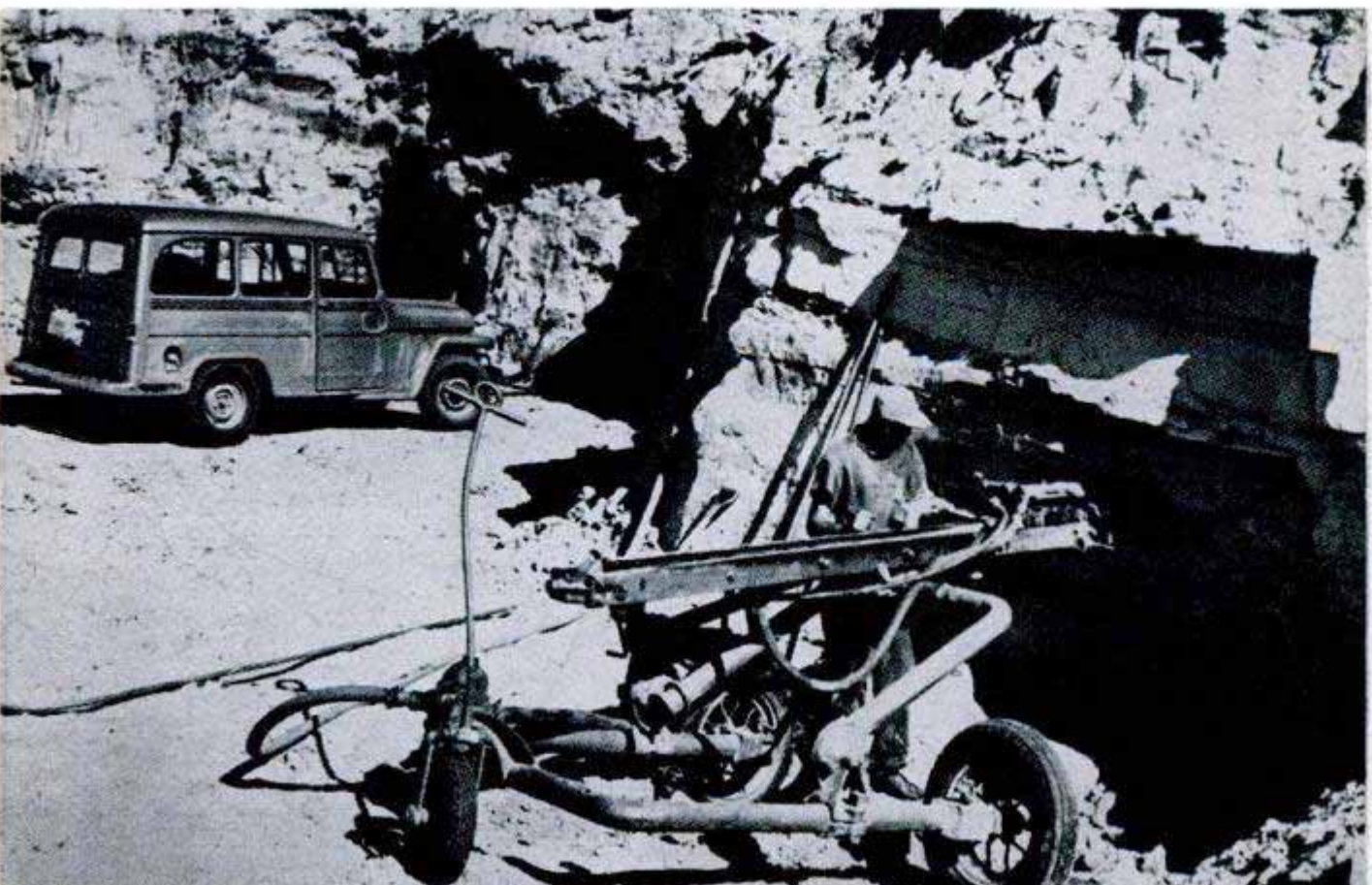
Uranium miners use air drill to make holes for dynamite charges in making tunnel to area of successful test
