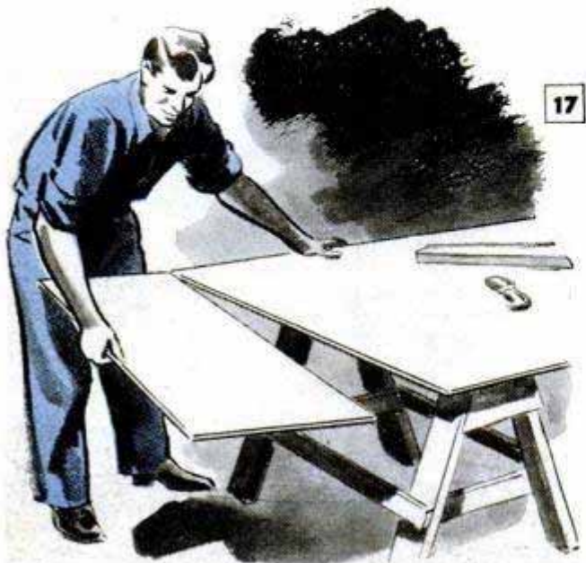
Next, cut cardboard layer on underside with knife which produces a clean uniform break as below
