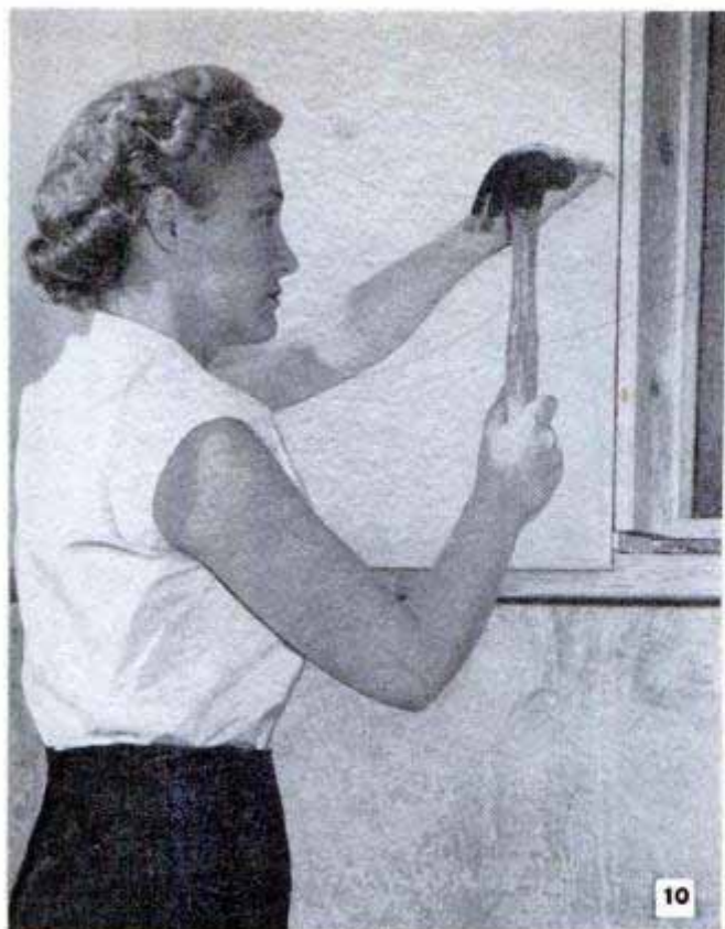
The family teamwork is going strong at this point. Olwen (Mrs. Ward) nails on fitted wallboard panel while Betty gets busy with crack filler to cover countersunk nailheads in the door and the window trim
