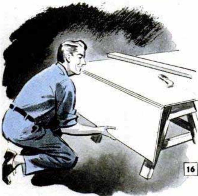
To cut Gypsum board, first cut top surface with knife, then press downward to break board as below
