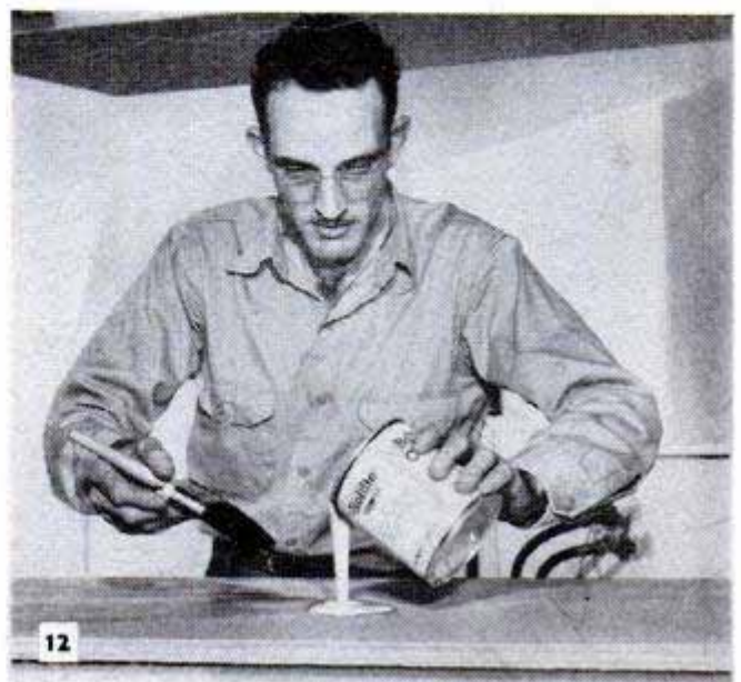
First step in applying decorative laminate to bar and counter tops is to spread adhesive and let it dry
