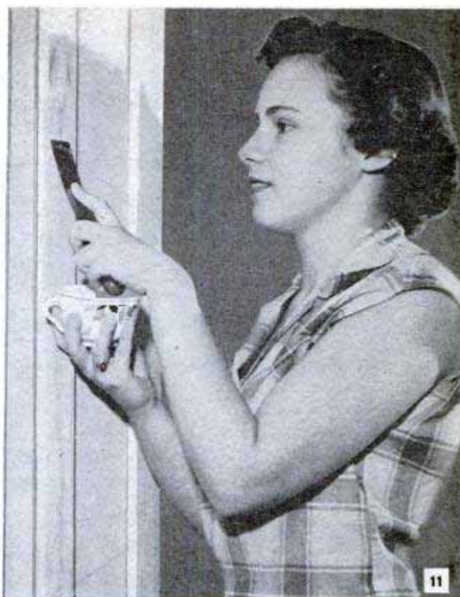
The family teamwork is going strong at this point. Olwen (Mrs. Ward) nails on fitted wallboard panel while Betty gets busy with crack filler to cover countersunk nailheads in the door and the window trim
