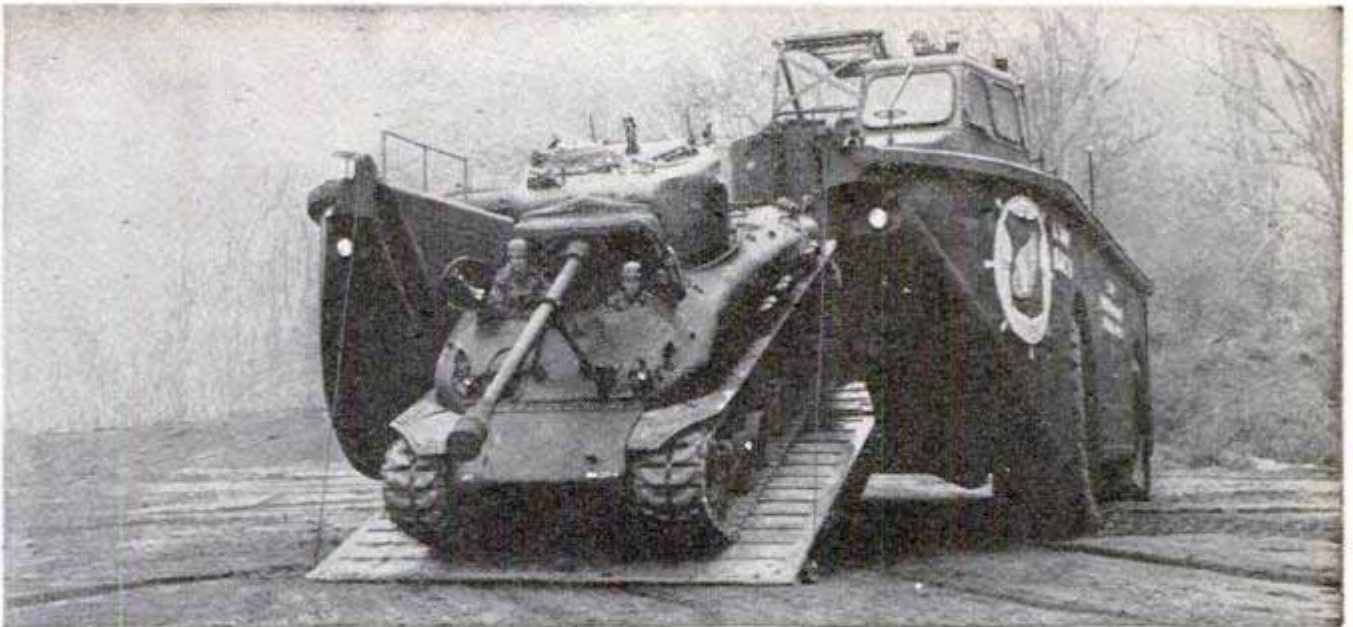
Sailing ashore, a "barc" can disgorge a 35-ton tank and a 35-ton crane in the same load. The Army's newest amphibious vehicle is 27½ feet wide, 61 feet long and 16 feet high. With fuel, it weighs 197,000 pounds
