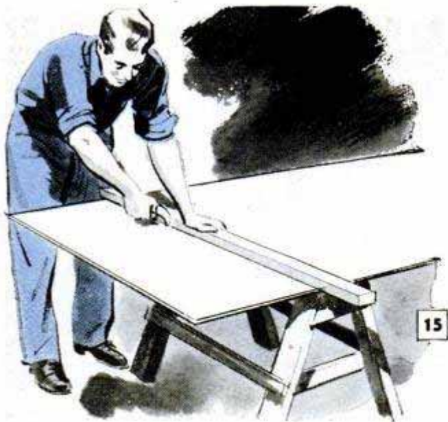
To cut Gypsum board, first cut top surface with knife, then press downward to break board as below
