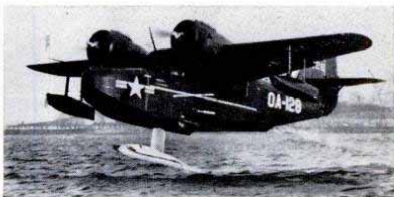
Above, JRF-5 hydro-ski test plane has single ski on a fixed strut below hull. This plane was tested for multibase operations and additional skis were added (below) for use on snow and ice. The ice tests were too rough on the airplane
