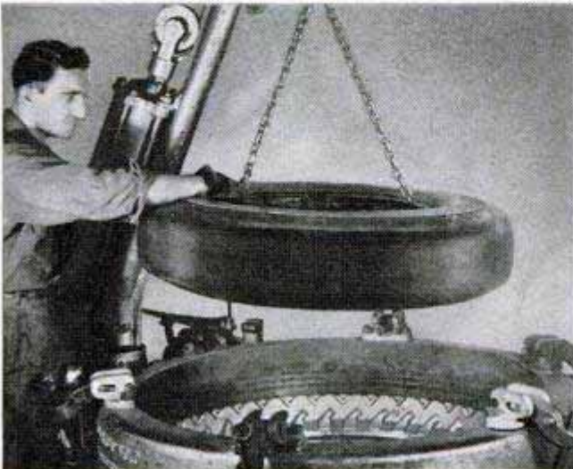
With a matrix to give the desired pattern to the tread, casing is carefully centered in the mold and clamped. Heat of the mold softens camelback rubber, while pressure is applied to force it into the matrix design
