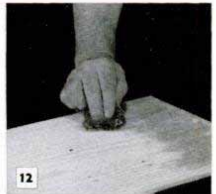
Left, remove softened paint with a dull putty knife. Right, use alcohol and rub with No. 2 steel wool in final cleanup operation
