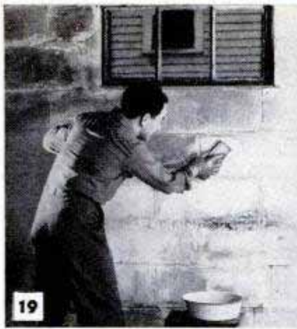
Left, applying 20-percent solution of muriatic acid to cut water-resin paint. Center, using 100-grit waterproof sandpaper to remove decals. Right, using electric peeler to remove paint on flat surfaces of door
