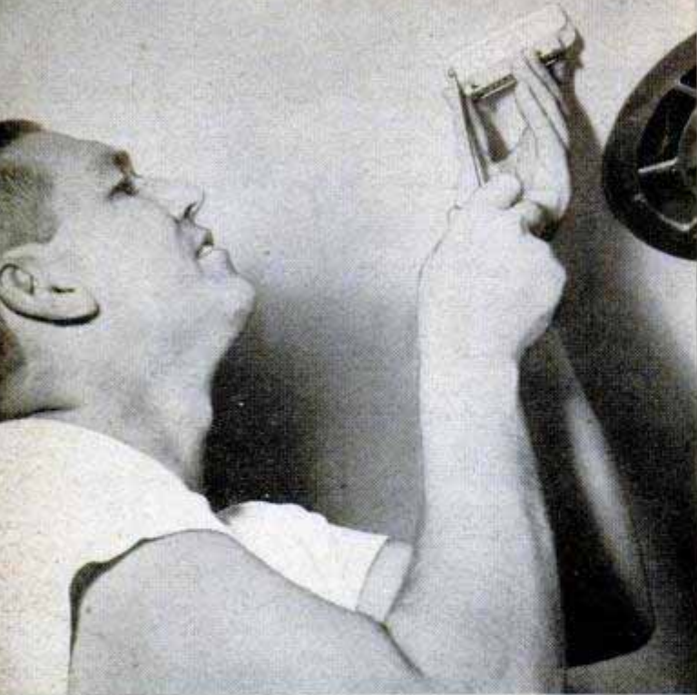
Heat detector on ceiling has bar of fusible metal that melts at 160 degrees and sets off fire alarm
