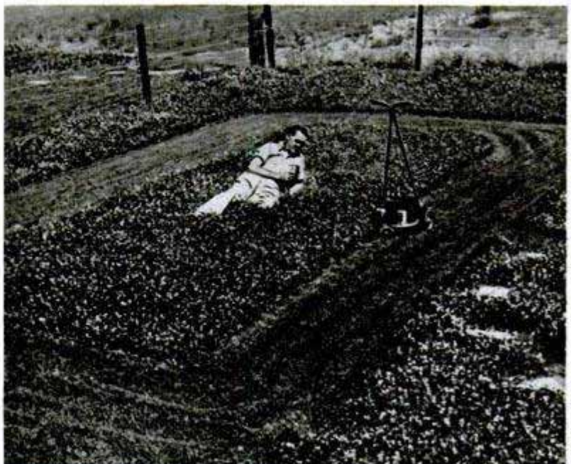
Designer Meyer makes adjustments (left) and then relaxes as automatic attachment guides mower around lawn
