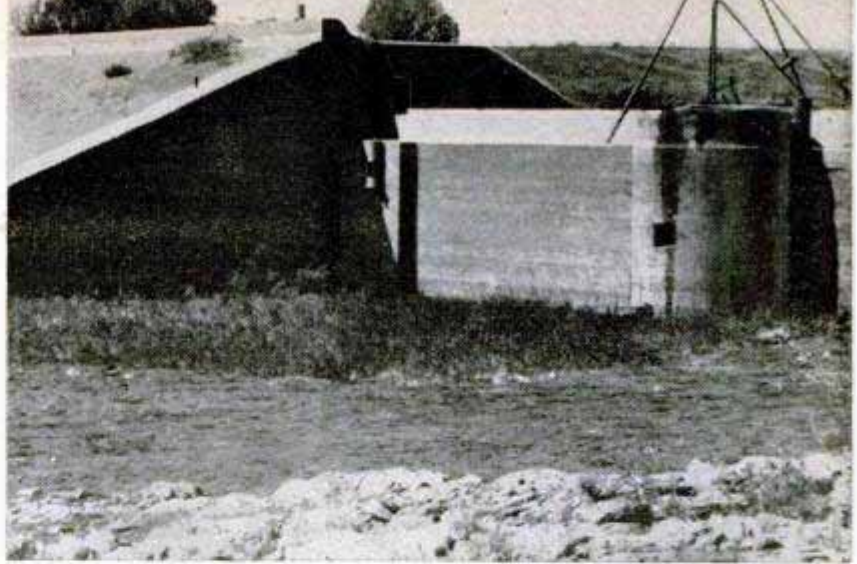
Broken Hill's main water reservoir at Stephens Creek looked as dry as the desert that surrounds it. Normally, 20 feet of water cover the sandy bed. Small hole in wall is the water-outlet valve
