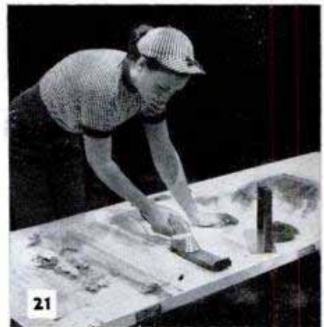
Left, applying 20-percent solution of muriatic acid to cut water-resin paint. Center, using 100-grit waterproof sandpaper to remove decals. Right, using electric peeler to remove paint on flat surfaces of door
