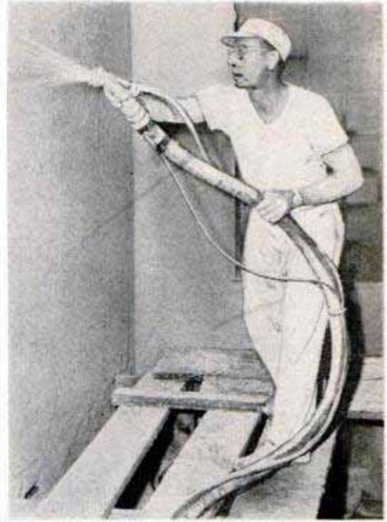
Left, workman prepares machine for a mix. Right, a stream of compressed air forces plaster against the wall
