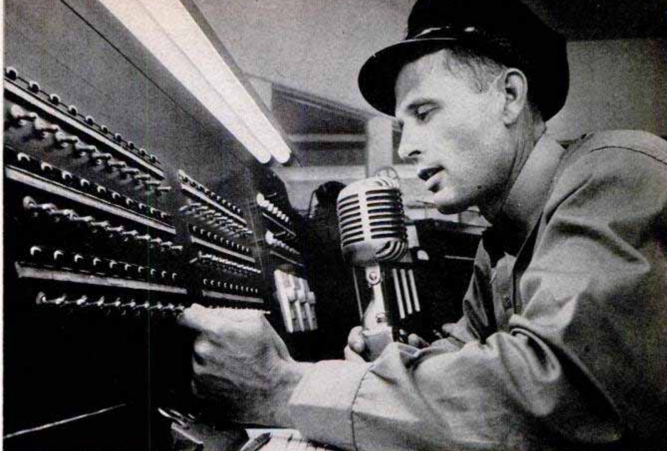
Control operator receives fire reports, alerts men, opens doors and switches traffic lights to clear route
