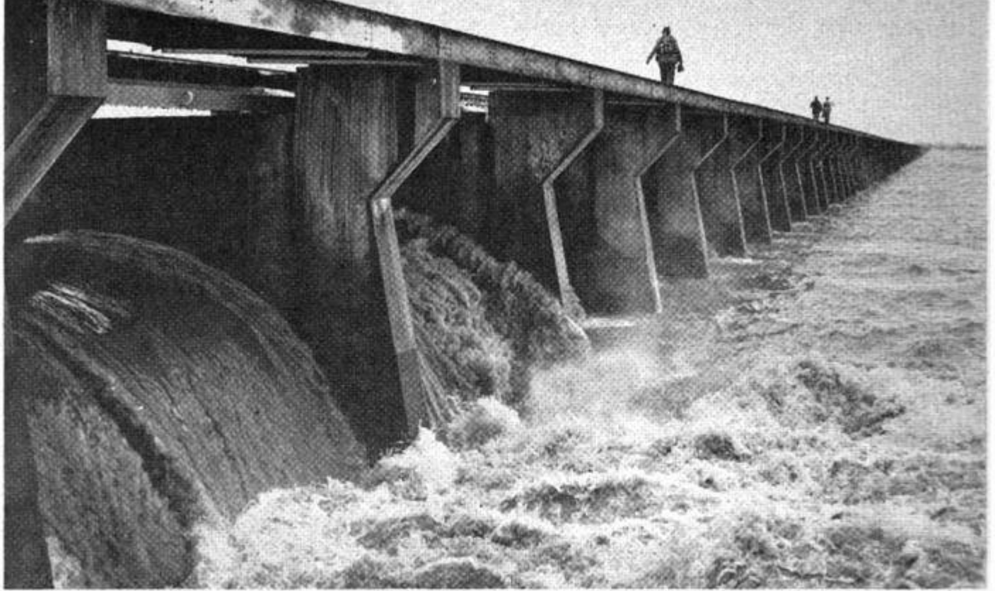
Water from the Mississippi races through Bonnet Carre as that "safety valve" is opened to release pressure
