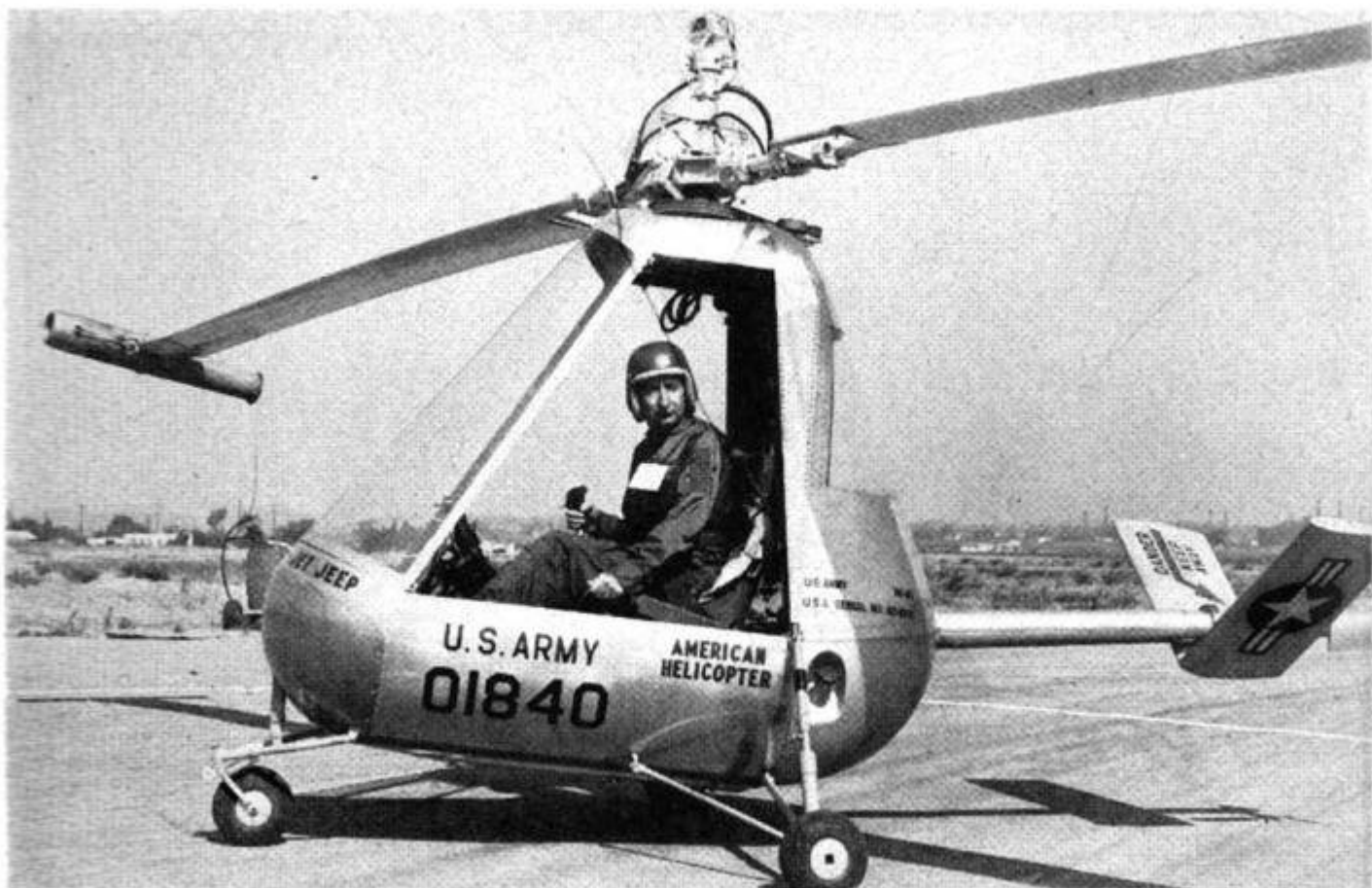
Pulse-jet engines at the rotor tips give the Army's new one-man helicopter an 80-mile-per-hour top speed
