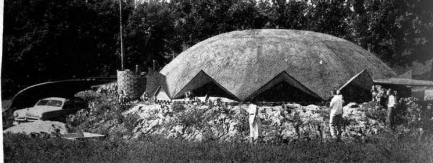
The earth itself forms outer wall of this round house with concrete dome; round chimney is for fireplace
