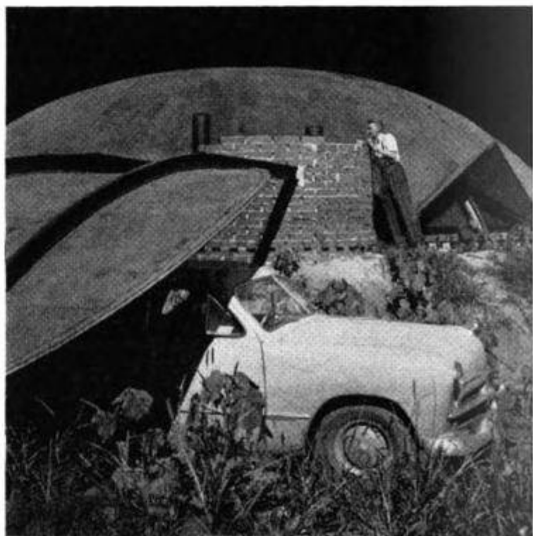
Slanting circular carport roof is made of plywood molded on the job. The floor plan below covers 1800 square feet. Beneath center skylight are hanging bowls of planted greenery to form woodland ceiling
