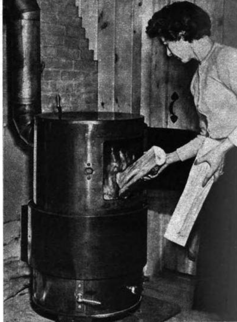
Commercial heater needs stoking only once or twice a day, burns wood slowly and completely and is governed by automatic controls. It roasts wood to charcoal and burns combustion gases before they escape
