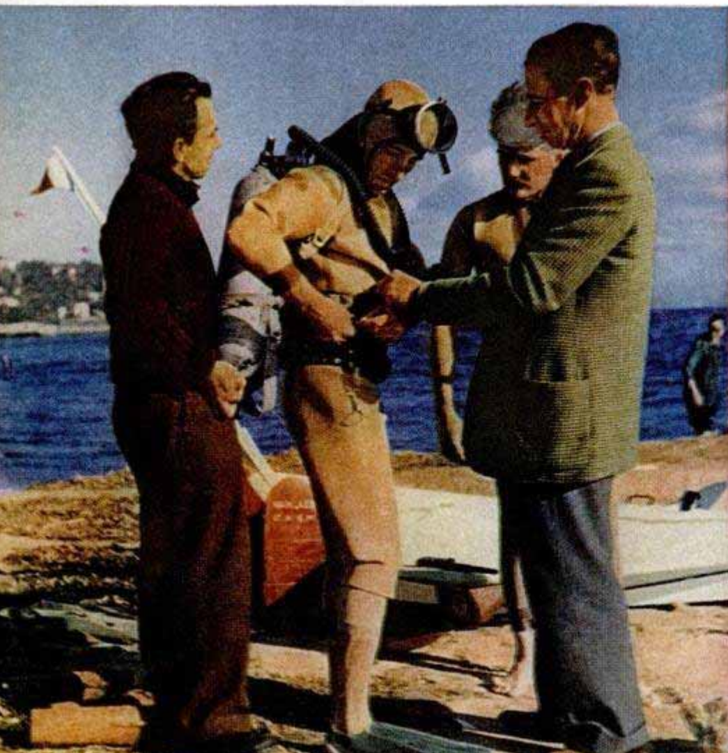
Compressed-air bottle is strapped to pilot's back. Each bottle provides 30 minutes' air supply and the pilot can wear three of them if he wishes
