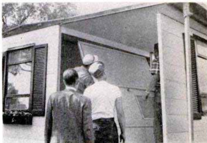
Panel wall with its doorway is tipped sideways and slipped into place. This is secret of home's mobility. Below, propped-up ceiling will become side of package
