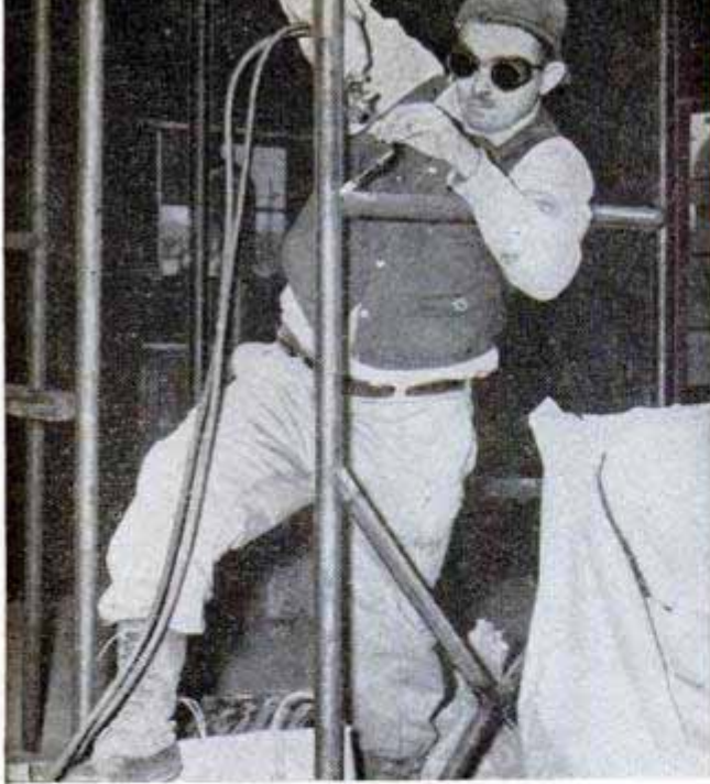
John F. Wagner of Johnstown, Pa., designer and builder of "pipe dream" house, uses steel pipes as both structural members and part of heating system
