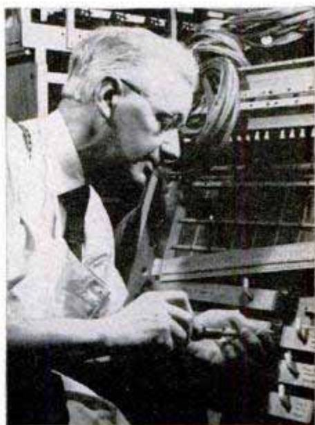
Air is introduced into each pipe by means of an electrically controlled valve operated by the keyboard. The organ expert above is working on one part of the control-valve mechanism
