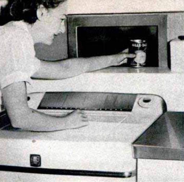
Trash goes through a hinged partition in kitchen wall, falls into a storage bin outside the house
