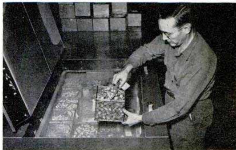
Aluminum rivets, made malleable by keeping them cold, are delivered to workmen from freeze chests. Below, 40-foot aluminum lifeboat carries 140 persons
