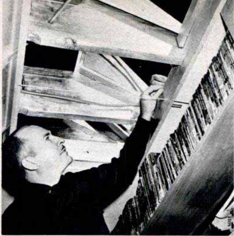
Skylight panels have mirrors which reflect sunlight into house. Behind panels are tubes for night lighting
