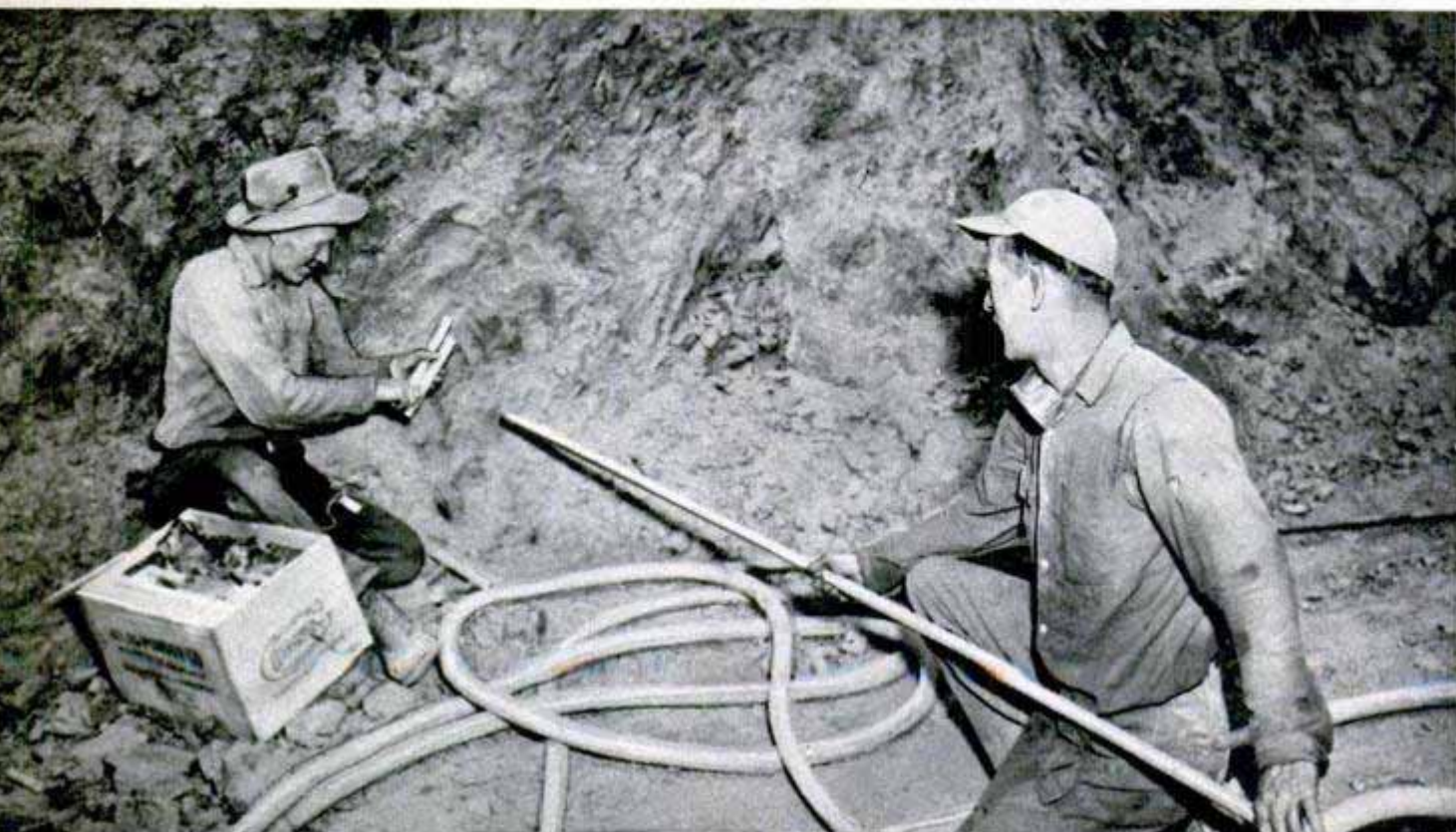
New roads to the cobalt mine had to be blasted through the mountains; one road took a carload of dynamite
