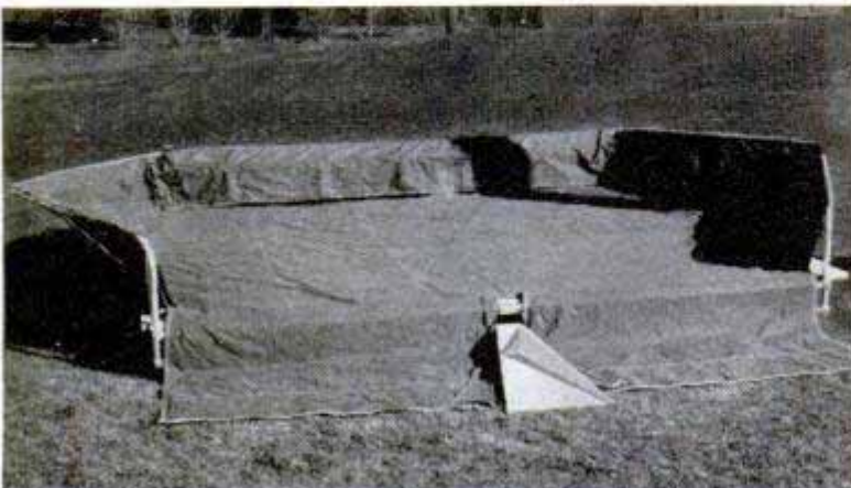
After the pit bottom is laid with loose wooden planks to give it a springboard effect, it is covered with a canvas tarpaulin
