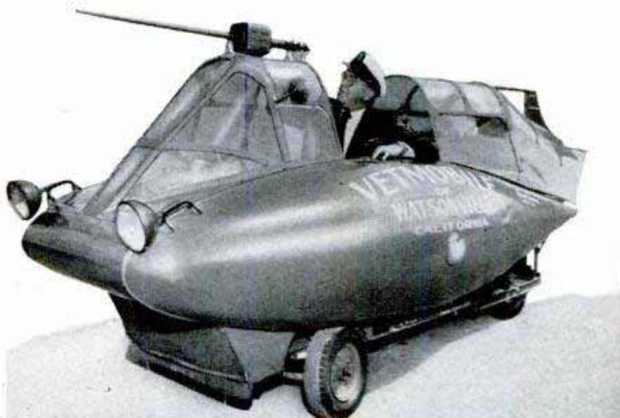
It may look like a machine gun, but it isn't. It's the antenna for the two-way radio. Seated in the cab is Ed Adkins, builder of the "Vetmobile"
